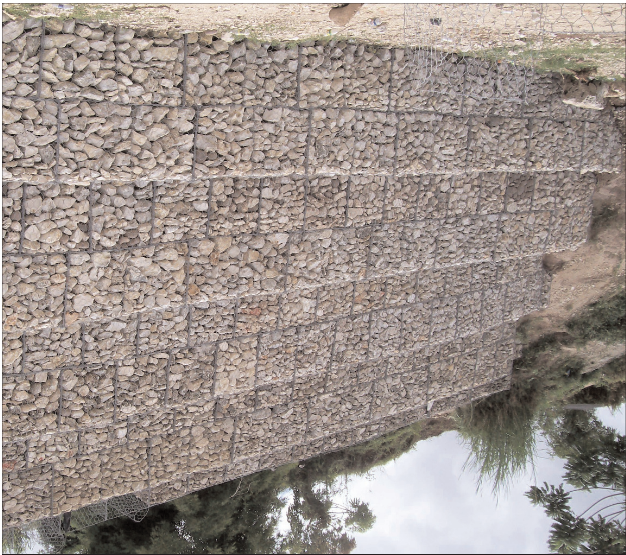
Figure 6: Gabion Wall under construction in Pitsgah, St. Elizabeth.
