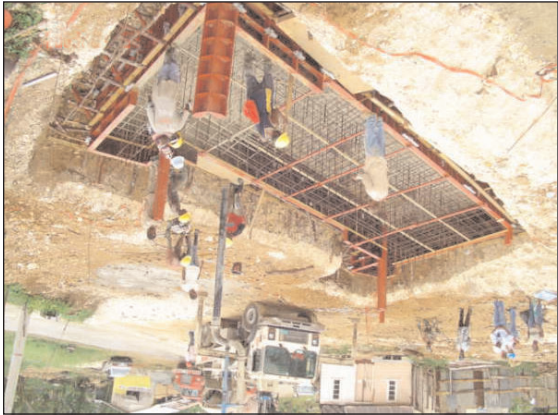
Figure 22:Concrete being poured for one of the Abutments of the Seven Rivers Bridge, St. James
