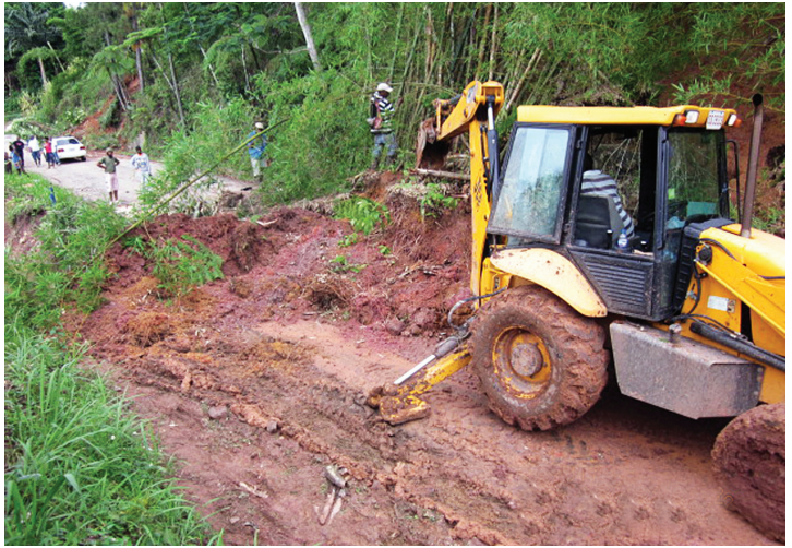
Work underway on the Mears Bridge to Grennock's Bridge corridor to clear one of several landslides at James Hill
