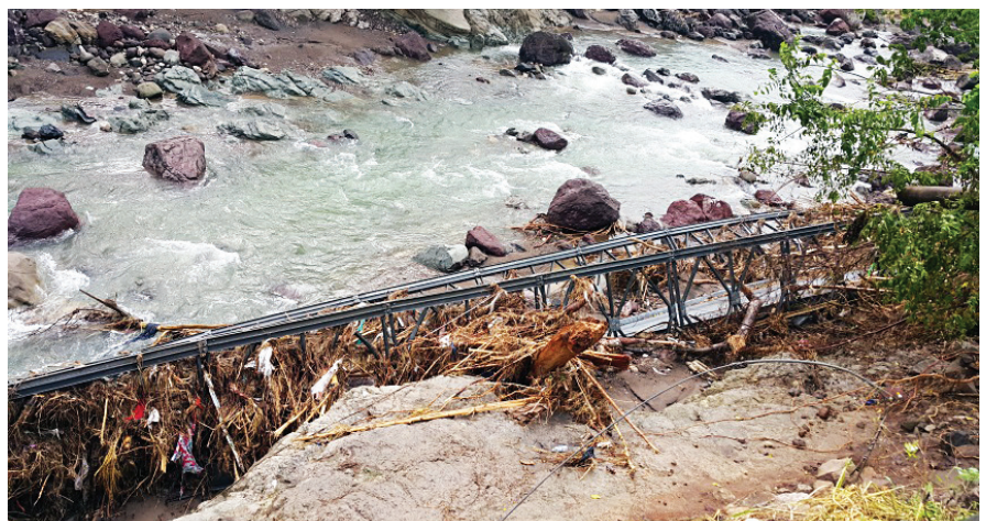
The four-year old Bailey bridge at Southwood was deposited at Dam Head 2km downstream by 40 feet high flood waters
