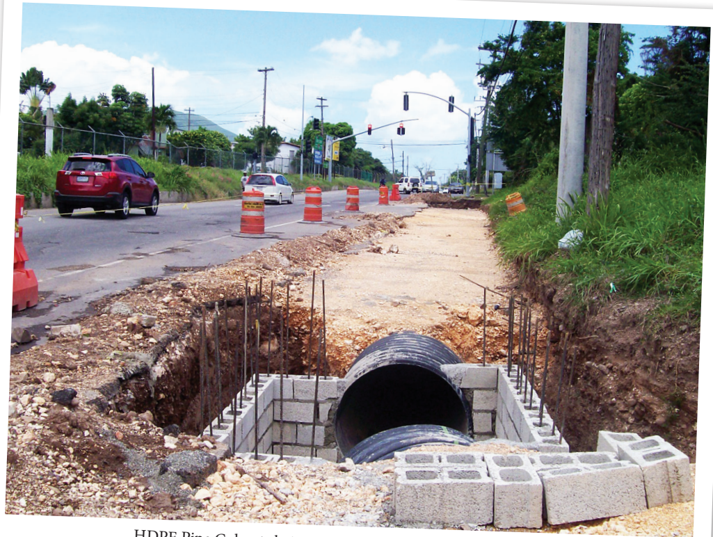
HDPE Pipe Culverts being installed along Mona Road as part of drainage solution
