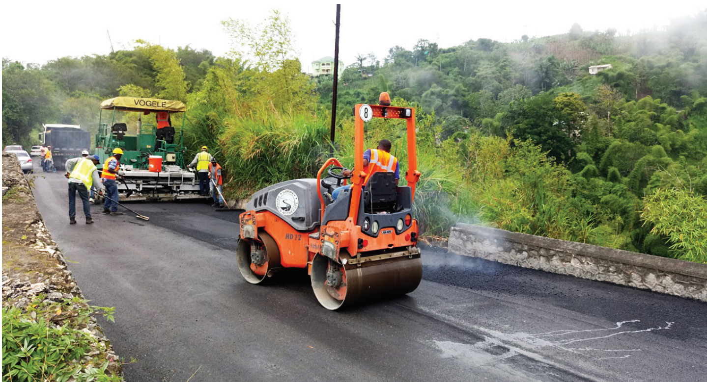
A crew from Surrey Paving and Aggregates Limited paving a section of the Highgate Hall roadway in Southern Trelawny. The roadway is being rehabilitated under the Wire Fence to Warsop road improvement contract.
