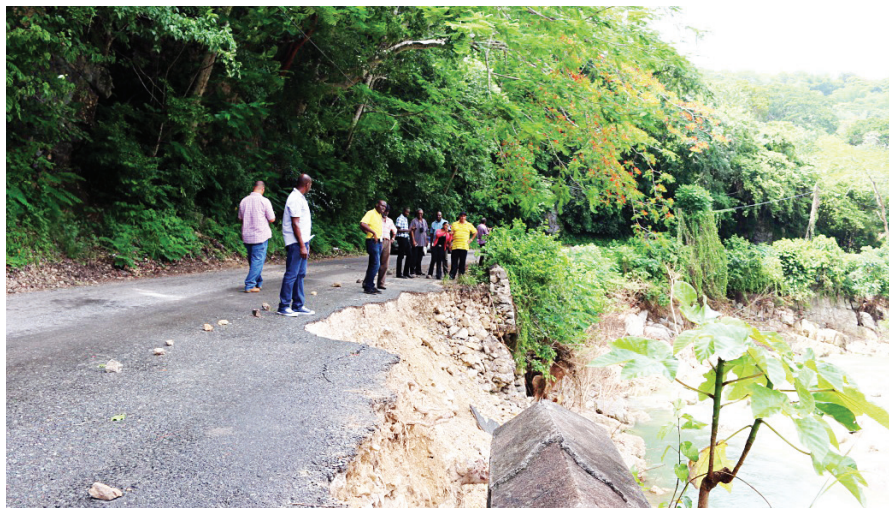
A breakaway at Kilsyth reduced the roadway to single lane traffic and imperilling motorists
