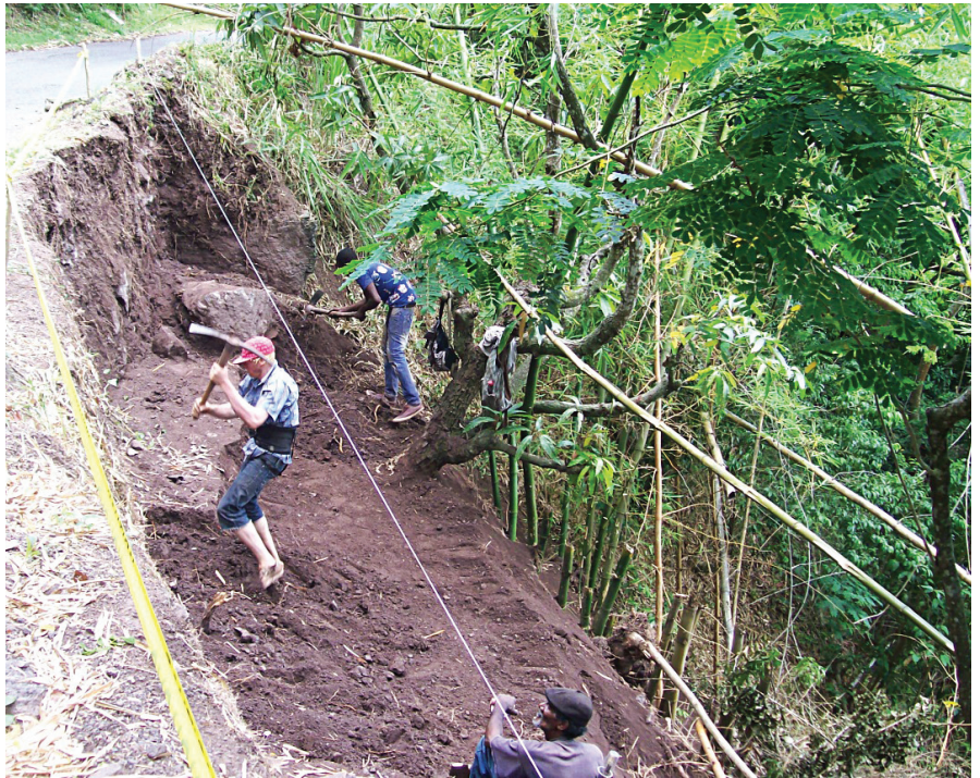
Excavation for the foundation of a Rubble Random retaining wall on Irish Town Road
