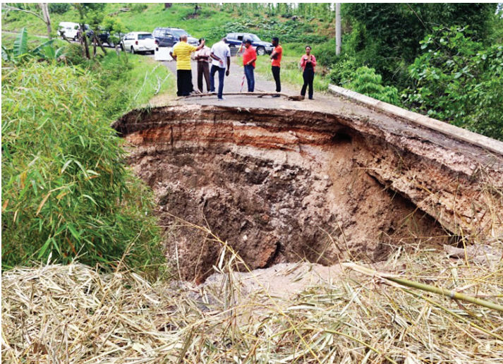
Collapsed box culvert at Dykes Hill will have to be rebuilt
