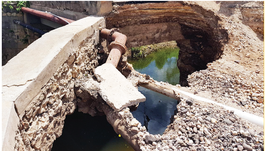
The Jacob's Hut bridge in Central Clarendon was overwhelmed by the sheer volume of water in its channel and caved in during April's heavy rains
