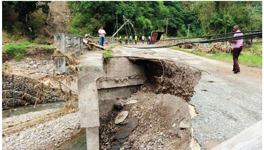
Both the Green River Bridge approach roads were washed out during the May flood rains.
