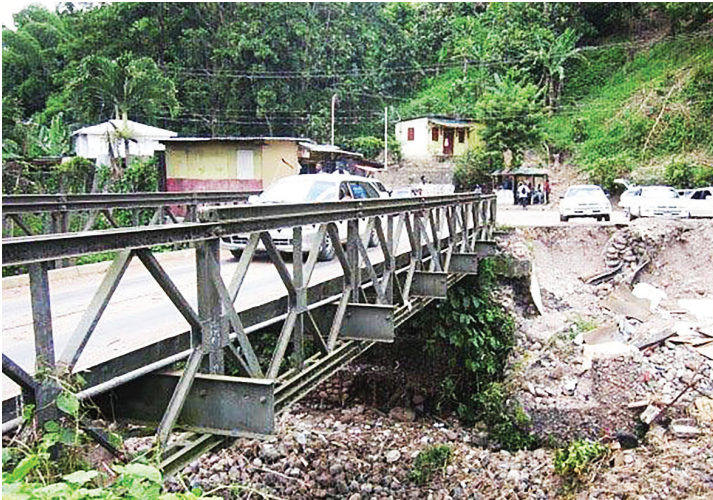
Rotted gabion baskets and eroded embankment at Pumpkin Bridge
