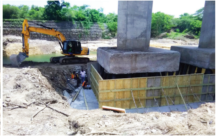
Pile protection using mass concrete to securely anchor the piers of the Rio Minho Bridge
