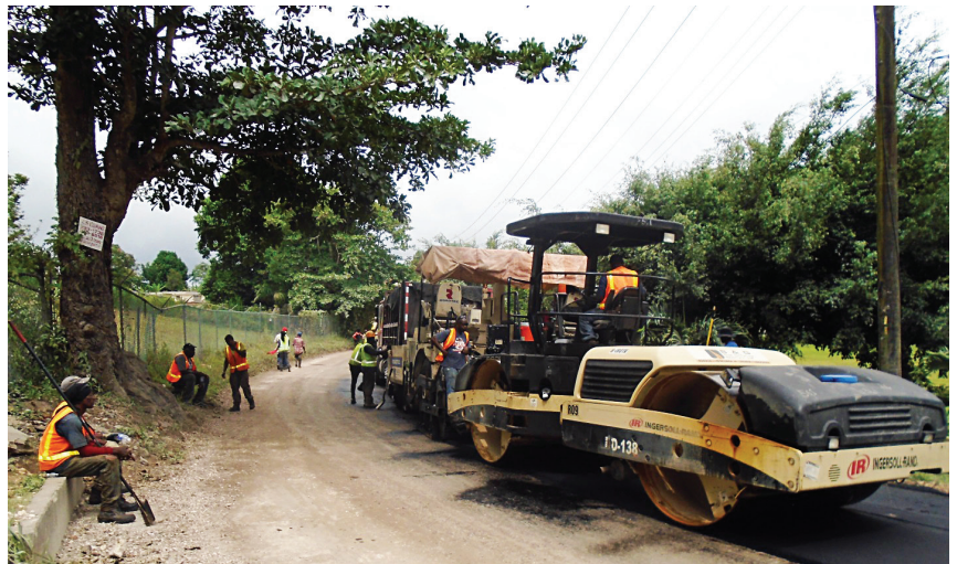
Overlaying works in progress
