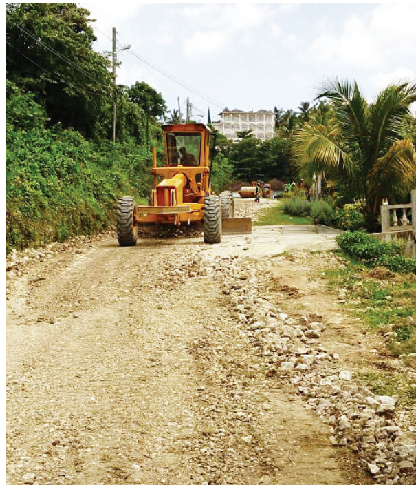
Base formation works along a section of Rhynie Drive in St. James.
