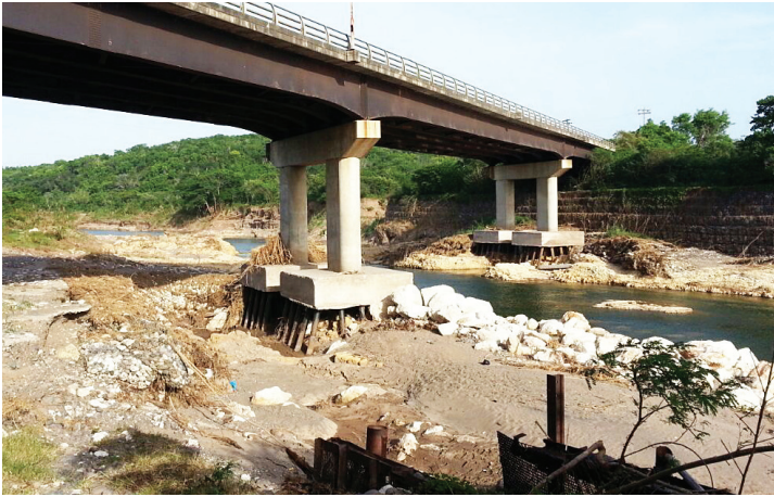
View of the piles which became exposed due to severe scouring during the May 13-18 heavy flood rains
