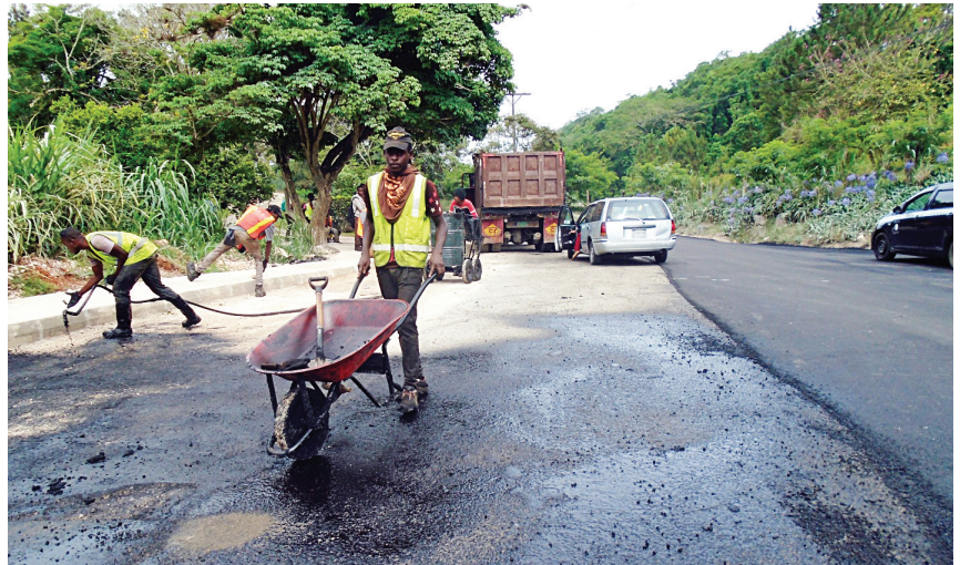
Tack coat being applied during overlay works
