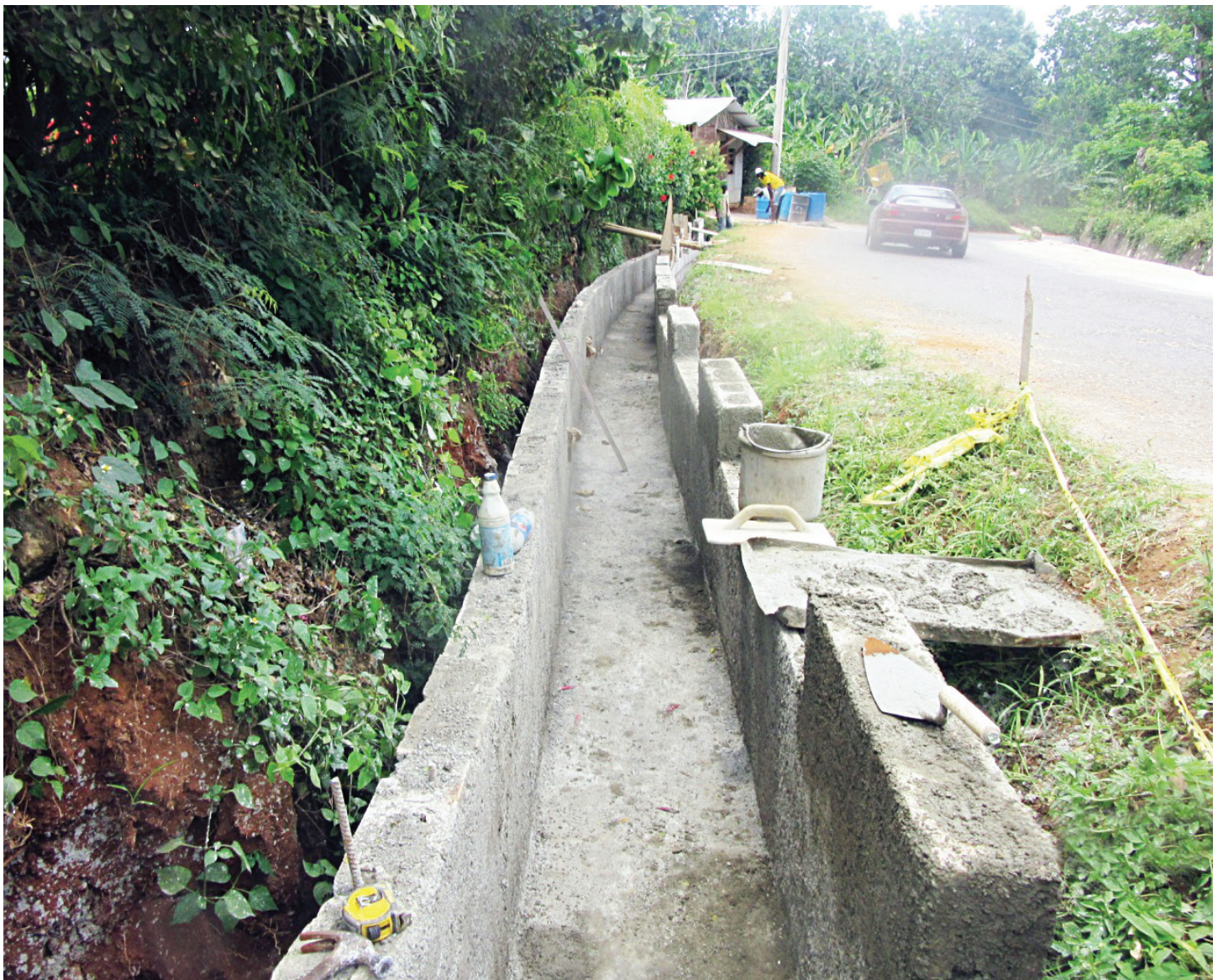
U-drain being constructed with outlets for storm water run off
