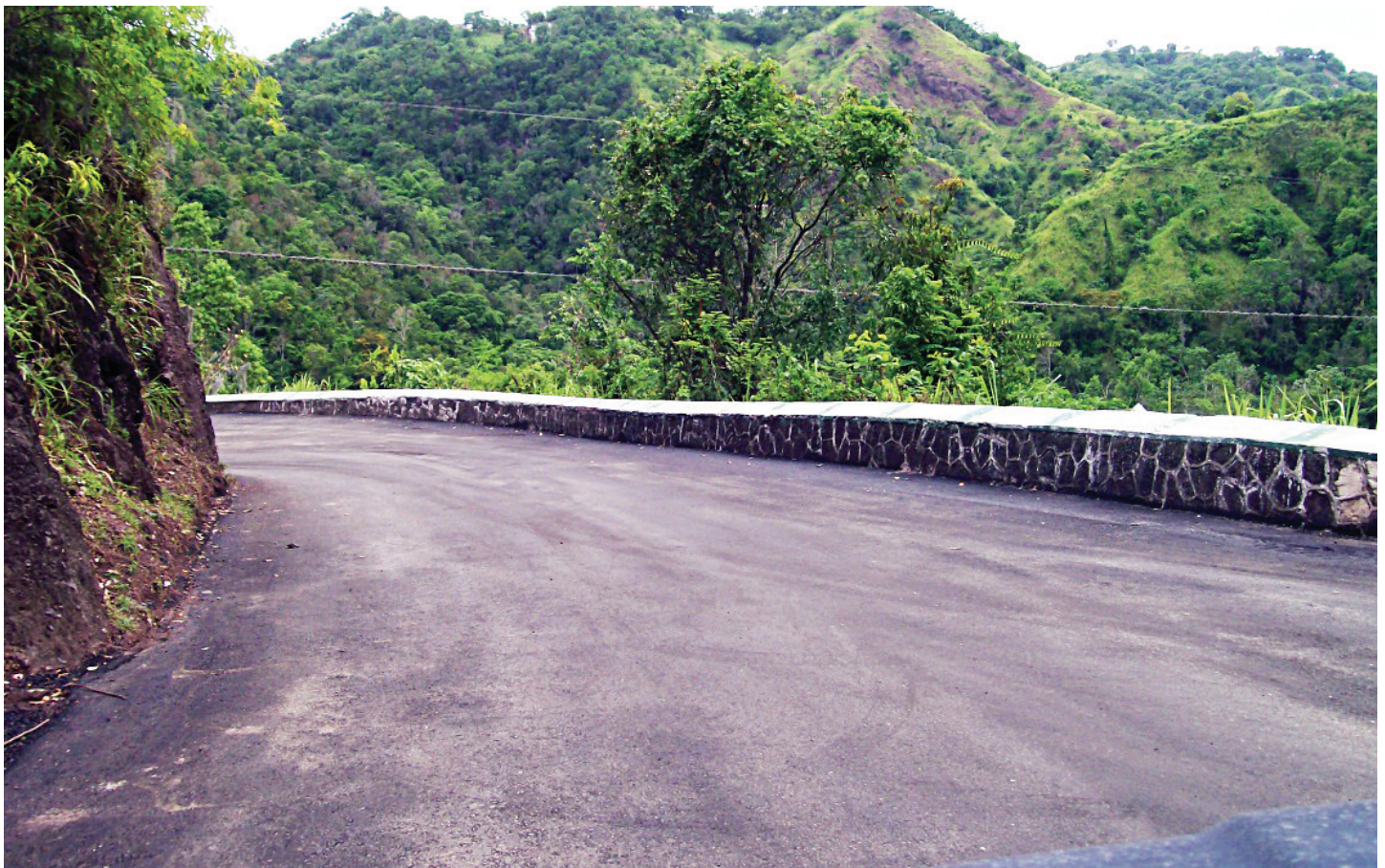
A section of the Papine to Redlight roadway that has been paved with Asphaltic Concrete
