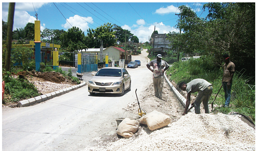
Kerb blocks being laid as an added drainage feature along the road
