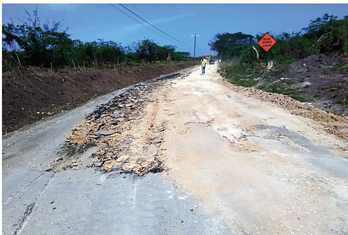
Scarified road surface in preparation for road formation
