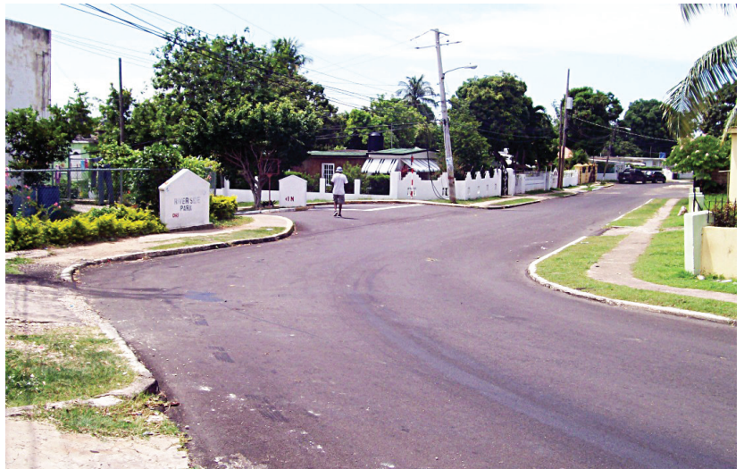
Denido Boulevard, main entrance to Riverside Park, part of 22707 M 2 , which has been overlaid with asphaltic concrete
