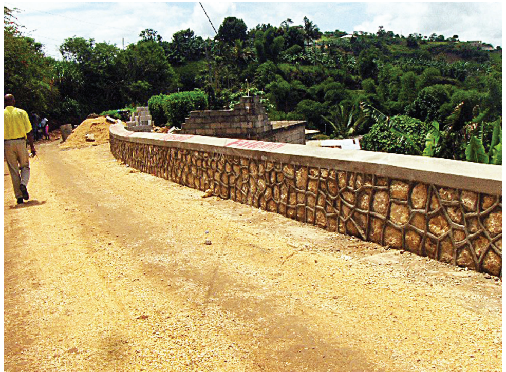
The Parapet of the retaining wall along with base material
