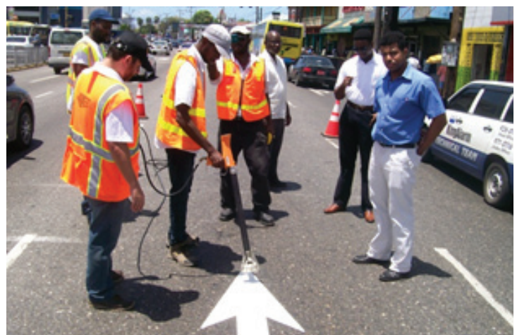
Directional arrow being installed along Constant Spring Road
