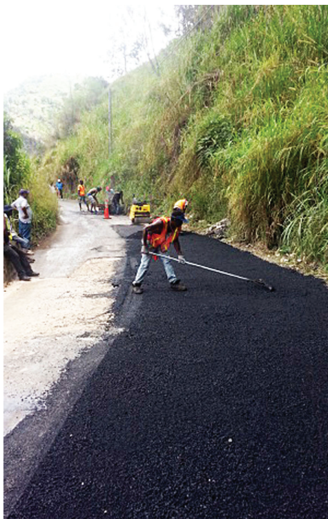
Workmen applying Hotmix to the Cooperage to Guava Ridge roadway
