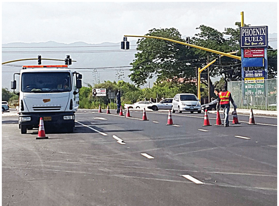
NWA road marking crew putting in lane markings prior to the traffic signals being commissioned into service.
