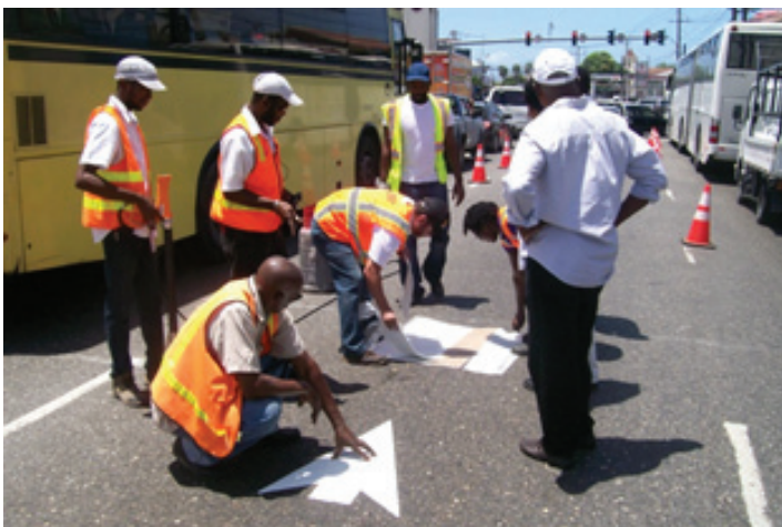
Directional arrow being installed along Constant Spring Road
