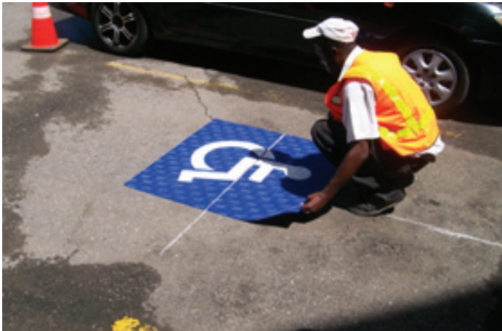
Technical officer, Michael Long, preparing the Thermoplastic sign for the application of the heat.
