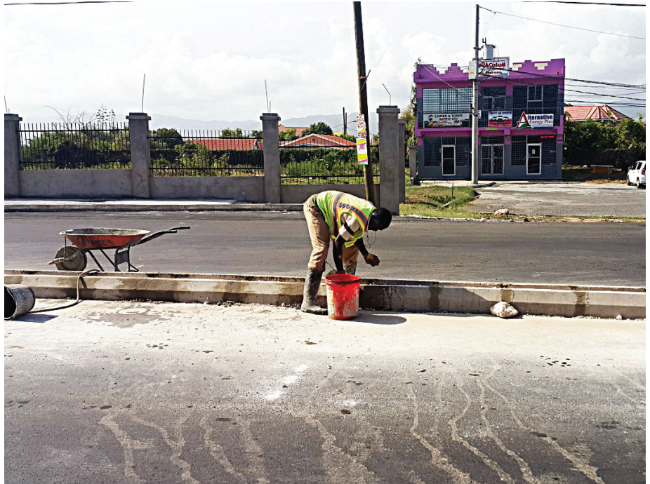
A mason putting final touches to a median along Passagefort Drive. The median will help to restrict conflicting movements in the vicinity of the intersection.
