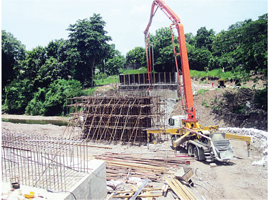
Construction of Pier at the new Kupius Bridge
