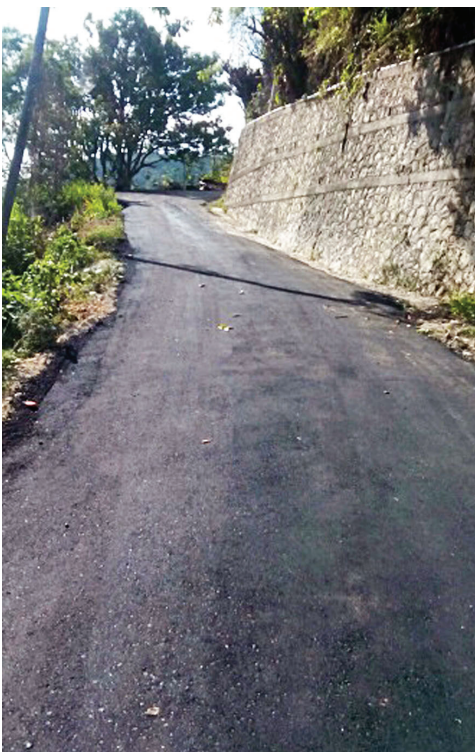
Sheet patching along a section of the Lindo's Gap to Constitution Hill roadway
