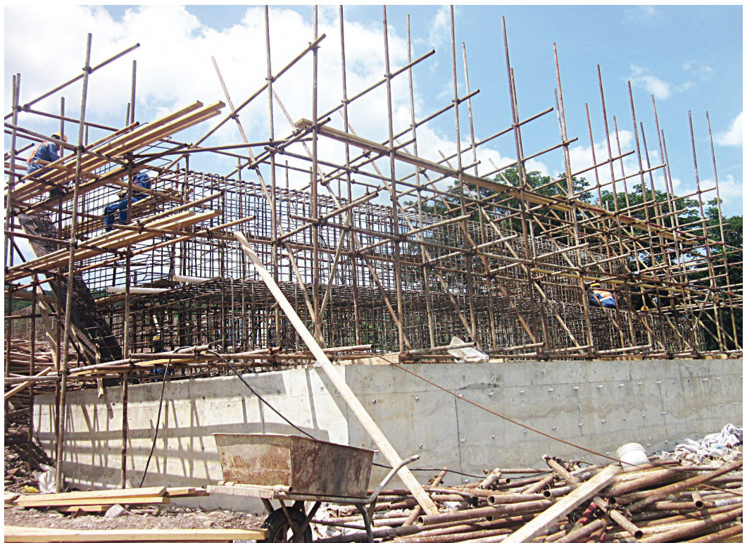
Construction of Abutment at the new Kupius Bridge
