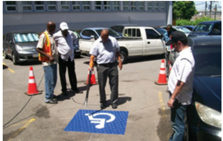
Director of Planning and Research, Patrick Rose (right) using the heat machine, which is used to bond the Thermoplastic to the Asphalt
