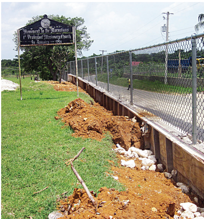
Section of the metal fence on a the concrete foundation
