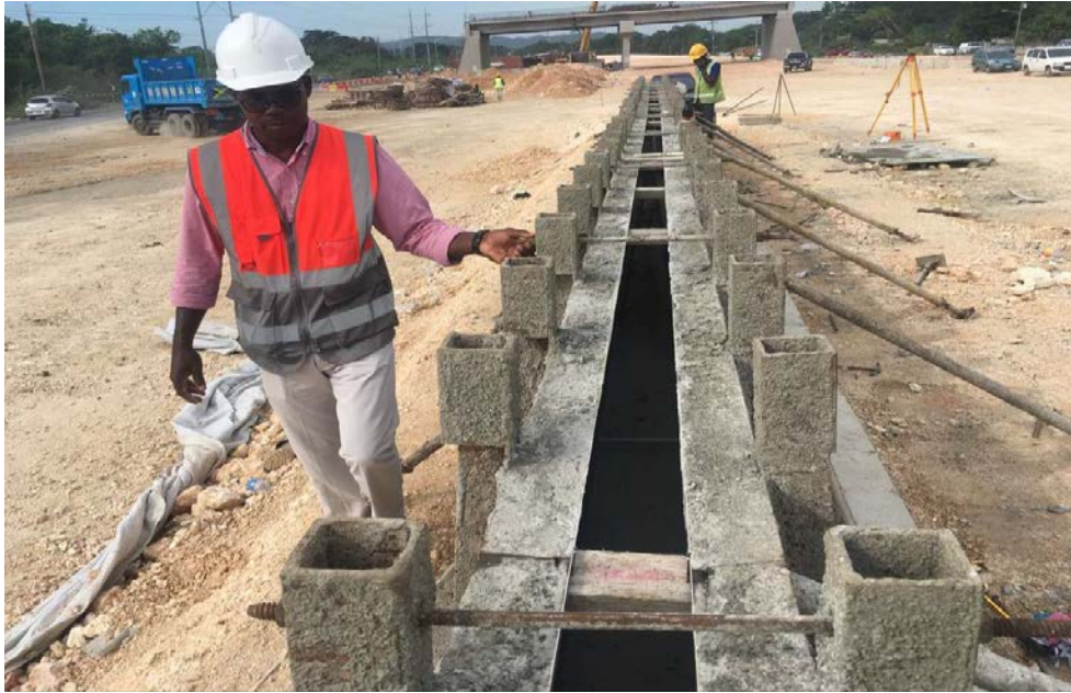
New Jersey Barrier formwork
