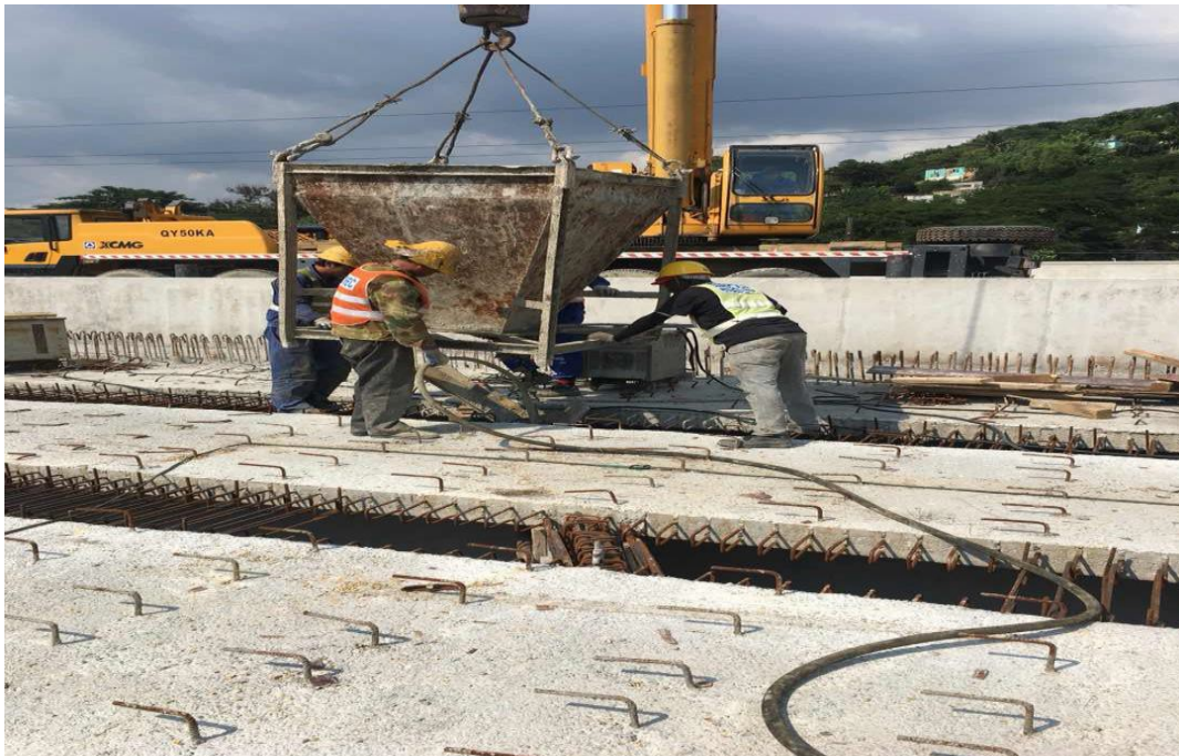
Pouring concrete to wet joint – Fresh River Bridge
