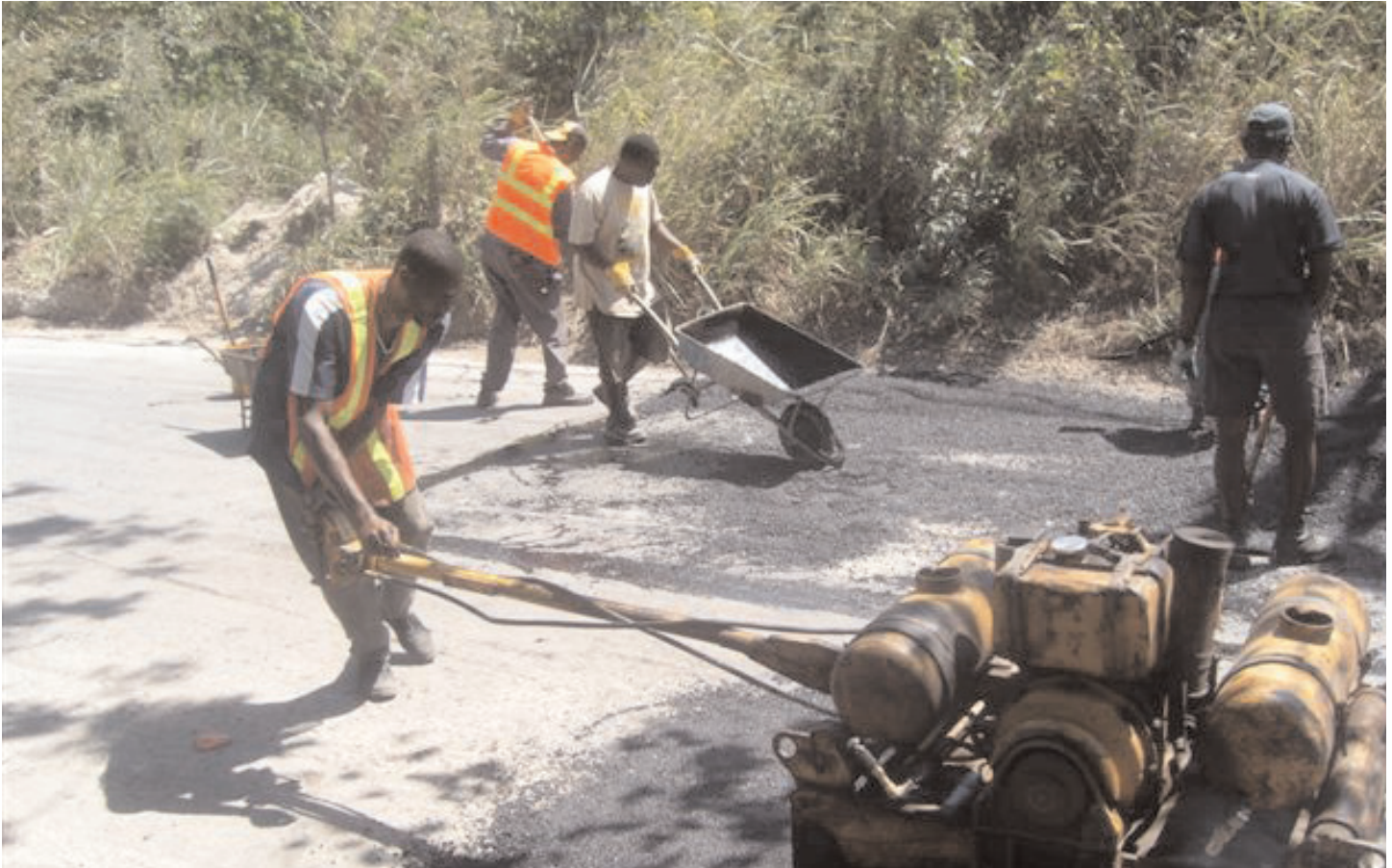
Workmen patching a section of the Fairfield main road in St. James
