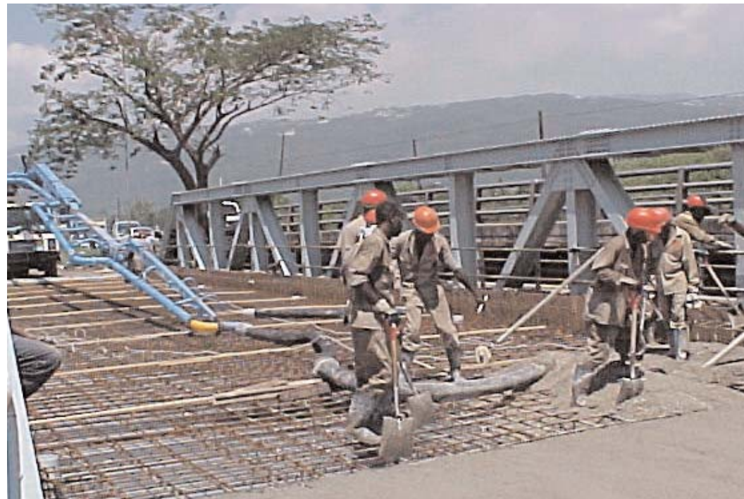
Workmen spreading concrete on the deck of the Sandy Gully Bridge, Spanish Town Road, Kingston.
