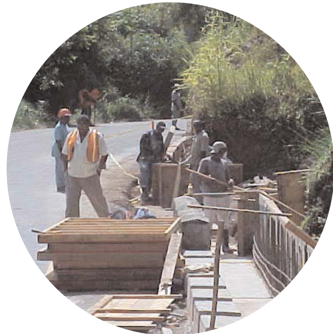
Workmen constructing a retaining wall along the Stony Hill to Toms River road, St. Andrew
