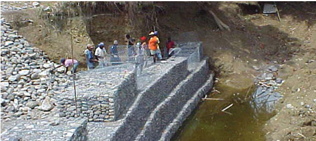
Gabion Basket works in progress at Haughten River, Orokage Hall Bridge, St. Mary.
