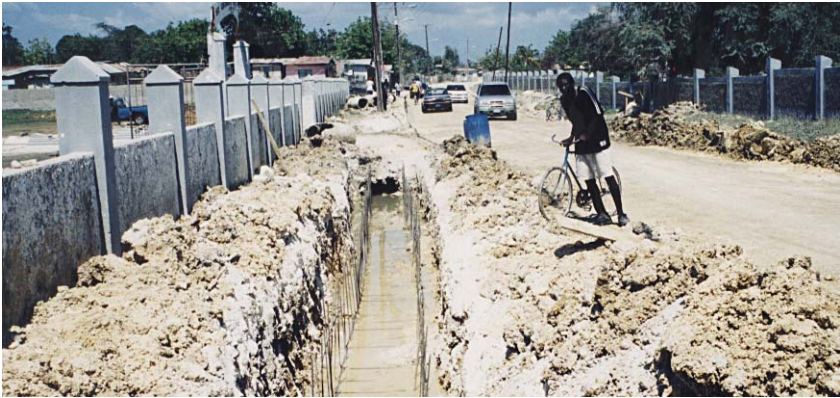
Rehabilitation of road and drainage systems underway on Dalling Street, Westmoreland.
