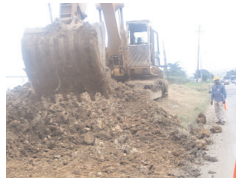
Bogue Road – (St. James) Construction work to widen the carriageway
