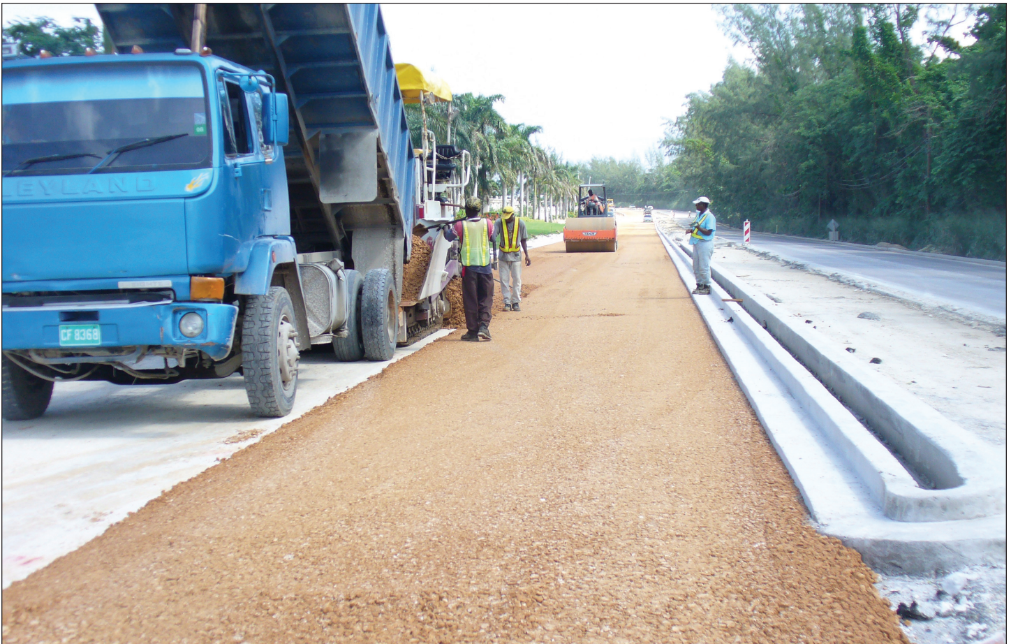
Base course being laid in the vicinity of the Iberostar Hotel (Segment 2A of the North Coast Highway)
