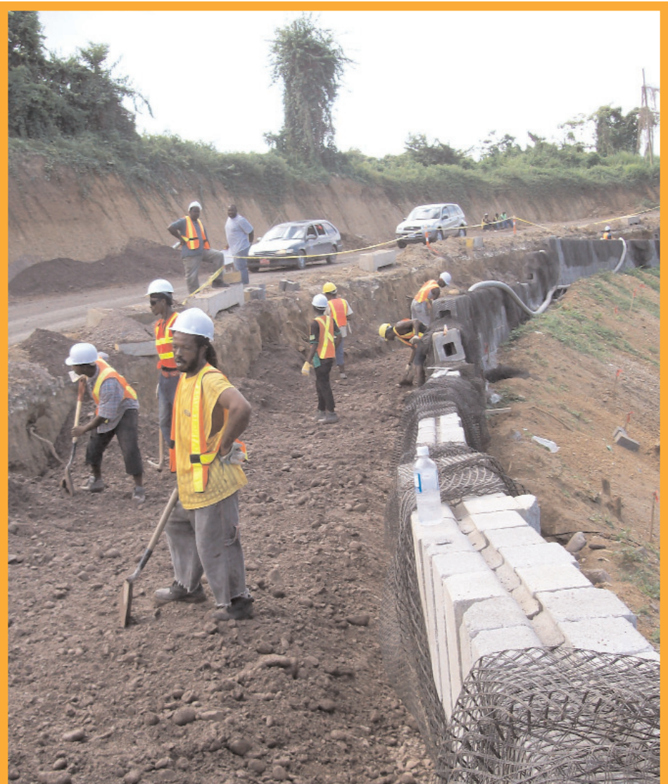
Workers backfilling a retaining wall on Segment Three of the Northern Coastal Highway Improvement Project from Ocho Rios, St. Ann to Port Antonio, Portland. Over 4,000 meters of retaining walls are being built as part of this $5.6 billion 96 kilometer roadway.
