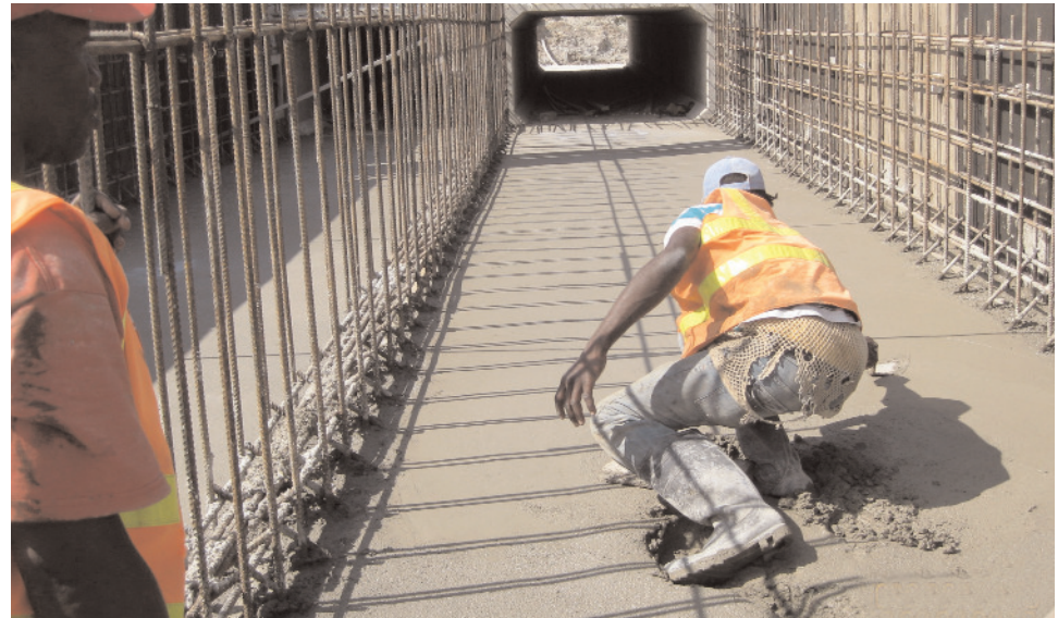
A labourer, contracted to Surrey Paving and Aggregates Ltd. puts the finishing touches to the floor slab of this double cell box culvert. This drainage system was constructed in the vicinity of Pye River cemetery in St. James under Segment 1A of the N.C.H.I.P.
