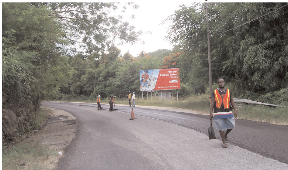
Workmen assisting with the Micro-surfacing of a roadway in St. Elizabeth
