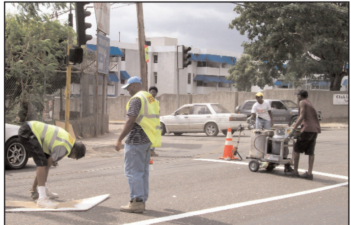
Road Marking exercise being carried out by NWA's Traffic Department
