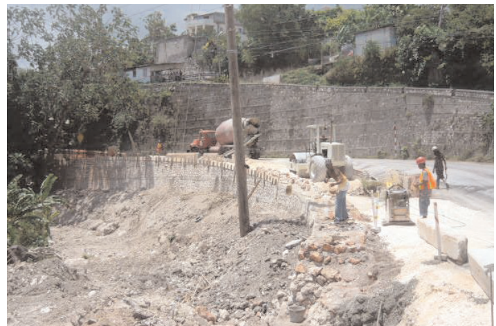
Retaining Wall being constructed to facilitate the widening of the approach road to the Steer Town Bridge
