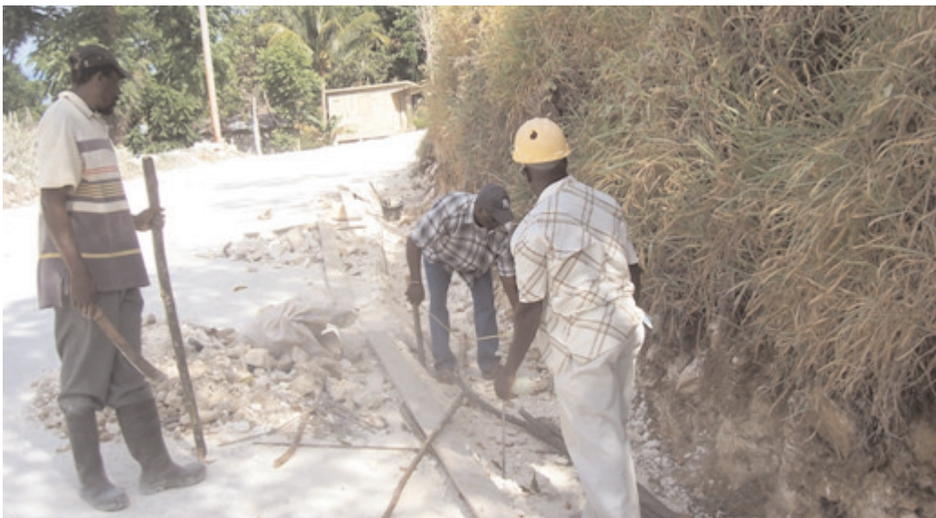
Workmen setting the levels in preparation for the construction of a V-shaped drain.
