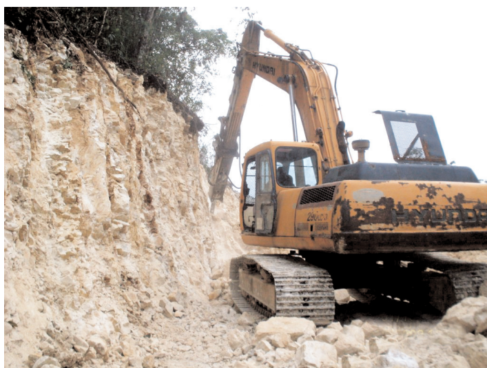
Excavation of rock formation to facilitate the construction of one of two box culverts which will be constructed in Johns Hall St. James.
