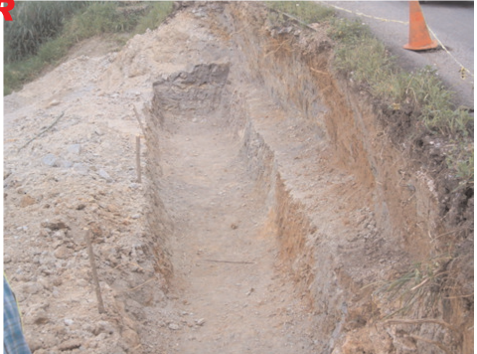
Excavation for Retaining Wall, Cane shop to Skull Point
