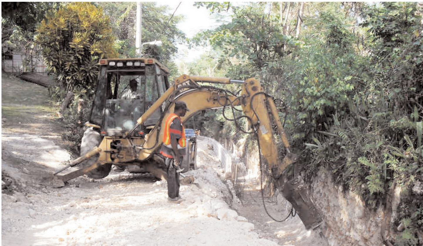
The operator of this Jack Hammer is in the process of excavating rock formation along a section of the Palmyra to Cornwall roadway in East Central St. James. The rock formation is being excavated as part of efforts to construct a concrete 'U' drain along the roadway.
