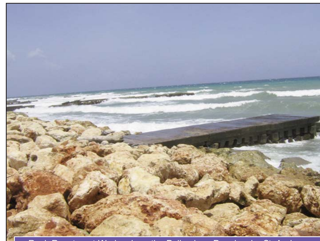
Rock Revetment Works along the Palisadoes Penninsula, St. Andrew
