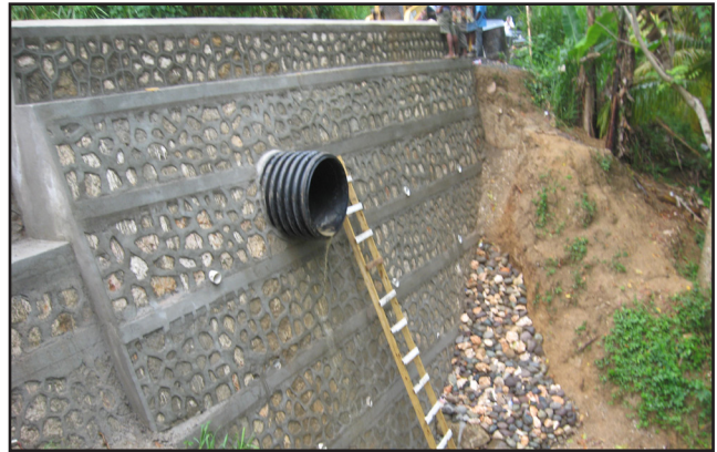
Completed Retaining Wall and drain; Williamsfield - Glengoffe, St. Andrew
