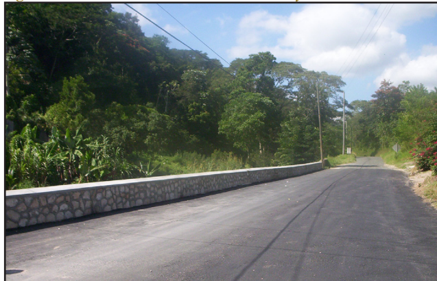
Completed Random Rubble Wall and road reinstatement; Trout Hall, Clarendon
