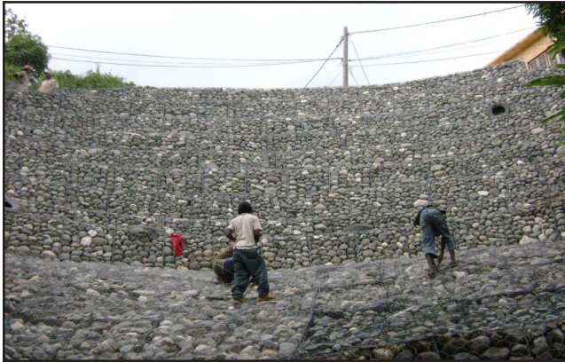
Completed Gabion Wall; Papine to Hardwar Gap, St. Andrew
