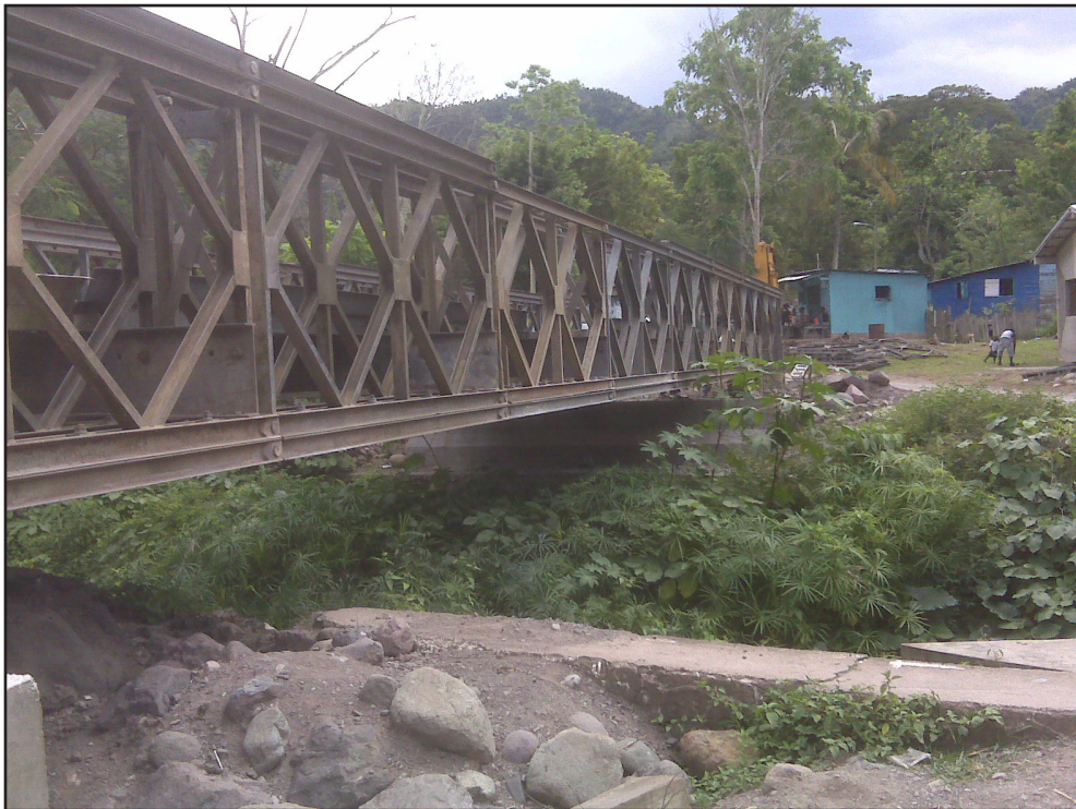
Bailey Bridge installed at Gobay, St. Catherine
