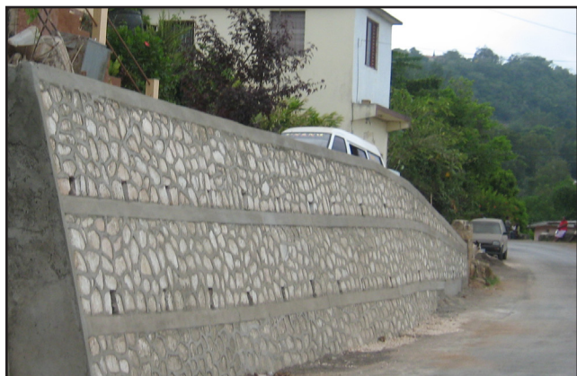
Completed Random Rubble Wall; May Pen - Spalding, Clarendon
