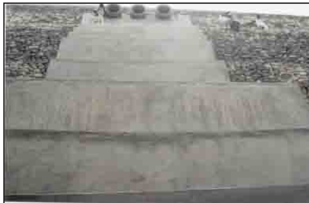
Completed Retaining Wall Cascade (The Buff Bay Valley)
