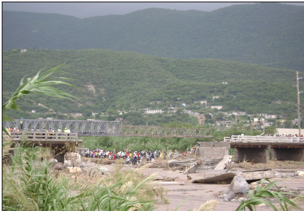
A badly damaged Dry River Bridge, St. Andrew being retrofitted with a Bailey Bridge in order to allow access in and out of Kingston. The Bridge was damaged by Tropical Storm Gustav in 2008
