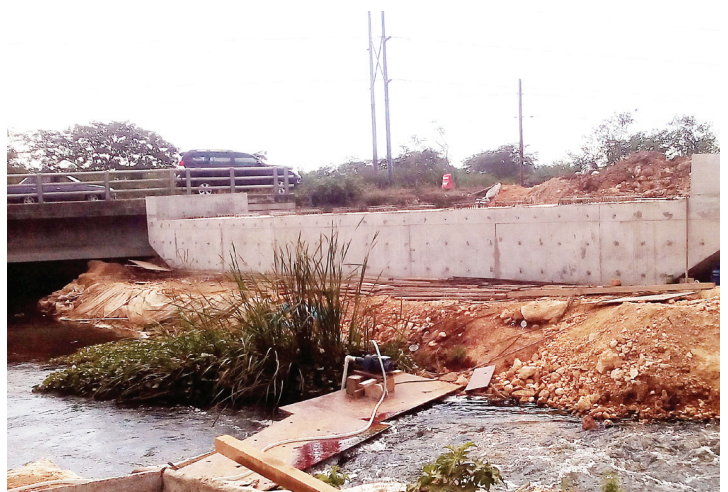
A section of the abutment of the new Fresh River Bridge
