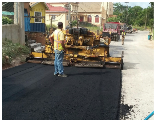
Asphaltic Concrete being laid along the Golden Grove roadway
