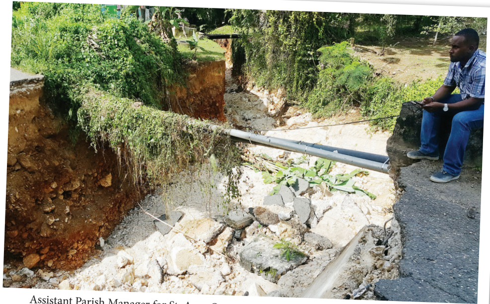
Assistant Parish Manager for St. Ann, Omari Whilby surveys the damage at Dumbarton in the parish. The road was cut in two, after a bridge collapsed during the heavy rain.
