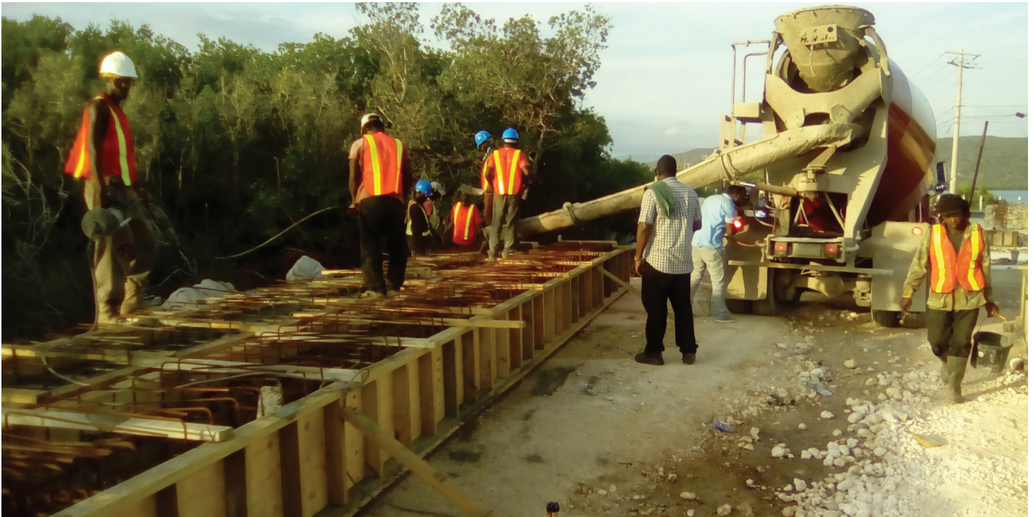
Concrete being poured for some of the Girders that will form a critical part of the Hellshire Bridge.
