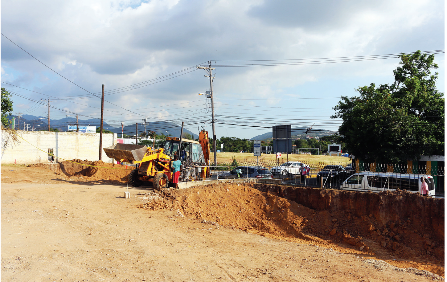
Work being carried out along Barbican Road. Boundary walls are being replaced in order to facilitate the planned widening
