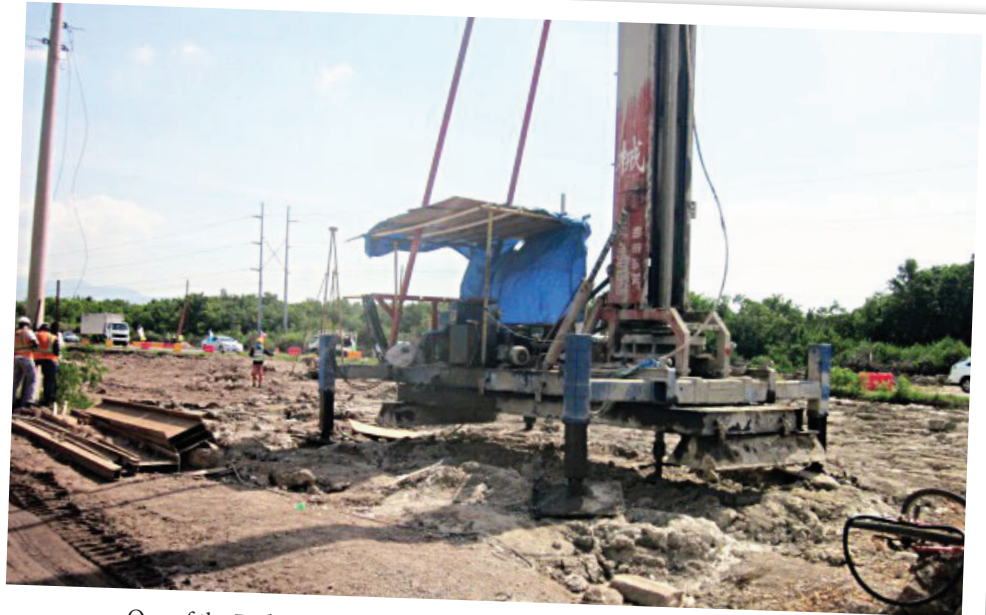
One of the Drills used to create holes to facilitate the deep pile foundation
