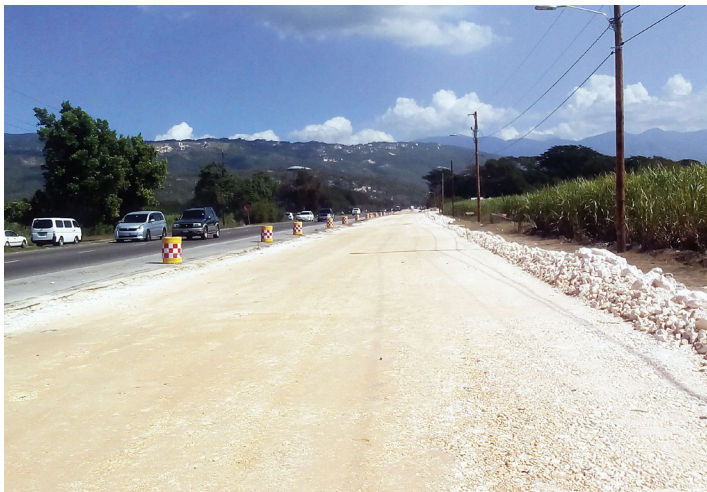
Graded material being used to fill and heighten a section of new roadway
