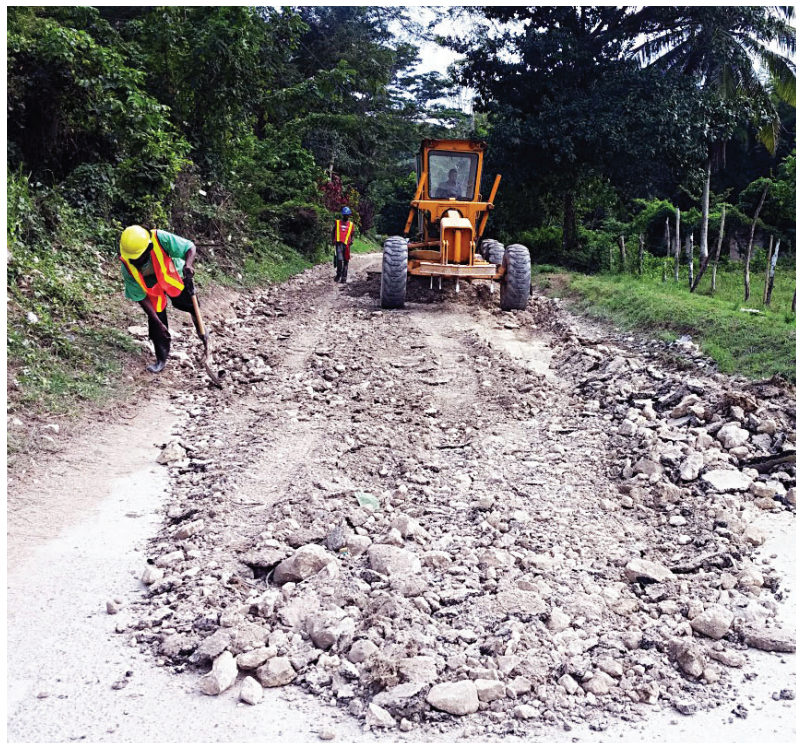
A Motor-Grader scarifying a section of the road.
