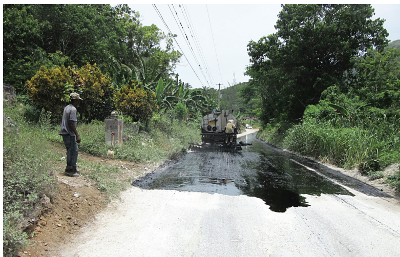
Base protection/prime coating in progress
