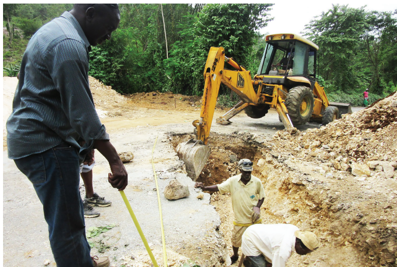
Preparation being made for the laying of a 500mm culvert along the road
