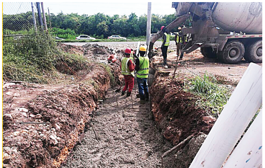
Left - Underground ducts being laid as part of plans to place street-lamps along the corridor. Right - The ducts being encased in concrete.
