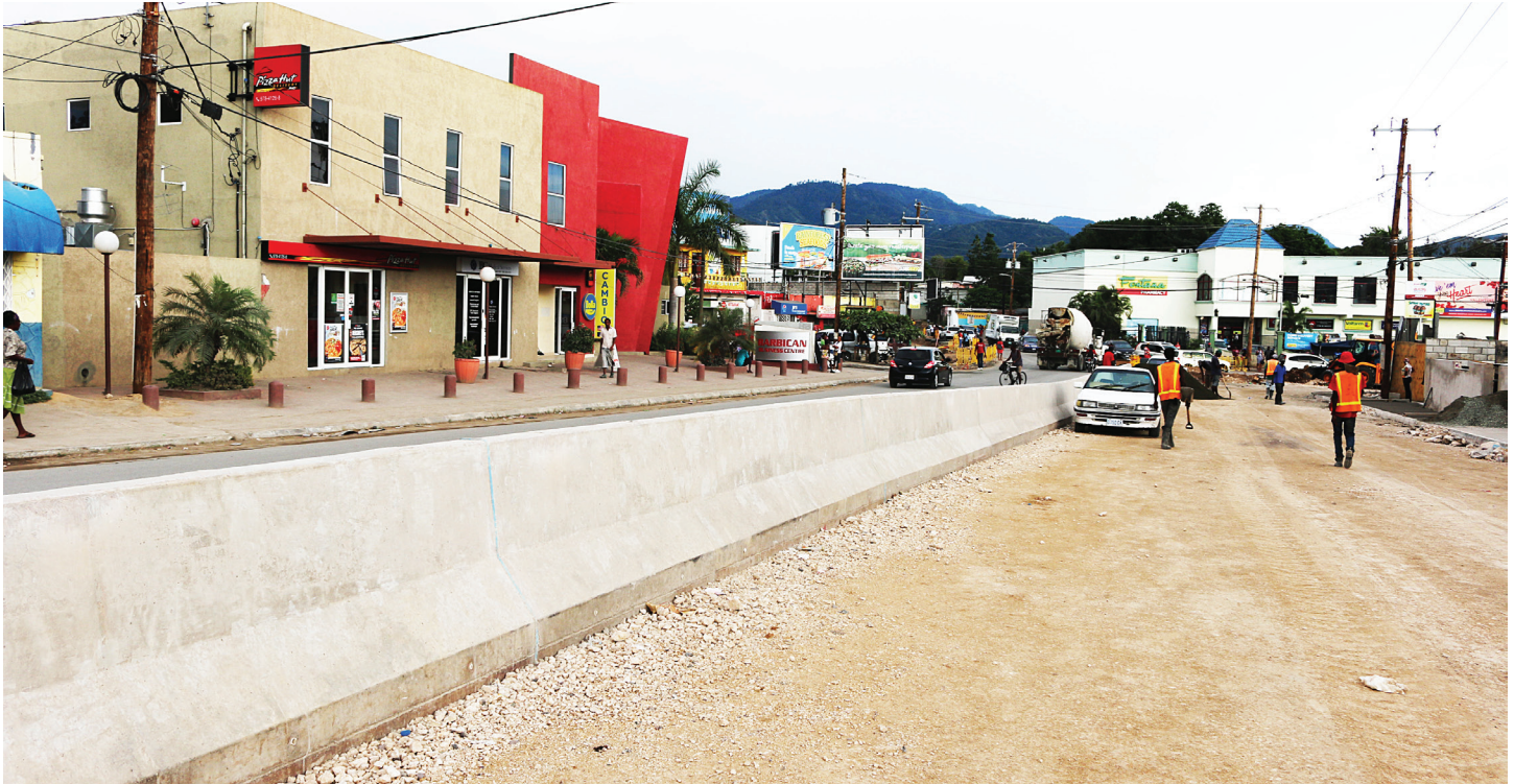
A section of the median (Jersey Barrier) being erected along Barbican Road
