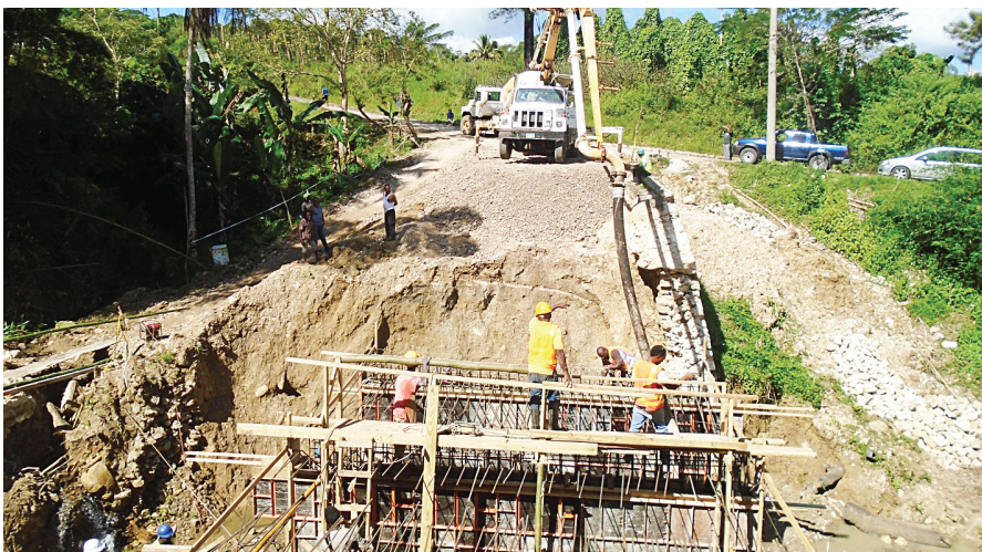
Workmen assisting with the pouring of concrete for the new box culvert
