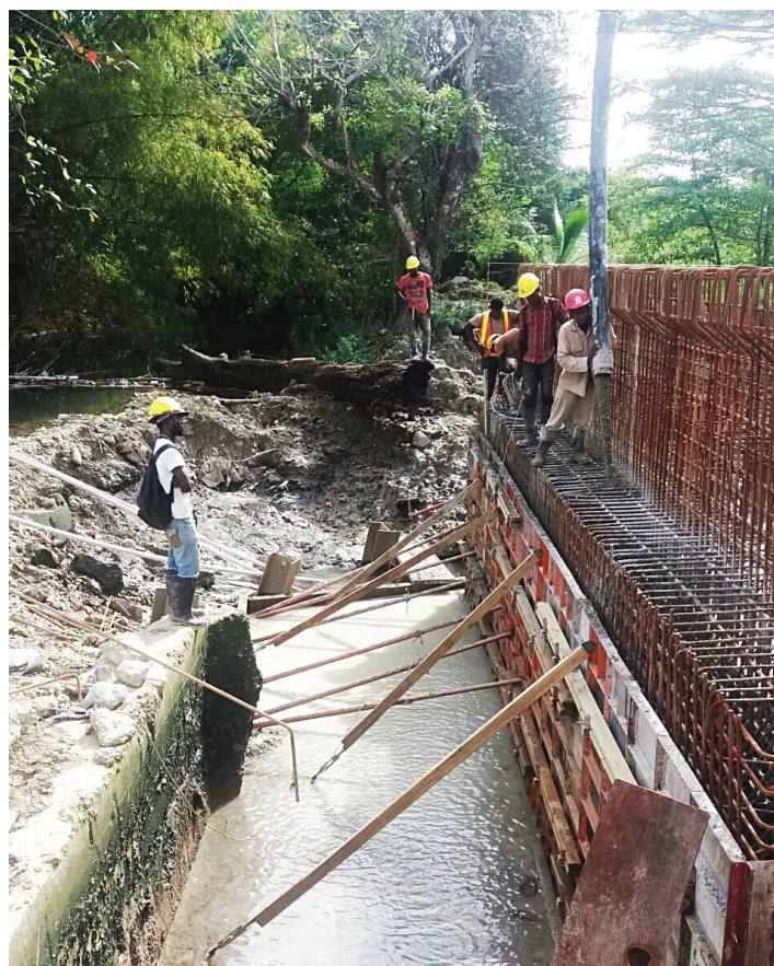
(top) - Workmen briskly pouring concrete in the formwork to start the bridge's abutment
