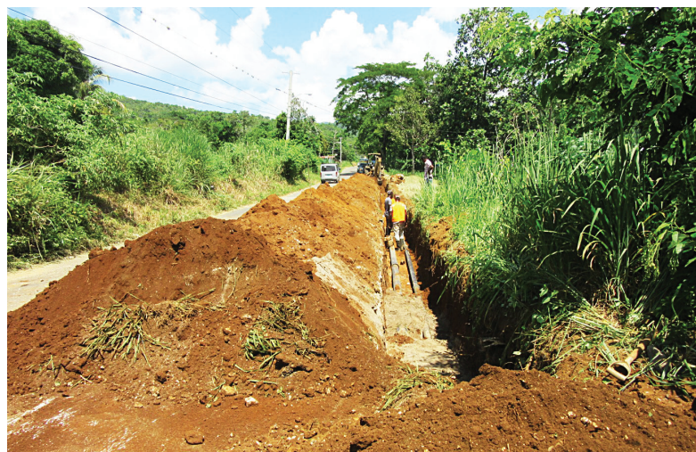
Excavation and laying of 100mm and 150mm diameter water lines
