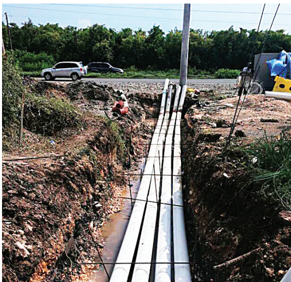
Left - Underground ducts being laid as part of plans to place street-lamps along the corridor. Right - The ducts being encased in concrete.
