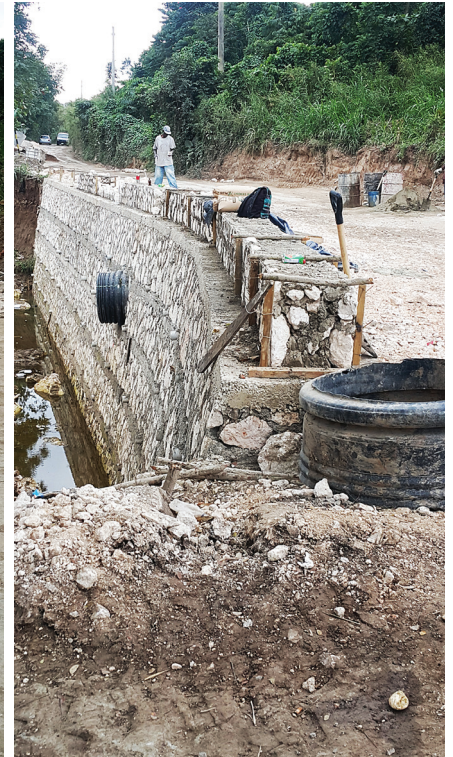
Retaining wall underway along road from Bog Walk to Riversdale
