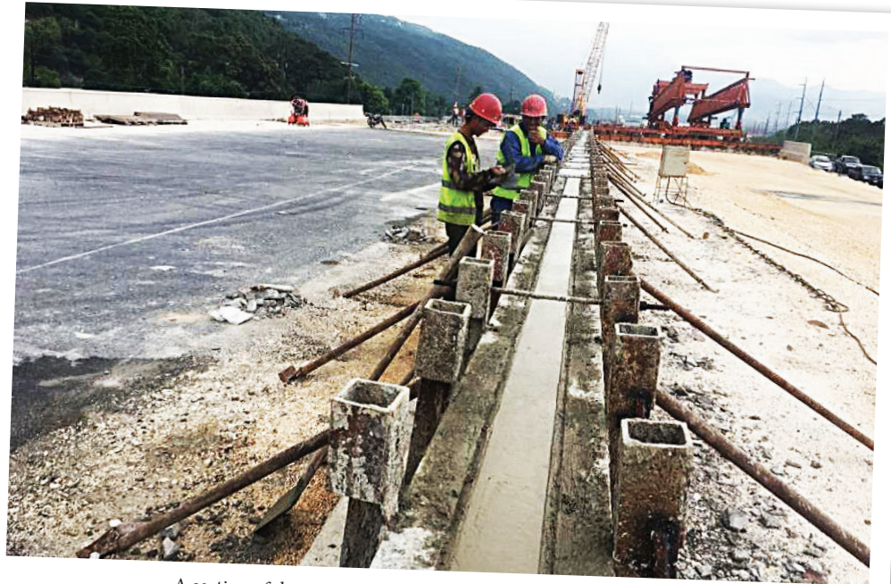
A section of the median (Jersey Barrier), now under construction
