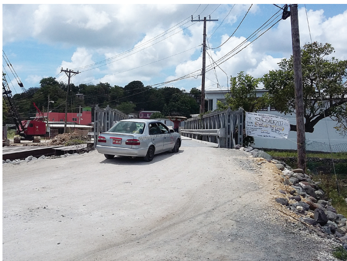
Direct access is maintained between Morant Bay and Port Morant via a temporary Bailey Bridge
