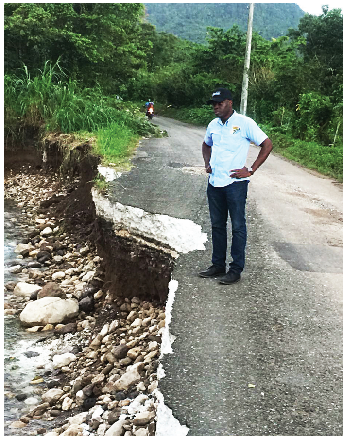
Communication and Customer Services Manager, Stephen Shaw, looks at one of the damaged areas along the road from Hope Bay to Fruitfulvale at Shrewsbury, Portland, where the river has taken away a section of the road embankment.
