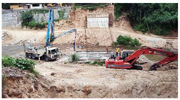
Labour and equipment worked long hours to get the structure completed. Abutments and Piers were built and soil replacement was done, as necessary.
