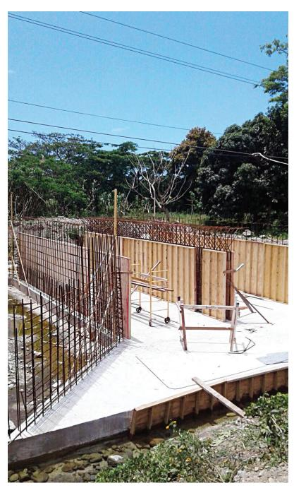
Formwork, being put in place to accommodate the concrete pour for the wing walls
