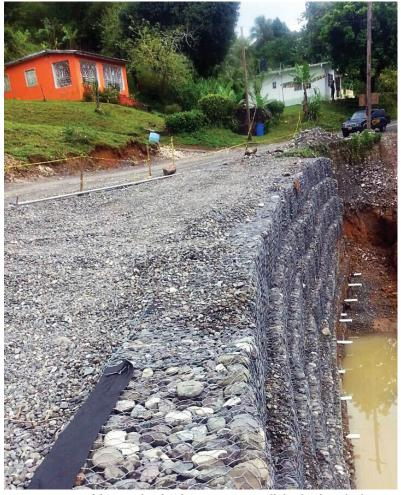
A section of the completed Gabion Retaining Wall that has been built at West Retreat
