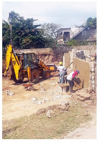
Work underway along a section of Barbican Road, where privacy walls and buildings are being removed to facilitate the widening of the corridor from two to four lanes. The project has so far employed a number of artisans, including Masons and Carpenters. In this picture, two of the Masons were photographed applying a final coat of mortar to one of the walls that have been relocated.
