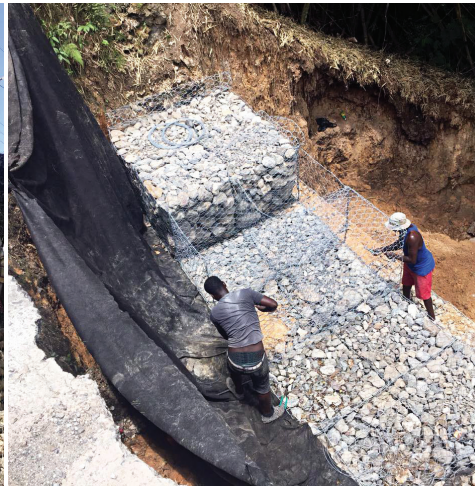
Mended: Fixing the breakaway with Gabion and Parapet Wall at Above Rocks, St. Catherine
