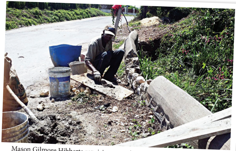
Mason Gilmore Hibberts repairing one of a number of parapet retaining walls along the roadway.
