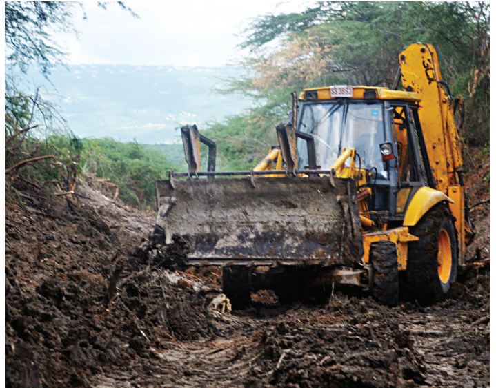
Backhoe cleaning earth drain
