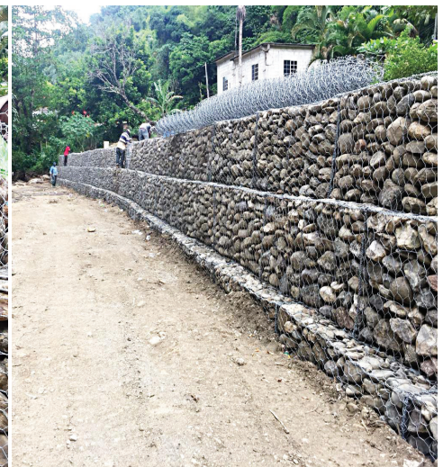
Controlling the channel; regulating storm water flow to the Sulpher River, St. Thomas
