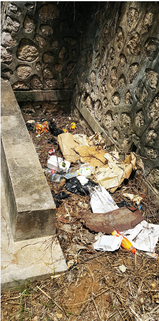
Blocked! Some of the discarded household waste responsible for the blockage of this catch basin along a main road in Trelawny
