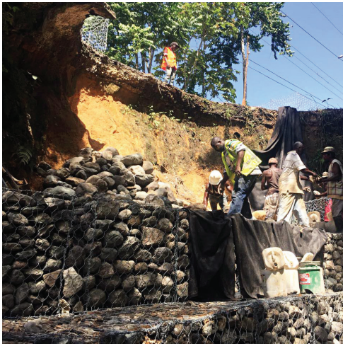
Mended: Fixing the breakaway with Gabion and Parapet Wall at Above Rocks, St. Catherine
