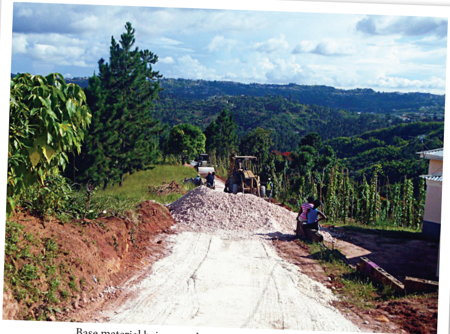
Base material being put down along Long Fearon PC Road
