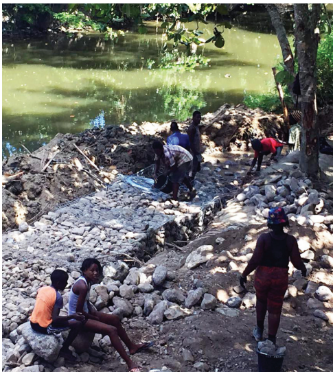
Mended: Fixing the breakaway with Gabion and Parapet Wall at Above Rocks, St. Catherine
