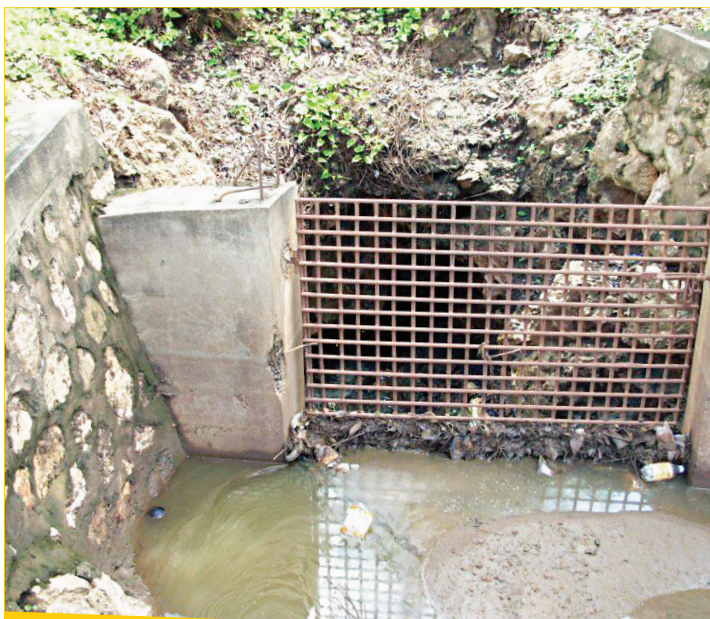
Drain with Trash Rack in front of sink hole near Big Pond, an existing but inadequate drainage feature
