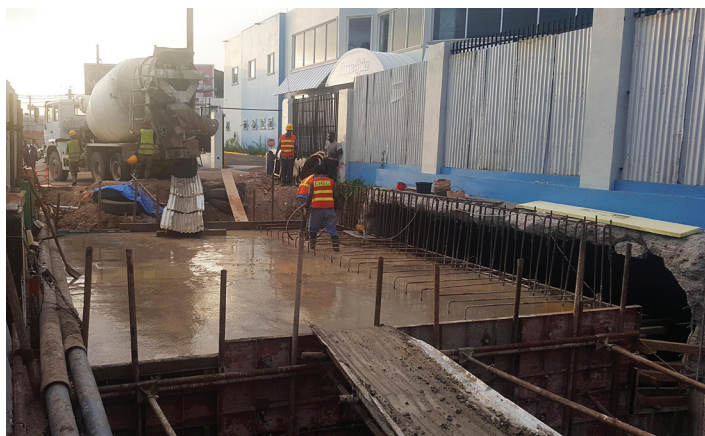
Ongoing works on casting one of two deck slabs on the Bustamante Bridge which will extend the structure by 6 meters on its northern side, including a 1.5 meter sidewalk.
