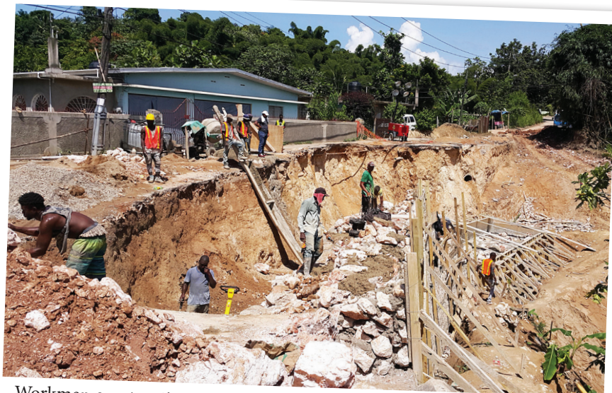
Workmen constructing one of the three walls that had to be built in order to restore the embankment that formed part of the Mount Ogle main road.
