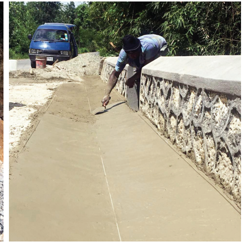
Mended: Fixing the breakaway with Gabion and Parapet Wall at Above Rocks, St. Catherine
