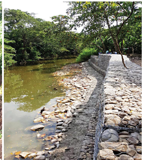
Mended: Fixing the breakaway with Gabion and Parapet Wall at Above Rocks, St. Catherine
