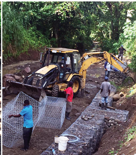
Training the river; cutting out the bend in the Otrum River, St. Mary
