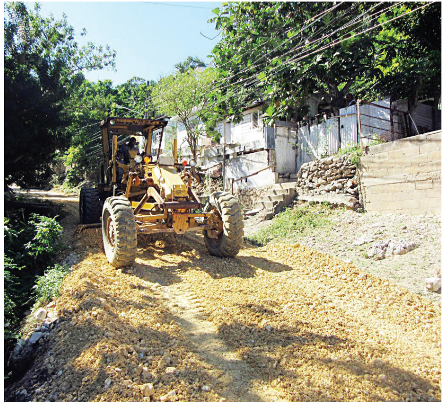
Base formation works underway along the Capital Heights roadway in St. James.
