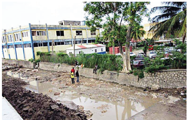
A section of damaged invert under repairs.
