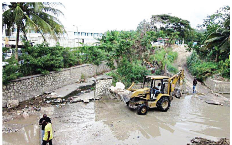
A backhoe transports stones which will form part of the engineered fill, used to backfill the areas being repaired.
