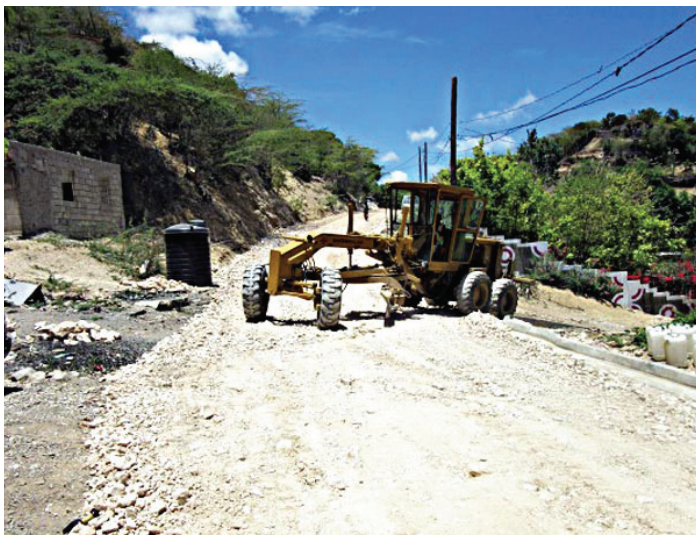
Base preparation for Double Surface Dressing (DSD)
