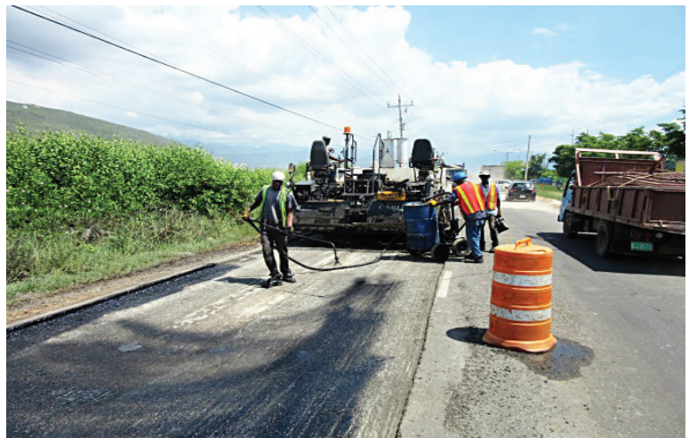
Repaving of damaged section of Mandela Highway
