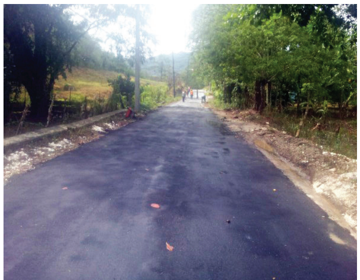
Sheet patching along the Grierfield to Moneague roadway
