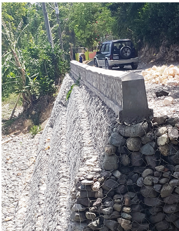
A completed section of a gabion retaining wall along the Spring Garden main road in St. Thomas. A second phase of the works is slated to take place during the next quarter of the financial year.
