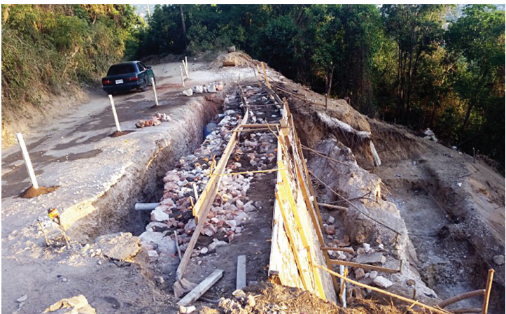
Jacks Hill Retaining Wall Under Construction
