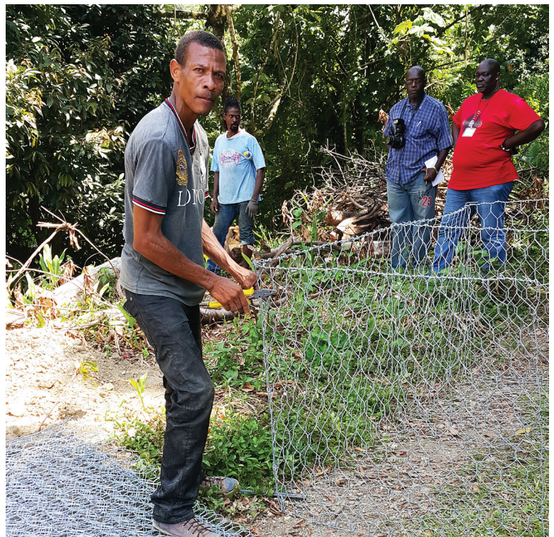
A workman preparing Gabion Baskets
