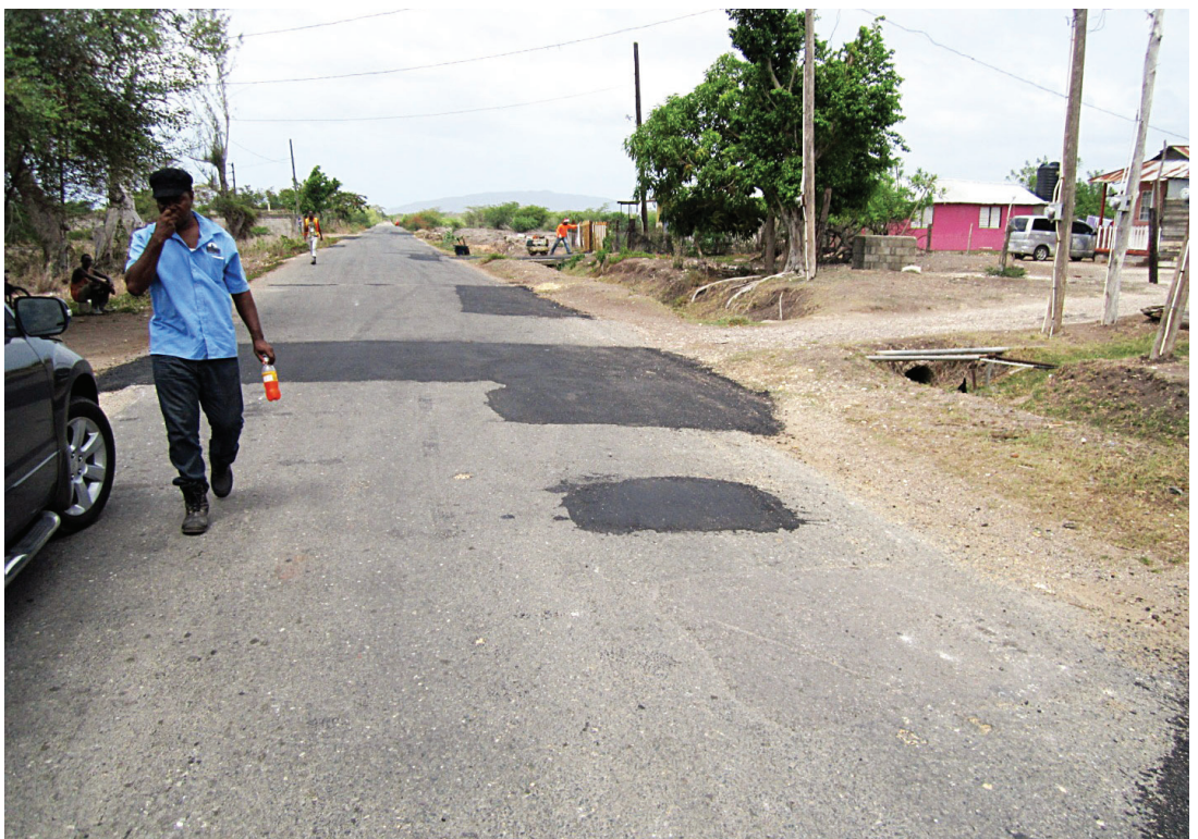
Hotmix Patching at Jacob Hut to Milk River
