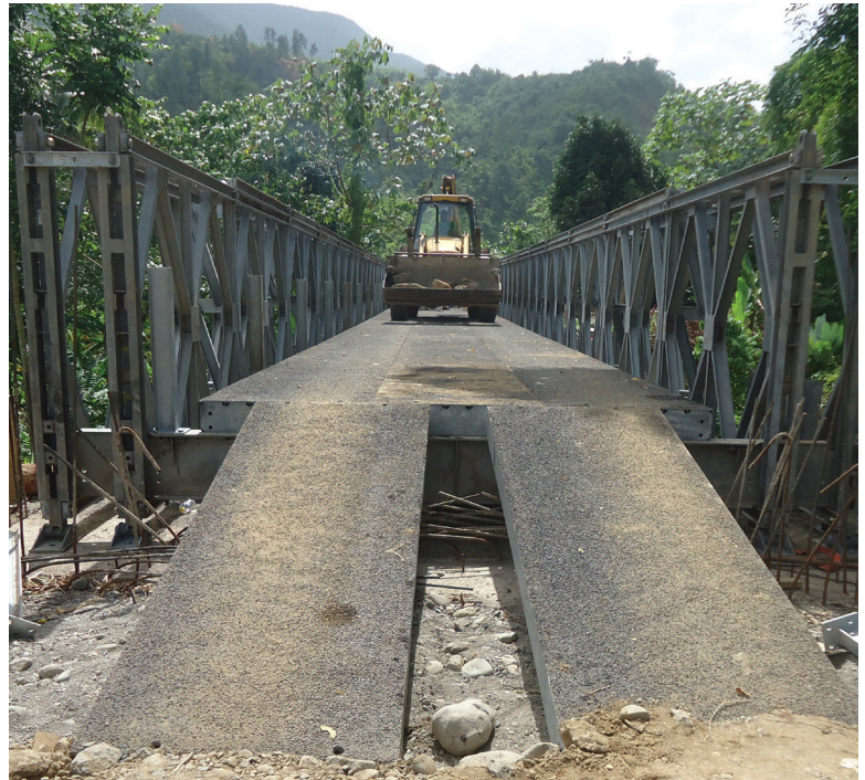
Bridge number one, hours after being launched, facilitating the passage of a heavy equipment on the site
