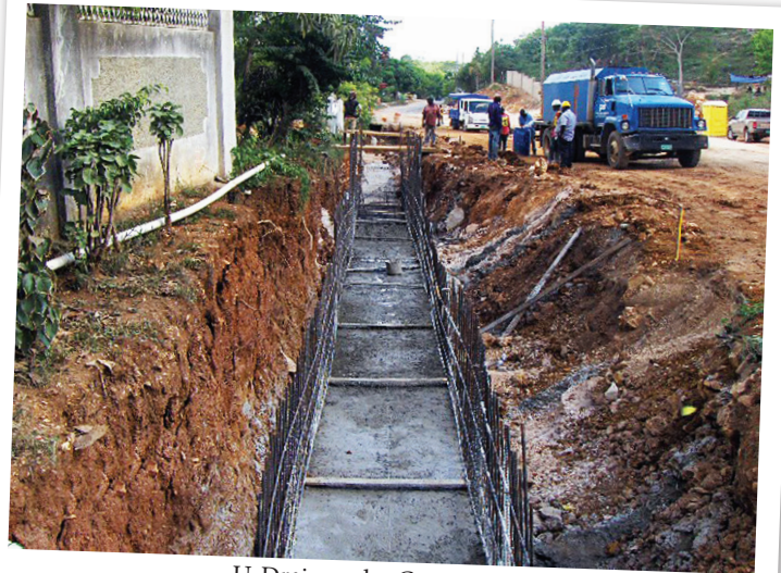
U-Drain under Construction
