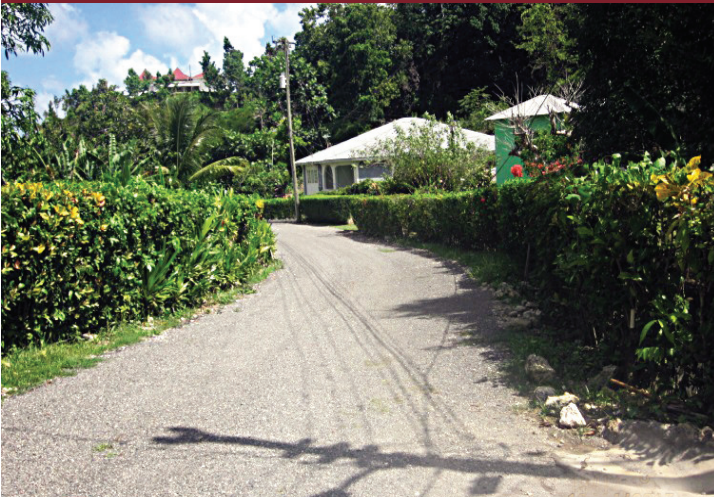
A section of Pompey Lane in Portland that was double surface dressed
