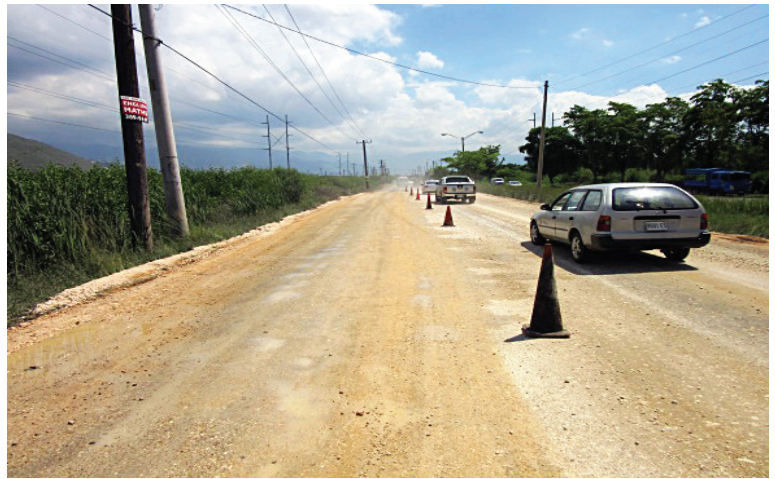
Base course completed along the damaged section of Mandela Highway
