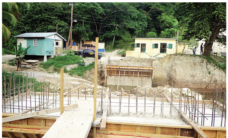
The abutments of the Latium Bridge in St. James
