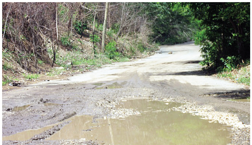
Blocked drains that caused inundation and scouring to road surface
