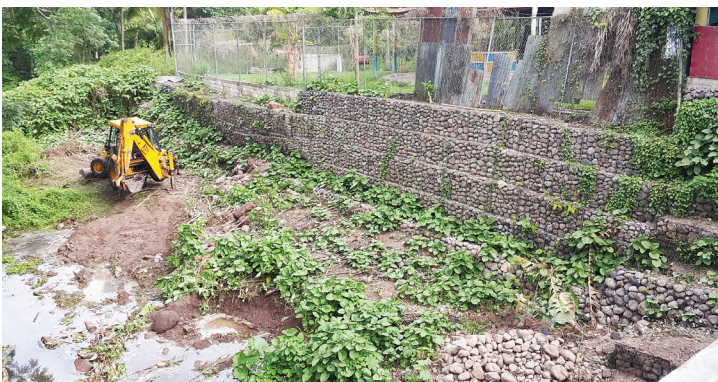
Protective work being done within a river channel in Pennant, Clarendon. Sections of the gabion retaining wall had been undermined by flood rains.
