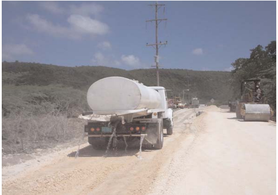
Base material being compacted
