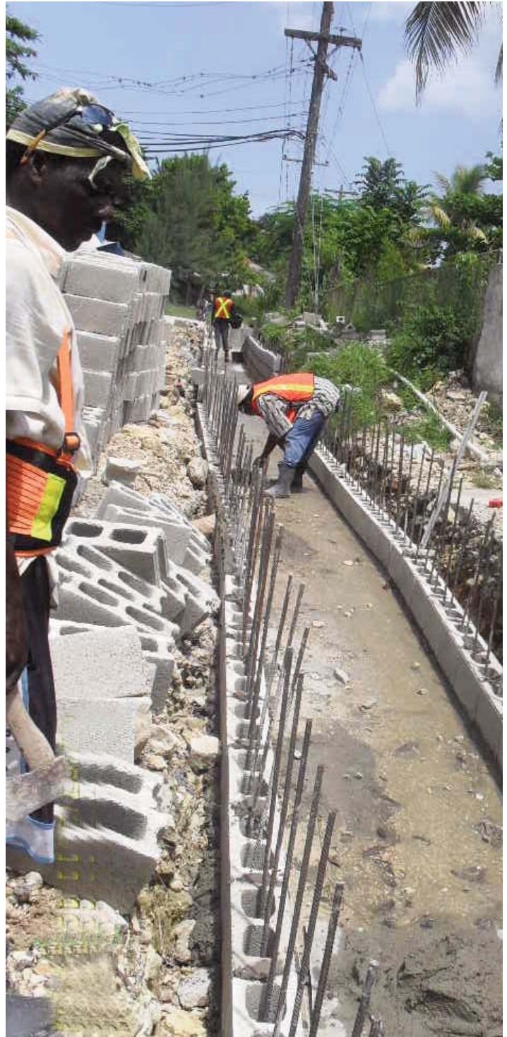
Workmen constructing a concrete 'U' drain along a section of the Granville to Retirement roadway in St. James. This roadway is being rehabilitated under the Jamaica Development Infrastructure Programme (JDIP).
