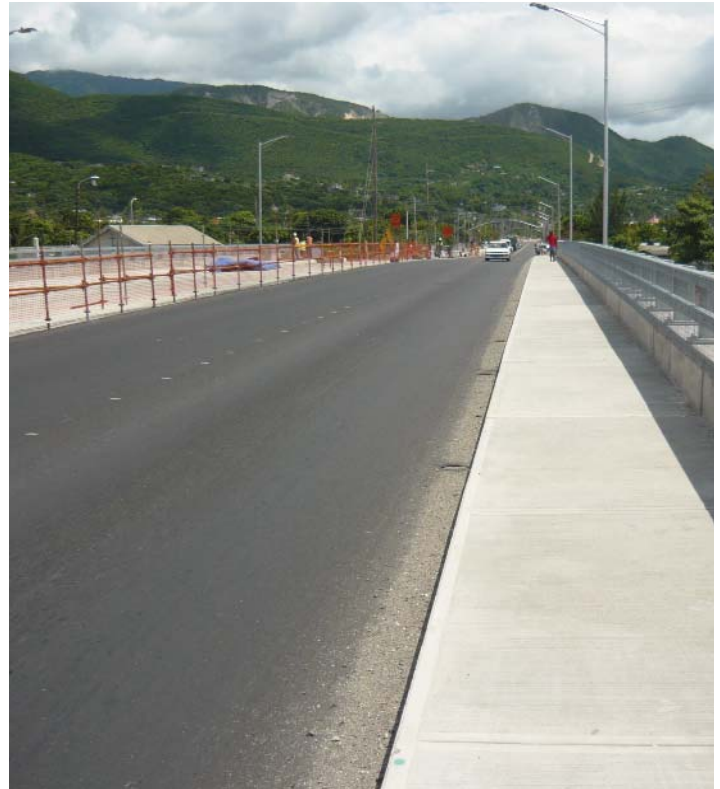
Opened - two southern lanes of the new Dry River Bridge in St. Andrew
