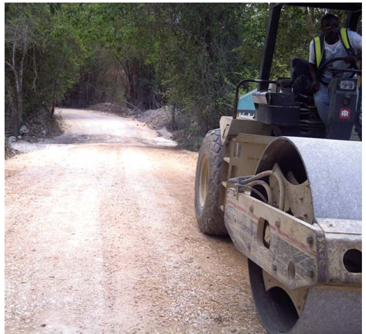
Martha Brae to Kinloss - Base course material being rolled
