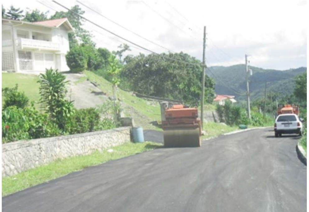
A section of one of the roads recently completed
