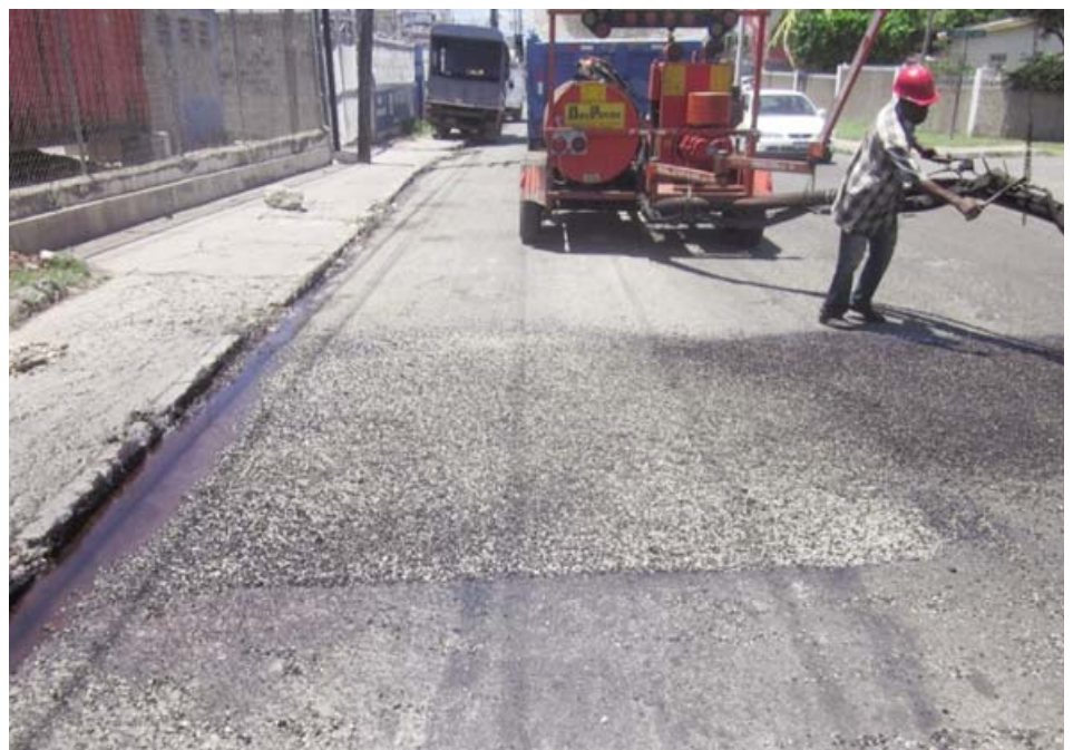
Spray Patching in Progress along Hagley Park Road in Kingston
