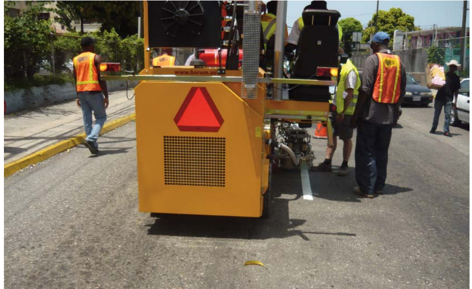
Road Marking Machine and Crew at work
