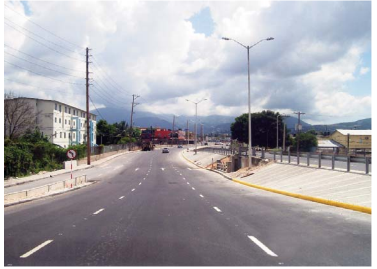
Red Hills Overpass
