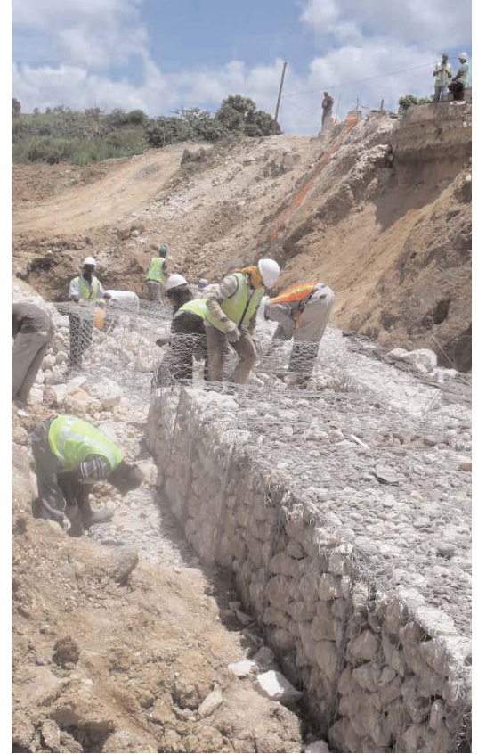
Warsop - Thompson Town - Gabion Retaining Wall under construction
