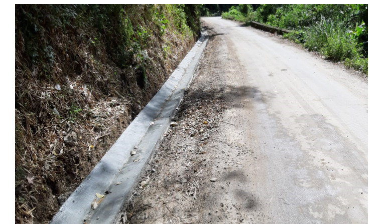
A V-drain which was constructed along the Riley roadway in Hanover.
