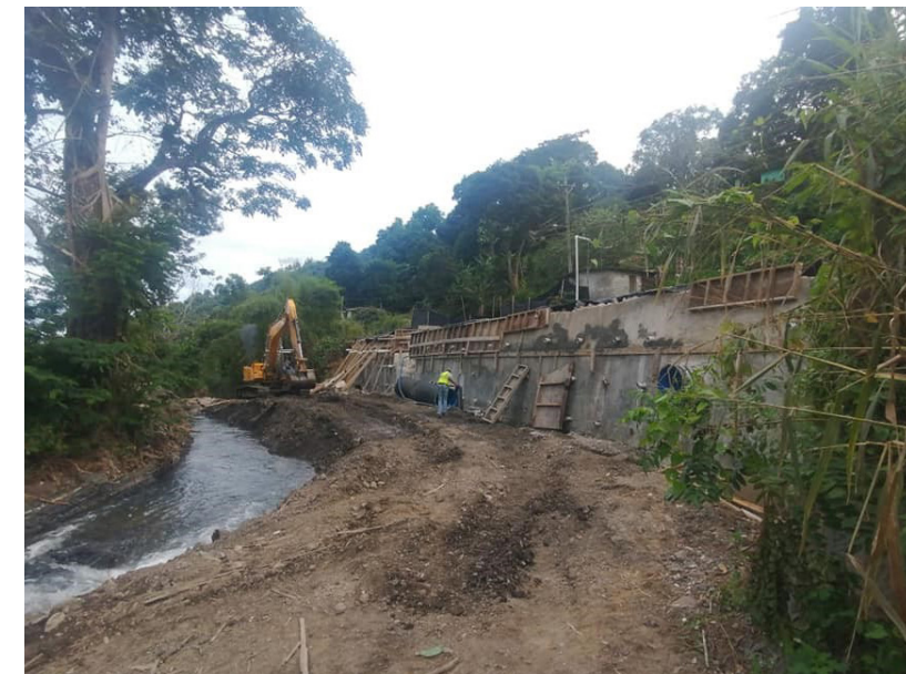
A view of the five-tier cyclopean masonry retaining wall at Cedar Valley.
