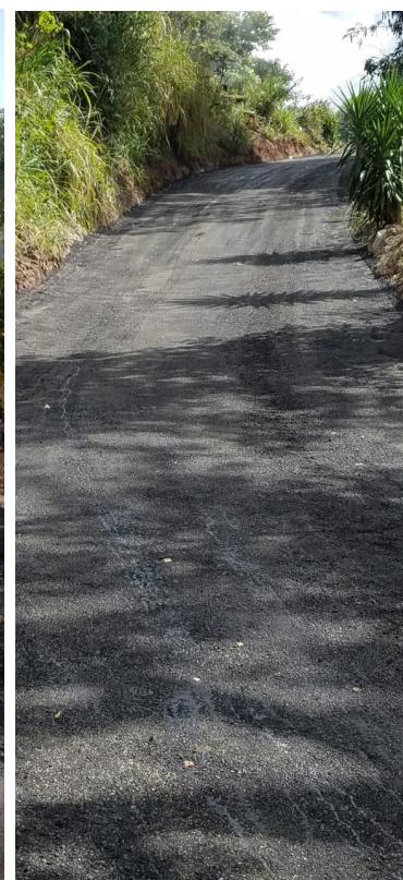
Savage Pen Road being paved with asphaltic concrete
