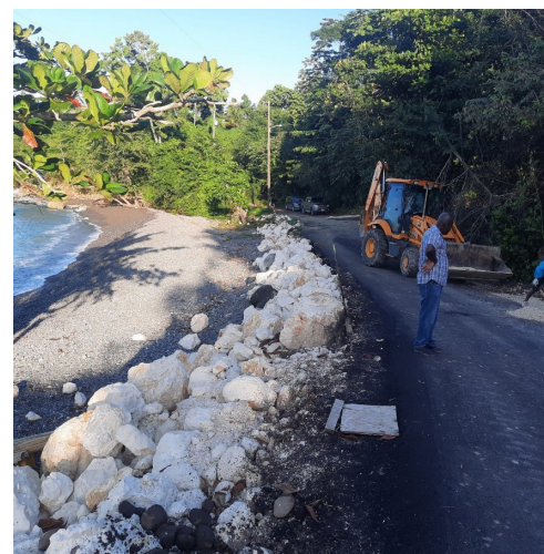
Shoreline protection works with the use of boulders
