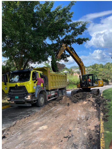
Excavation and preparation of roadway for the construction of the concrete pavement
