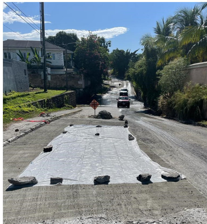
The concrete curing process being employed as part of the process
