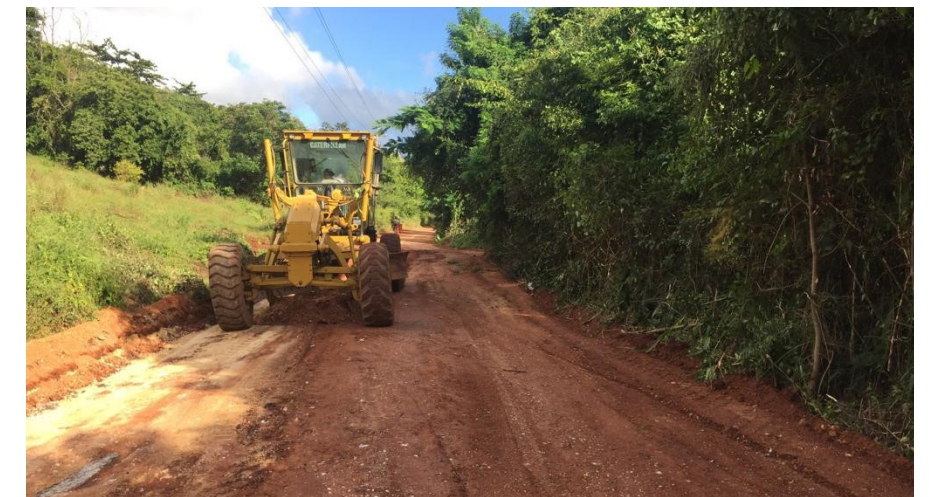
Scarifying and Preparation of Formation
