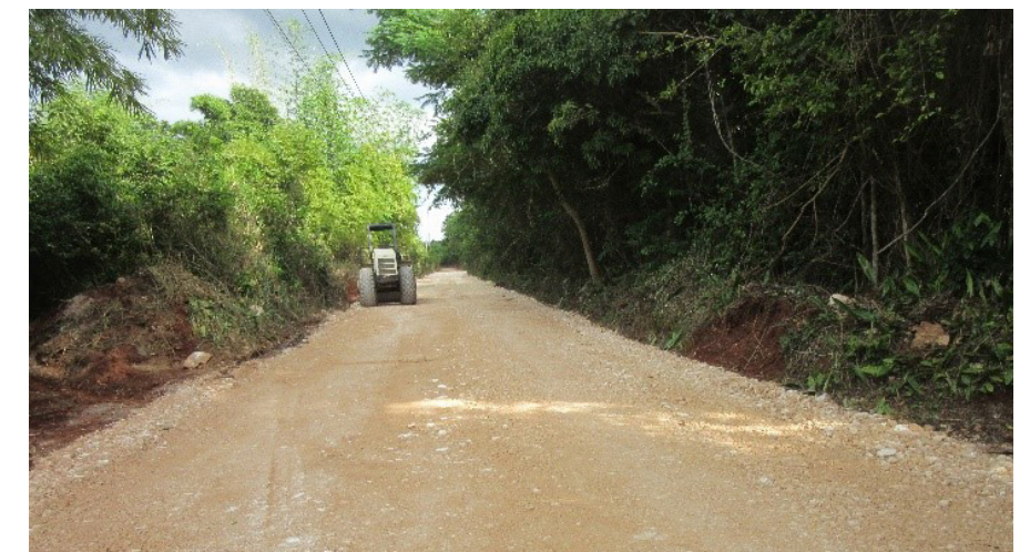
Compaction of work surface
