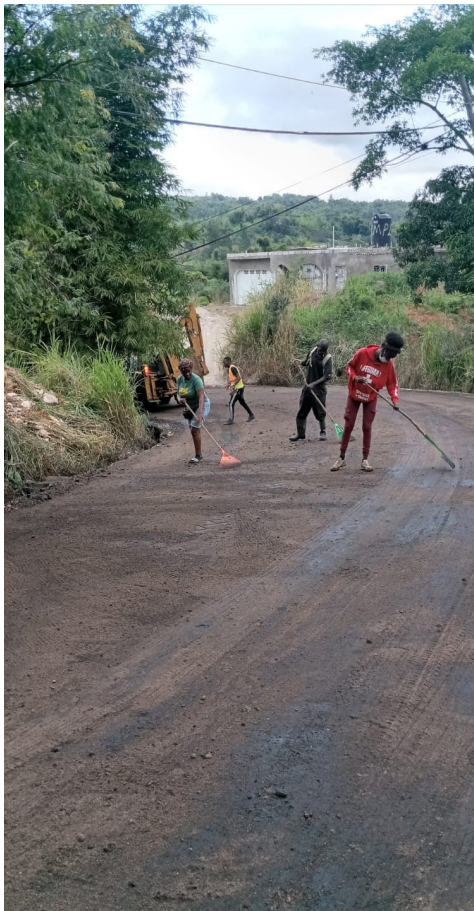
Cleaning road surface before Overlay works
