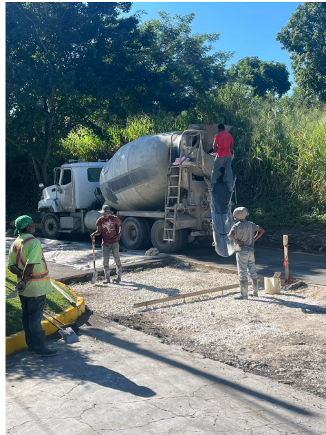
Excavation and preparation of roadway for the construction of the concrete pavement
