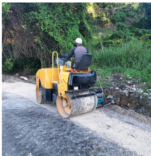
Soft spots being corrected as part of the rehabilitation of Wharf Lane
