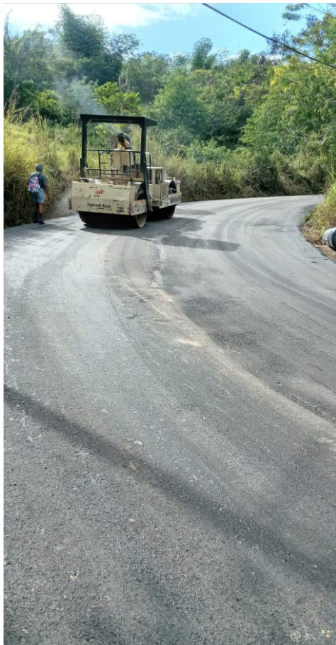
Compaction-Overlay Works
