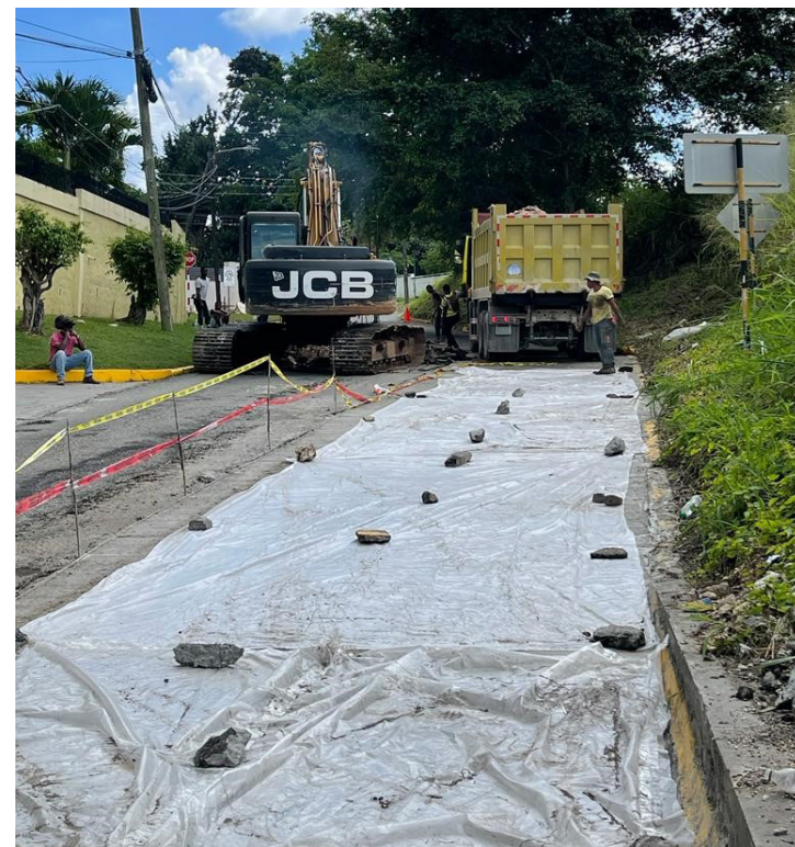
The concrete curing process being employed as part of the process
