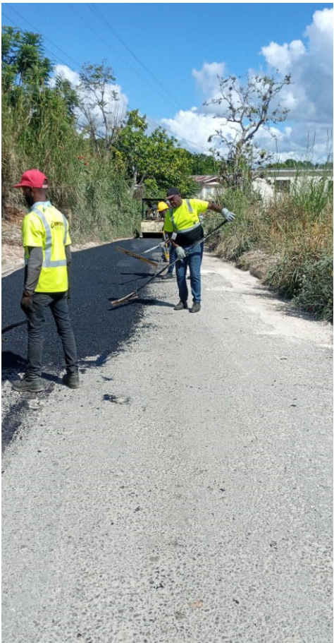
Asphaltic Concrete Overlay Works with Lutemen.
