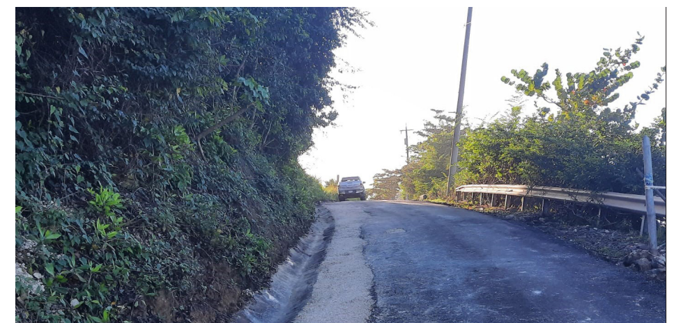
V-drains that were constructed as part of the project
