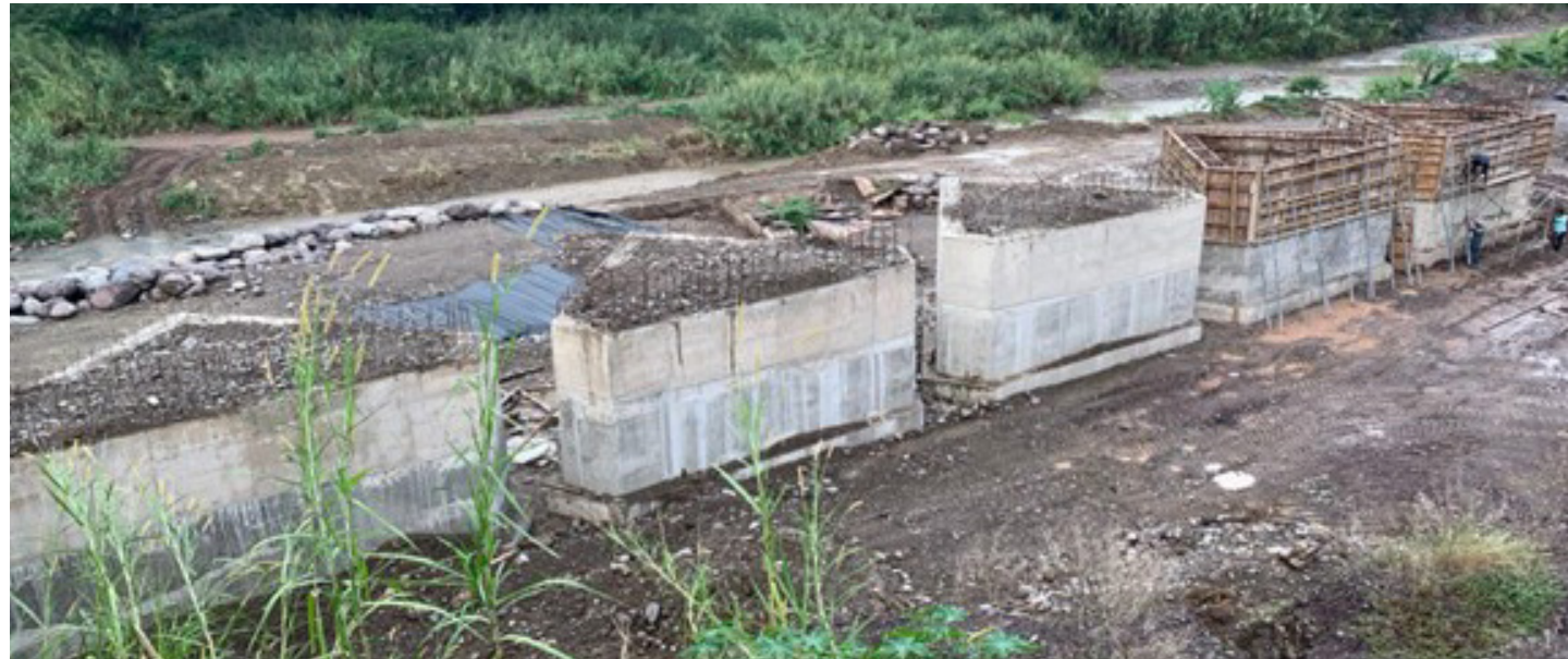
Formwork being installed for the second lift of armour block
