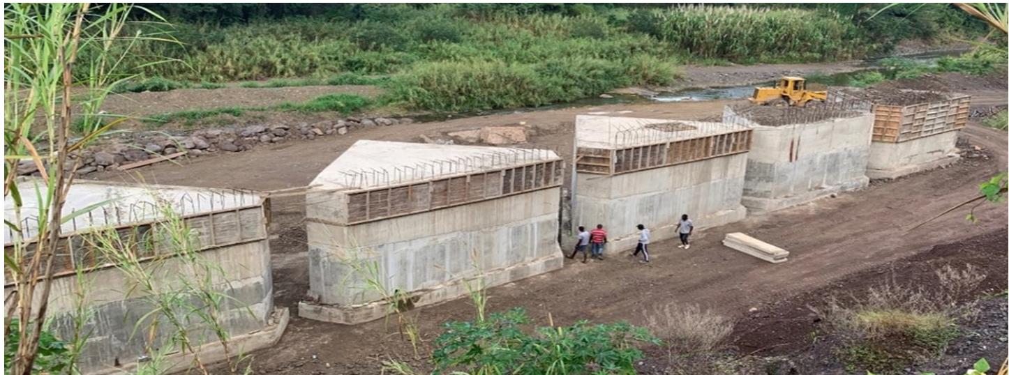
Several of seven diamonds which make up armour block wall
