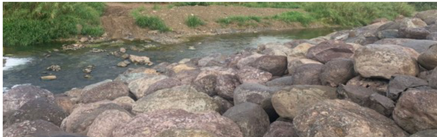
Boulders used to stabilise and protect the hillside – Boulder Protective Works
