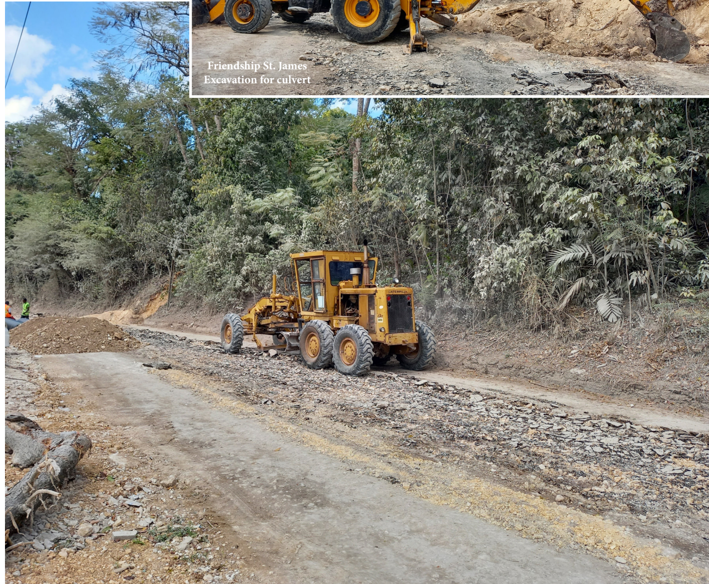
Scarifying and reshaping of the Friendship roadway in St. James
