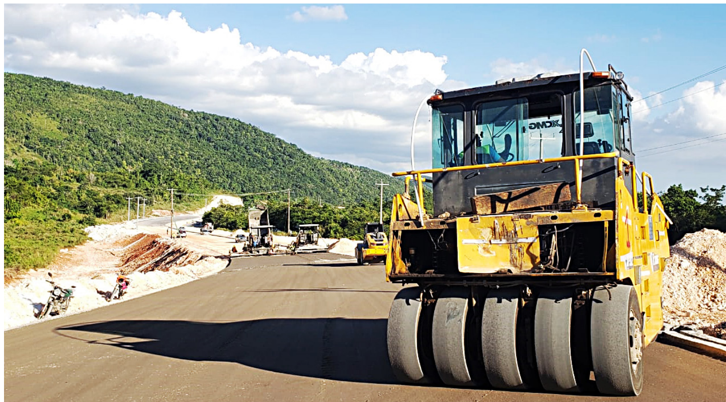
Compacting Roller at work
