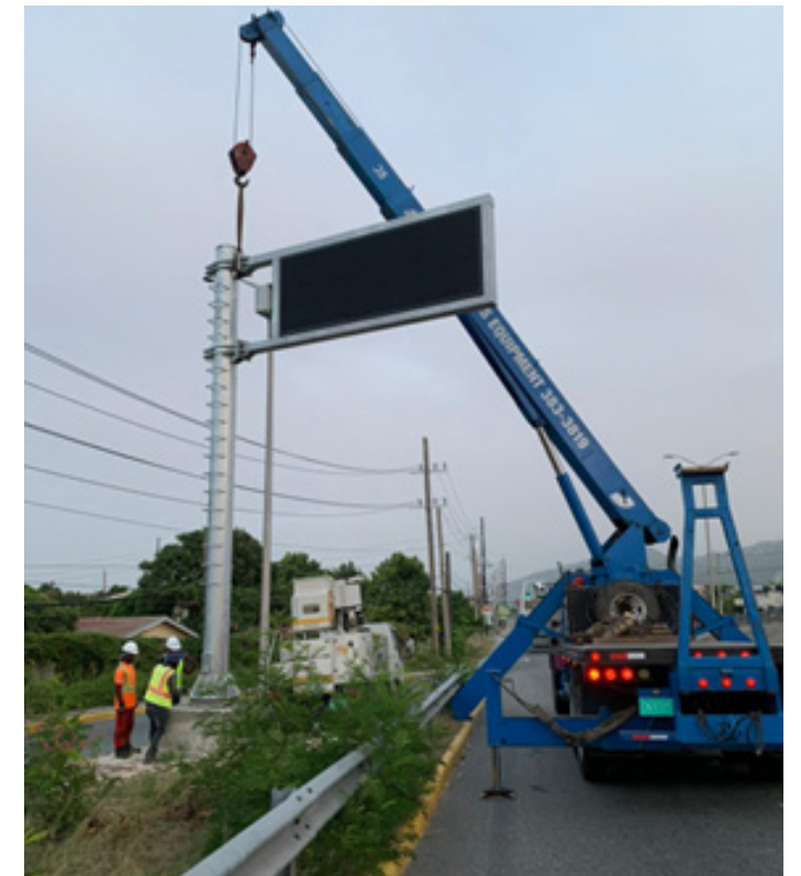
Variable message sign being installed at Dunrobin Avenue/Red Hills Road in Kingston
