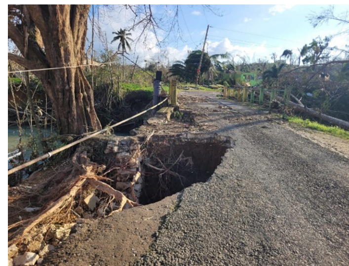
Grange – Friendship, Westmoreland. A section of the approach to this bridge was severely undermined following the storm.
