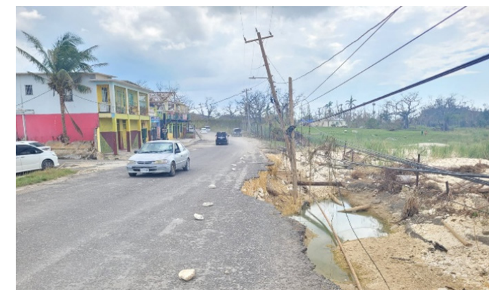
Scouring along a section of the Goodens River to Glasgow roadway in Westmoreland
