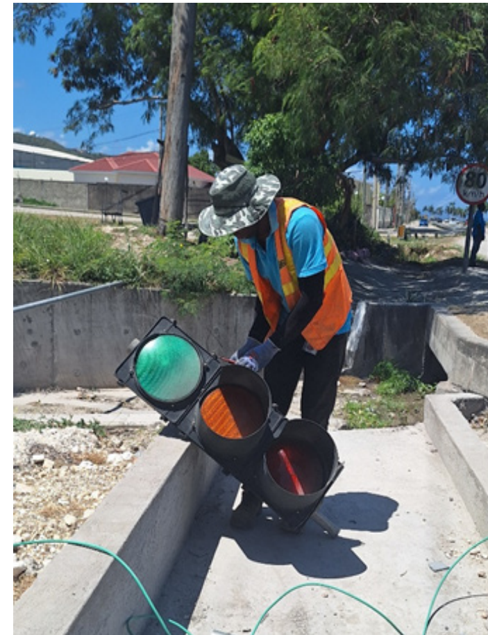
Quacy makes adjustments to a traffic signal head.
