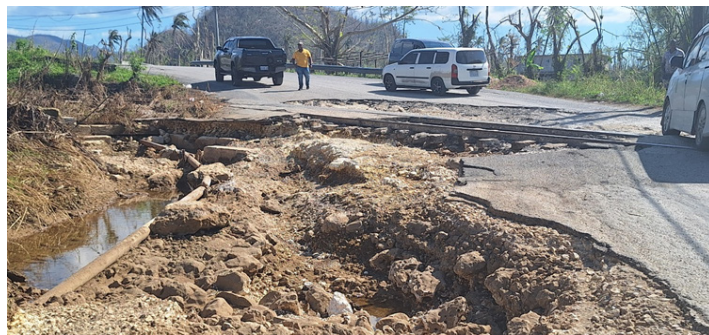
A scoured section of the Seven Rivers (Montpelier- Cambridge) roadway in St. James. This section was inundated by feet of water several days after the storm.
