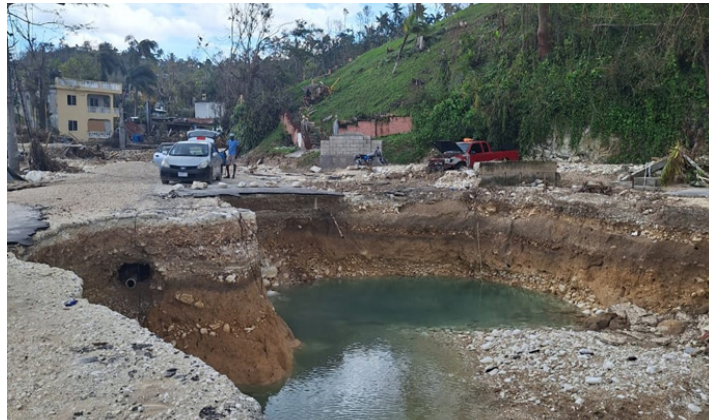
An eroded section of the Chelsea roadway in Irwin, St. James which was severely eroded following Hurricane Melissa. The roadway has since been temporarily restored.
