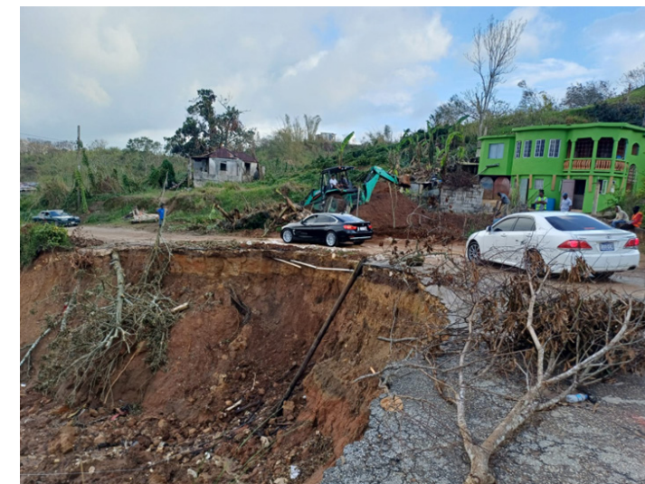
A massive breakaway along a section of the Stetting to Highgate Hall roadway in the vicinity of the Lowe River community.
