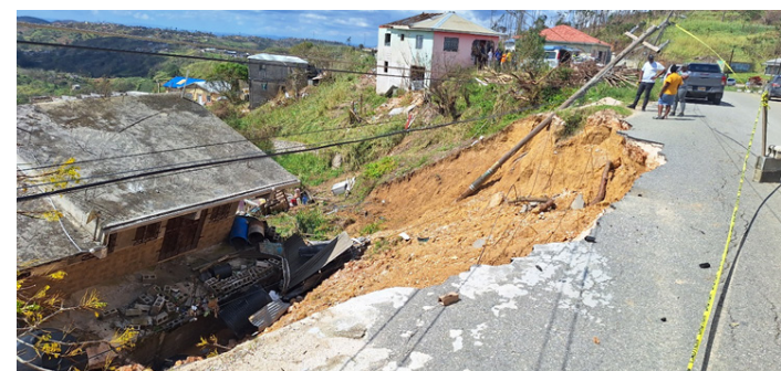
Stetting - Highgate Hall Trelawny This concrete two story dwelling buckled under the pressure of Hurricane Melissa, slipping several metres after the roadway was undermined.
