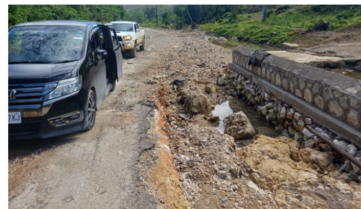
Salt Marsh - Kent, Trelawny. The roadway was severely scoured following the passage of the Hurricane
