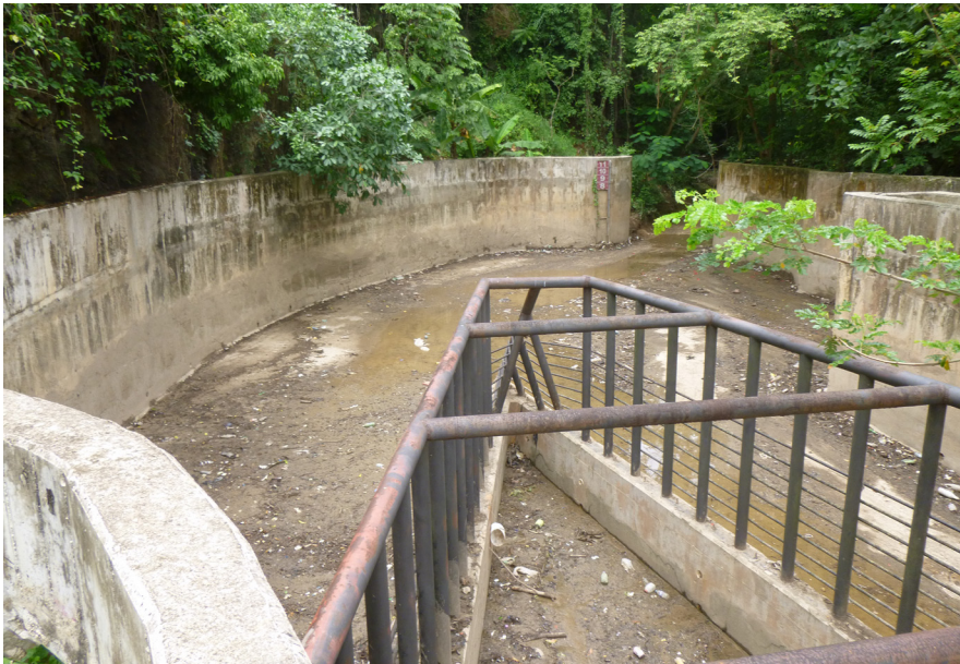
A section of the South Gully Silt Trap in St. James which was recently cleaned under the NWA's Mitigation Programme.
