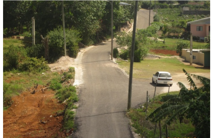
V-drain Works Completed on the Mt. Prospect Road, Manchester
