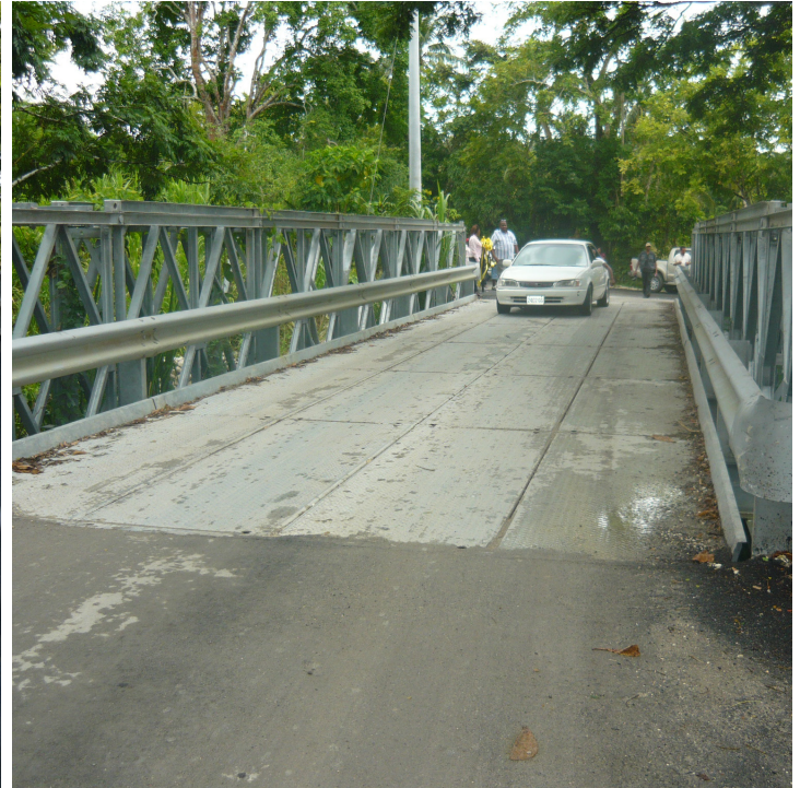
Fontabelle Bridge, St. Mary
