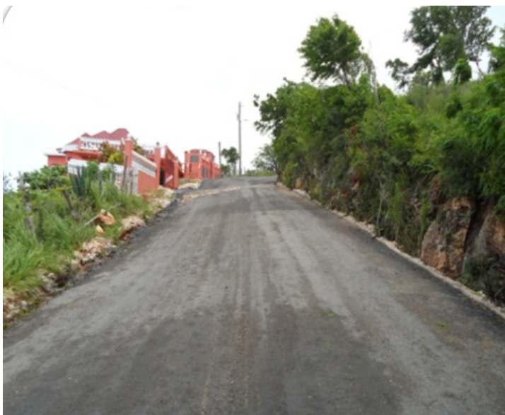
A section of road prepared for surfacing
