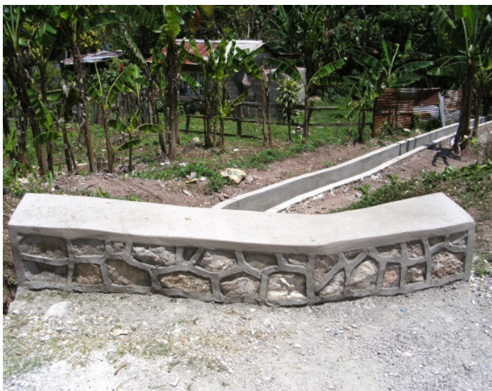
Crooked River "U" Drain and Parapet Wall
