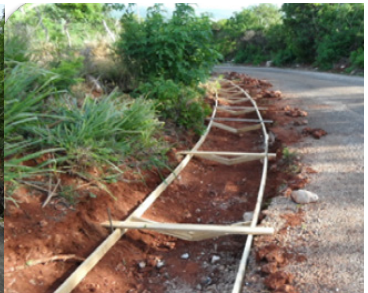
V Drain construction along the Round Hill road
