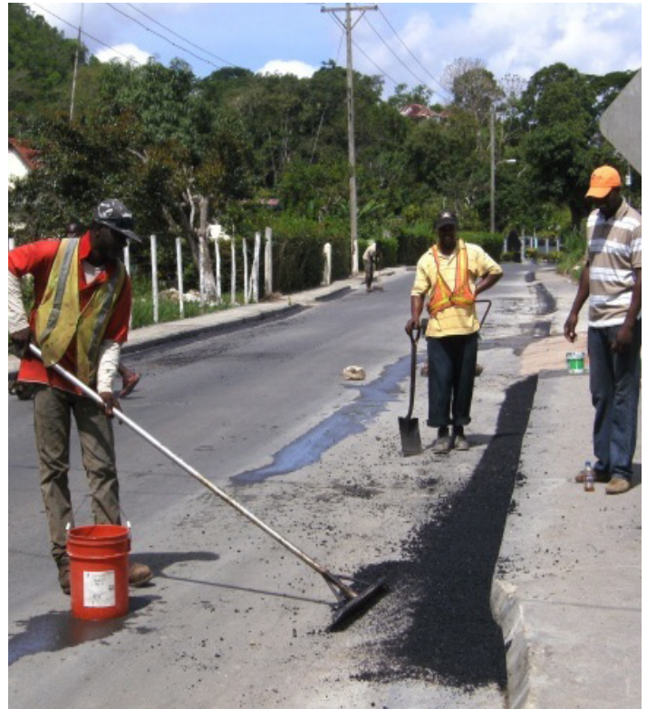
Aenon Town Sidewalk and Patching
