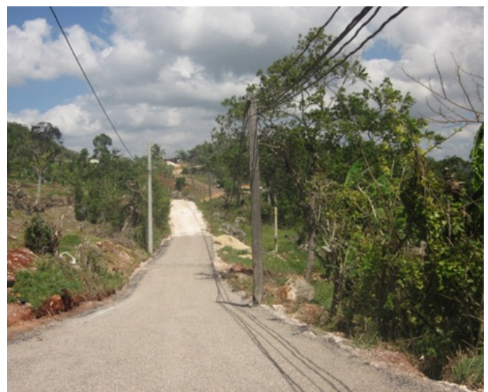
Big Heads Road Rehabilitation, Manchester
