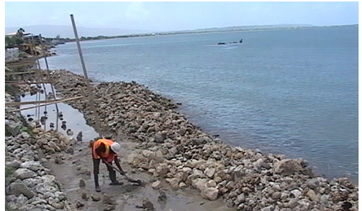
Construction of foundation of the seawall on High Street
