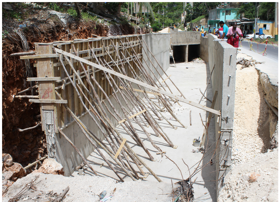
A section of the drain
