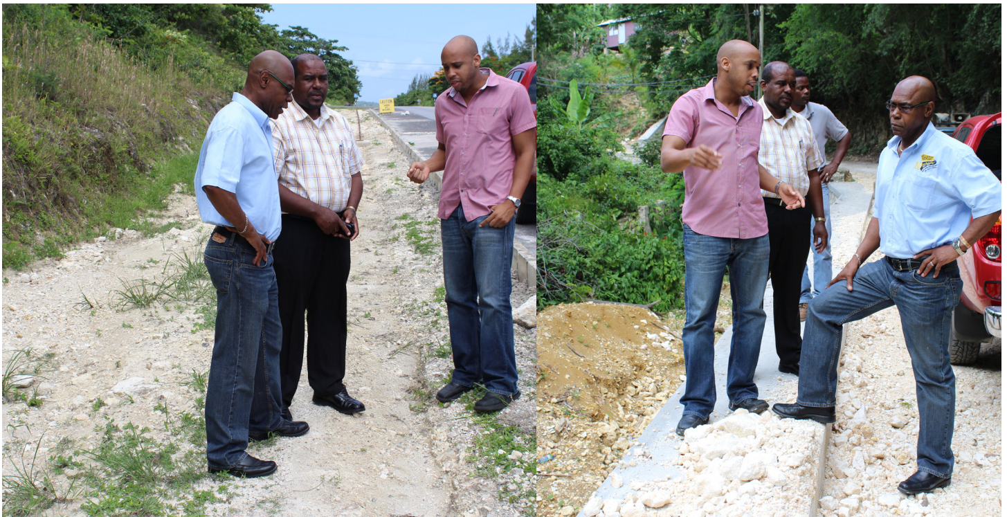
E. G. Hunter on tour of projects in Hanover, including the construction of sidewalks near Hopewell High School and the rehabilitation of the Sandy Bay to Montpelier Corridor.
