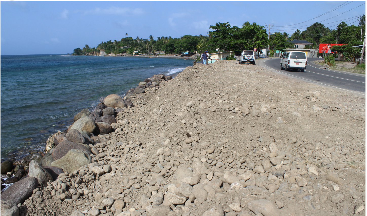
Sea Defence works being undertaken at Orange Bay, Portland
