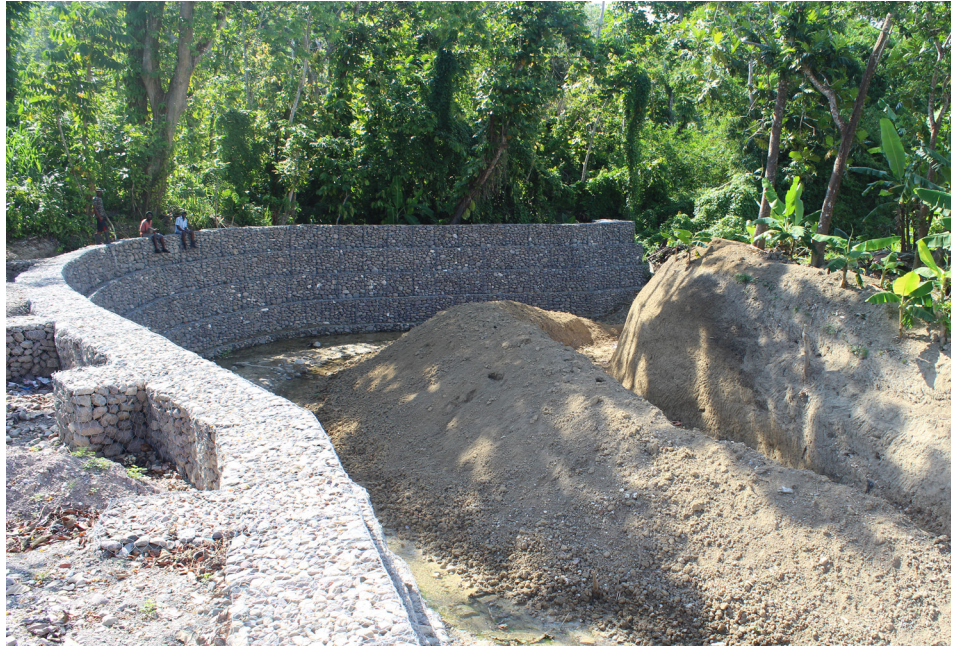
Gabion Wall at Otrum River, St. Mary
