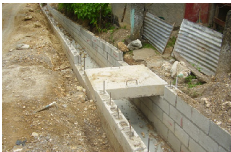
A concrete slab, allowing access to a private property, placed across the concrete U-drain that is being constructed along the Spring Head to Days Mountain roadway in St. Mary
