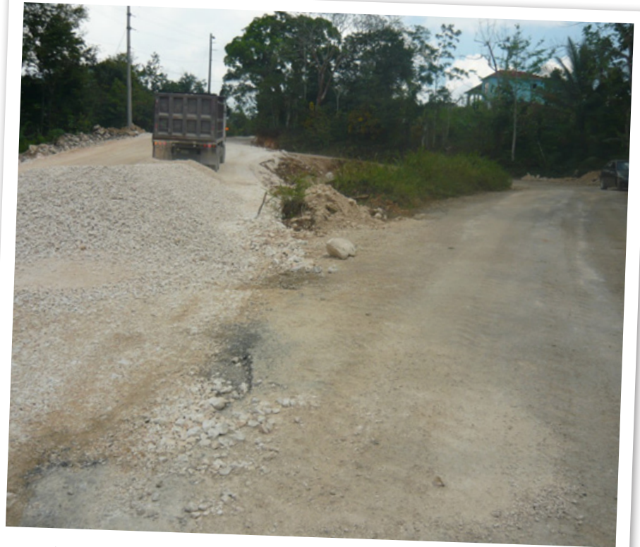
Truck depositing material in preparation for paving of the Sligoville roadway
