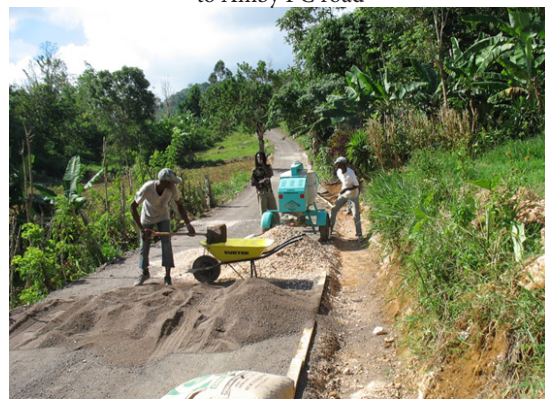
Construction of V-drains on the Far Enough PC Road
