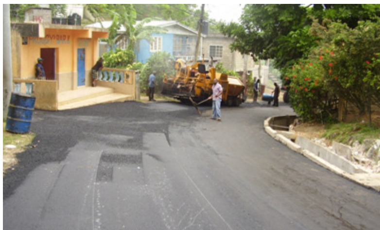
Roadway being resurfaced with Asphaltic Concrete along the Spring Head to Days Mountain control section in St. Mary
