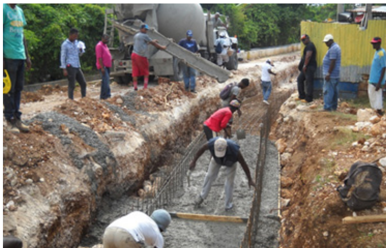
Concrete being poured to construct the invert of an underground drain along the Oracabessa to Days Mountain (Canoe Pond and Airy Hill) roadway, St. Mary
