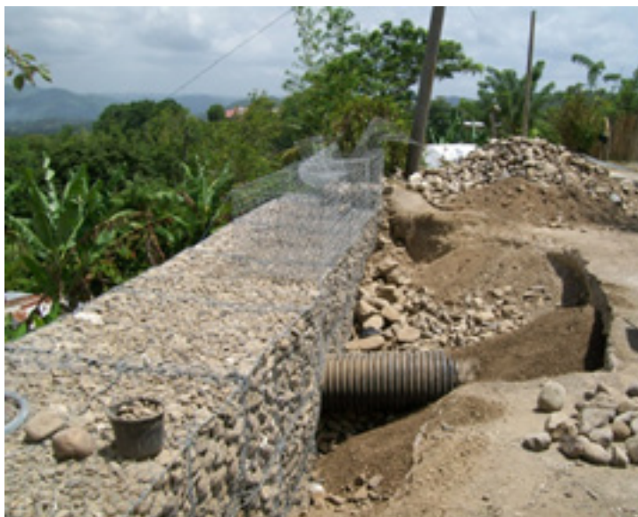
Gabion Retaining Wall being constructed at Pear Tree Grove in St. Mary
