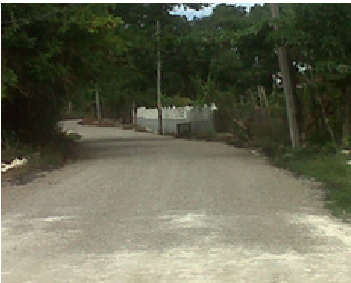
Hamstead roadway in St. Ann newly rehabilitated with Double Surface Dressing
