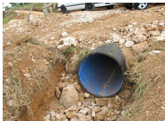
Construction of culvert on the Silver Grove to Amby PC road
