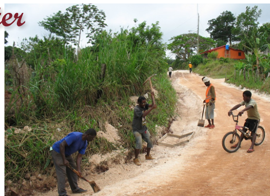
Construction of V-drains on the Medsfield to Barry Hill PC Road
