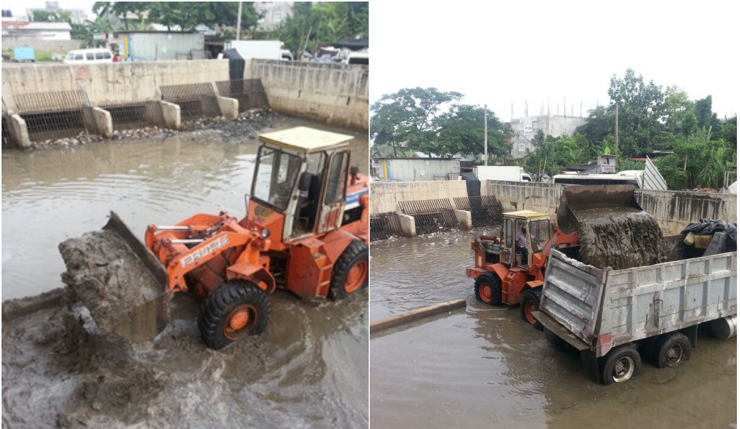
Cleaning of a section of the South Gully (Dome Street Silt Trap) in St. James
