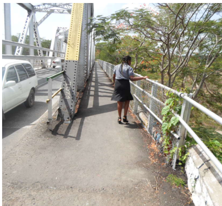
A pedestrian making her way across the May Pen Bridge along the newly refurbished walkway. The two walkways were fixed and new rails put up to improve the safety of persons.
