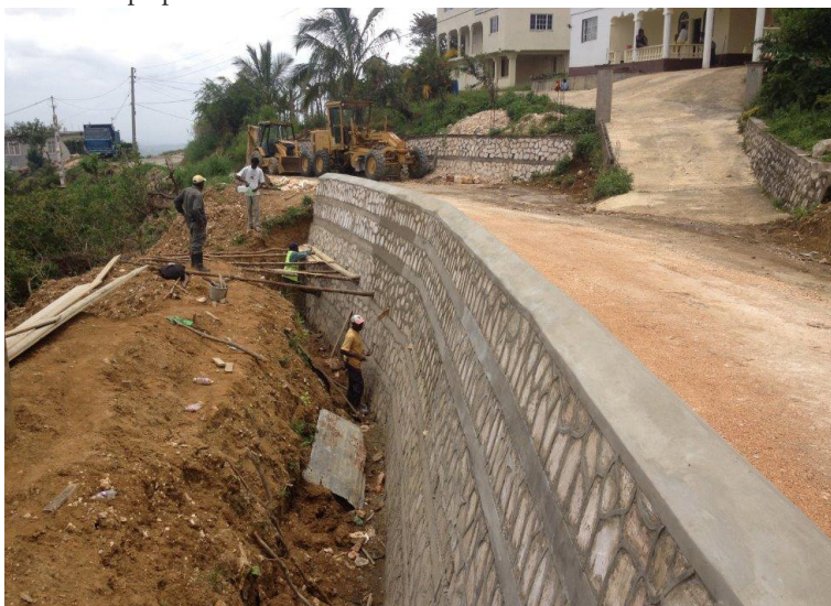
A section of the Top Litchfield roadway in Trelawny, where a retaining wall was constructed under the JEEP.
