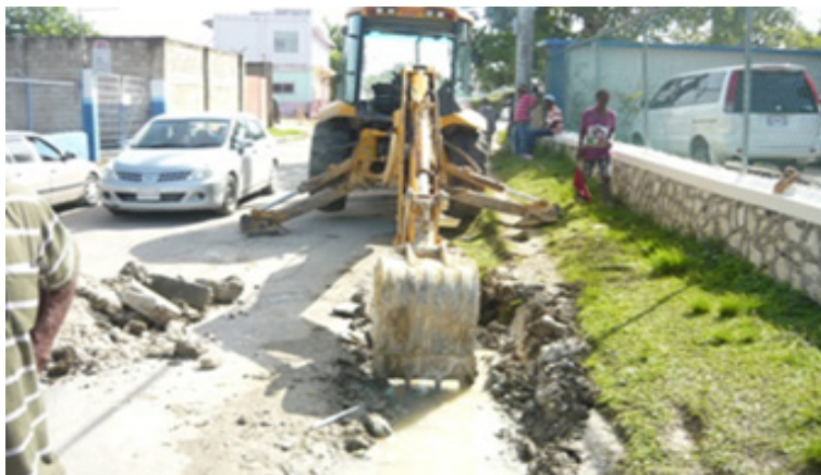
Rose Street , Savanna la Mar Westmoreland – The area is being excavated in preparation for the reconstruction of a concrete U drain
