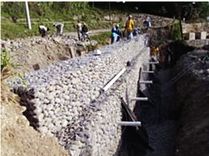
Gabion wall being constructed at West Hill, along the Breastworks to Windsor roadway in Portland
