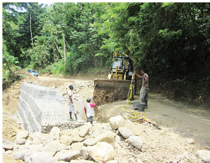
Gabion retaining wall being constructed along the Fort George to Camberwell control section
