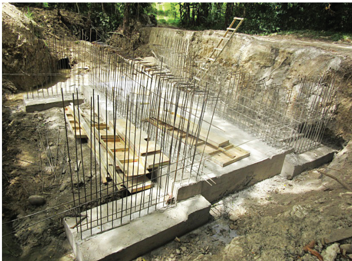
Concrete casting of the foundation of the Box Culvert completed, along Palmetto Grove to Pear Tree Grove roadway
