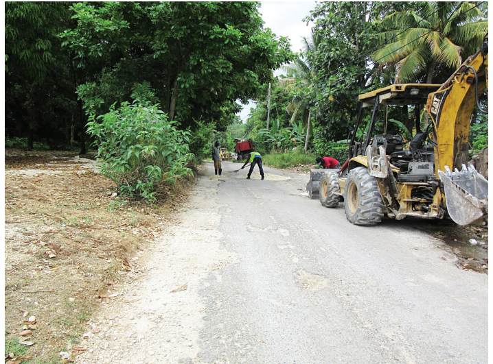
Preparation of road way for patching
