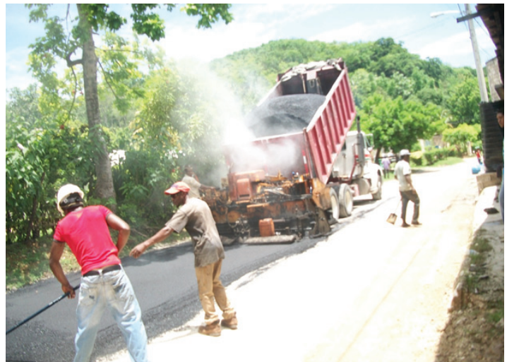
Hot mix patching in progress
