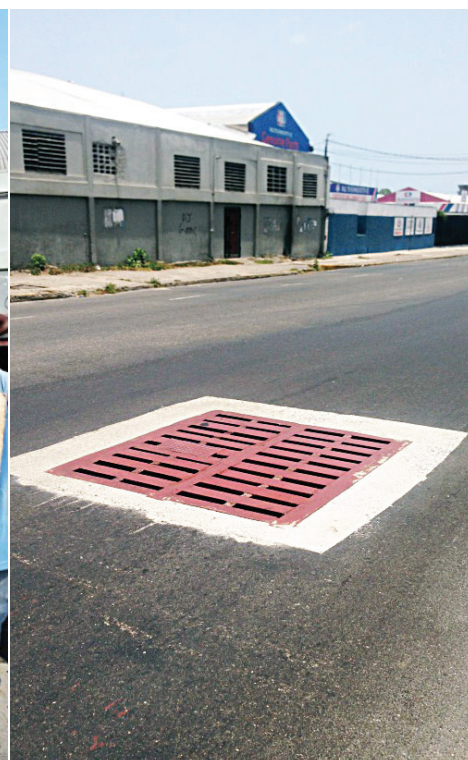
Installation of new Grating along Hagley Park Road
