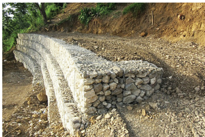
Toe wall at Frontier Heights, after being backfilled
