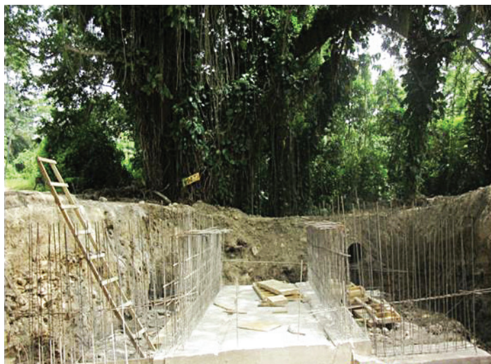
Concrete casting of the foundation of the Box Culvert completed, along Palmetto Grove to Pear Tree Grove roadway
