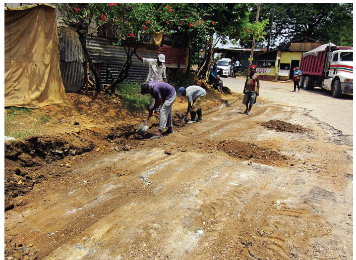
Clearing of a blocked drain
