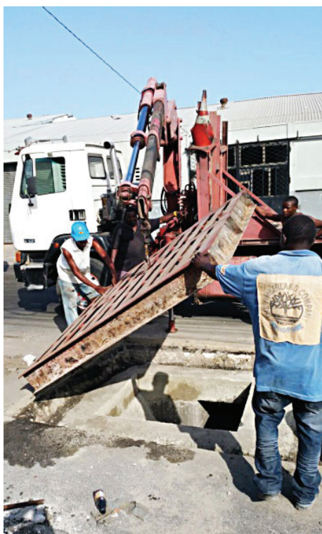
Installation of new Grating along Hagley Park Road
