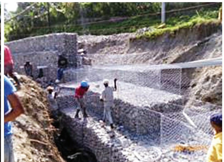
Gabion wall being constructed at West Hill, along the Breastworks to Windsor roadway in Portland
