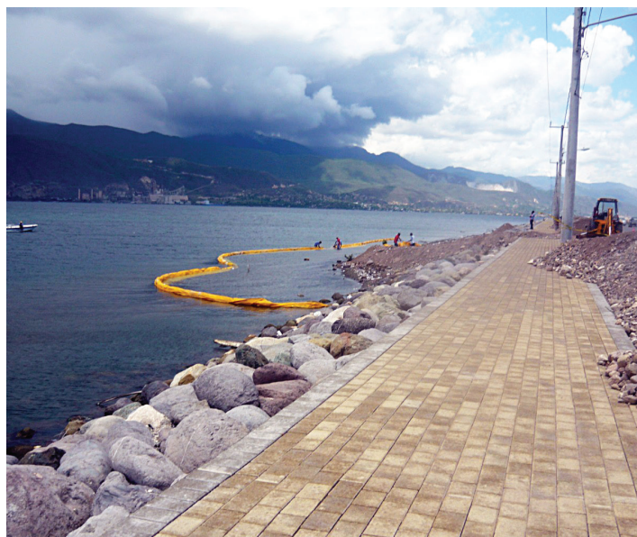
Turbidity barriers are being put in place. These barriers act as silt traps and also control contaminants brought into the area. These barriers also control wave action and protect newly placed material from erosion.
