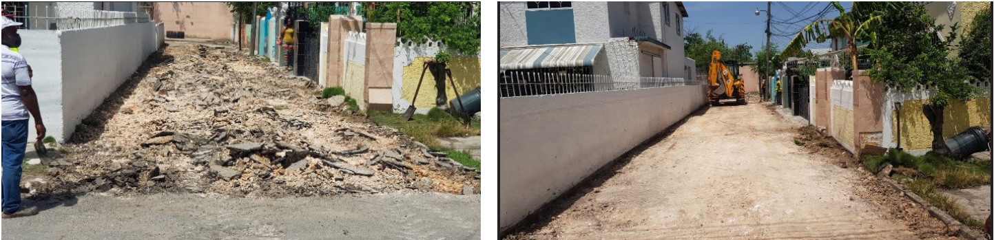
Milling and base works being undertaken at Bob Marley Way in Cooreville Gardens
