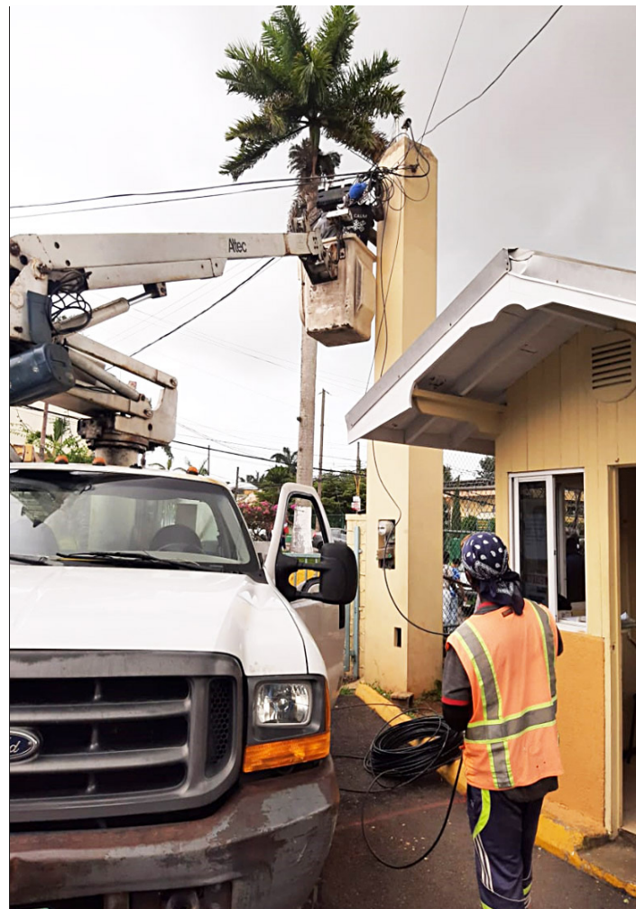
Fibre Optic Cables being laid at the Manchester Municipal Corporation the fiber network.
