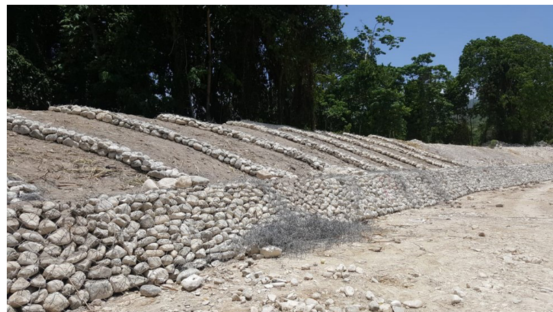
River Training works that were undertaken in the Woodstock housing scheme in Buff Bay, Portland
