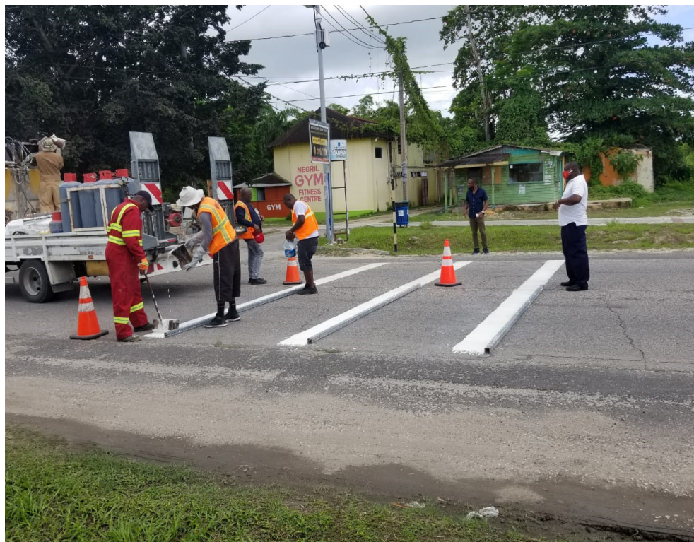
An NWA team installs Rumble Strips along a section of the Norman Manley Boulevard.
