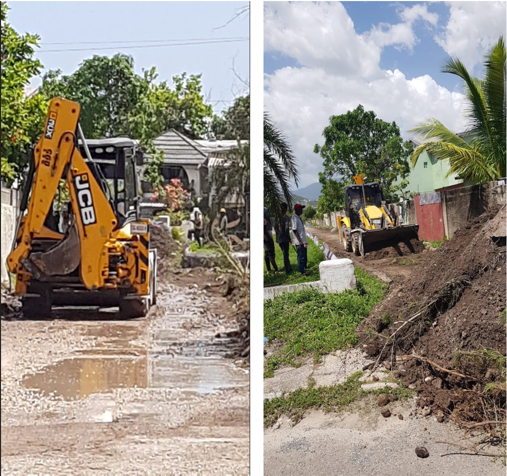
A backhoe clearing a section of roadway in Cooreville Gardens in preparation for surface reconstruction
