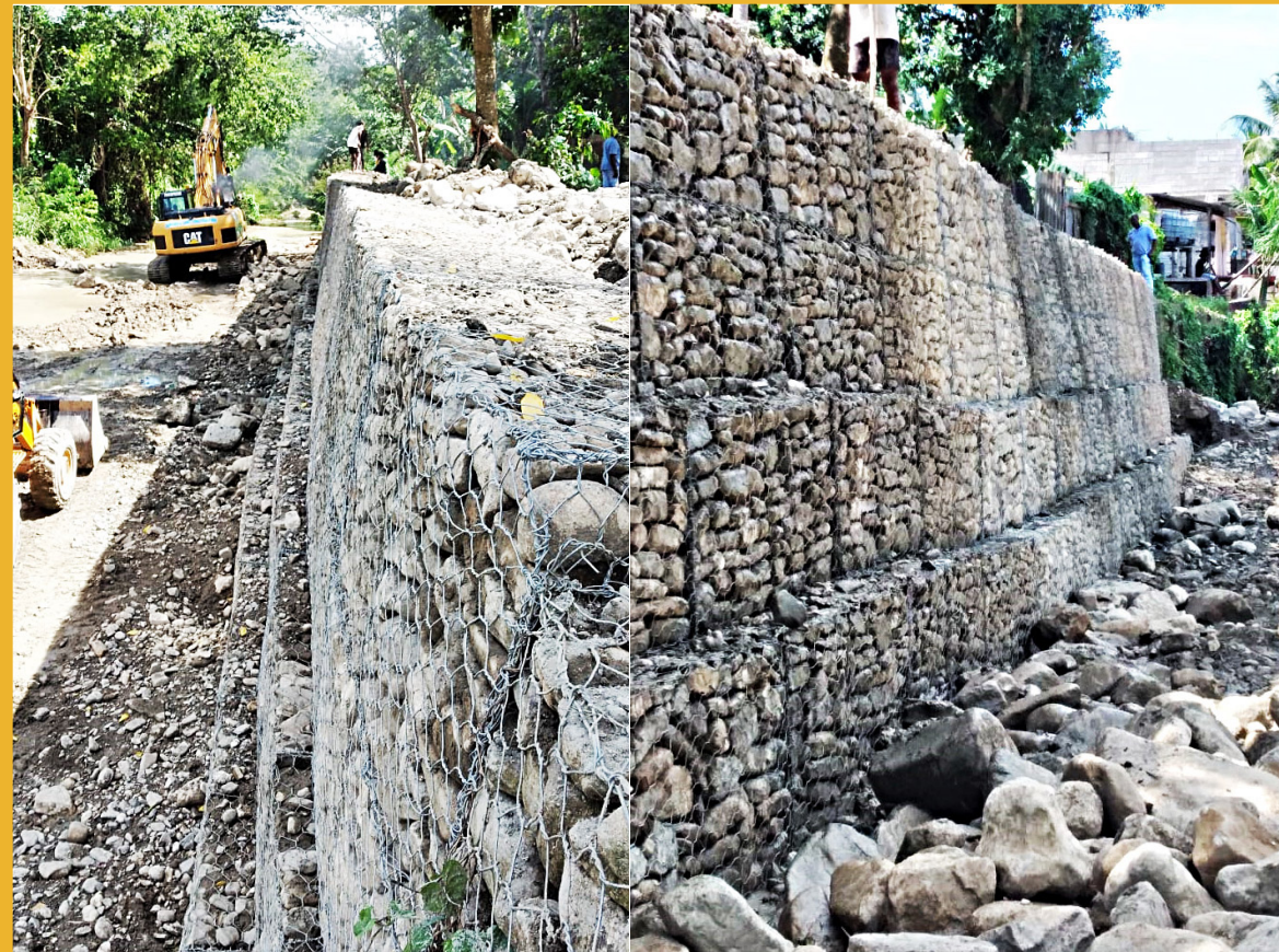
Completed River Training Works at Orange River, St. Mary. The works were undertaken through a contract valued at $3.1 -Million. It saw the construction of some 37 metres of Gabion protective wall reinforced with geotextile fabric as part of the works to protect the community from Orange River, especially when in spate.
