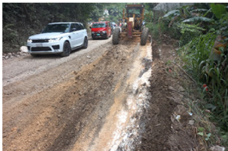
Surface preparation for subsequent paving
