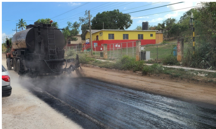
Applying Prime coat in preparation for paving
