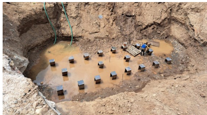
Capping of piles in north abutment
