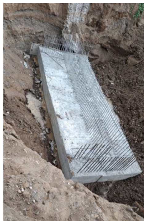
Completed foundation for north
