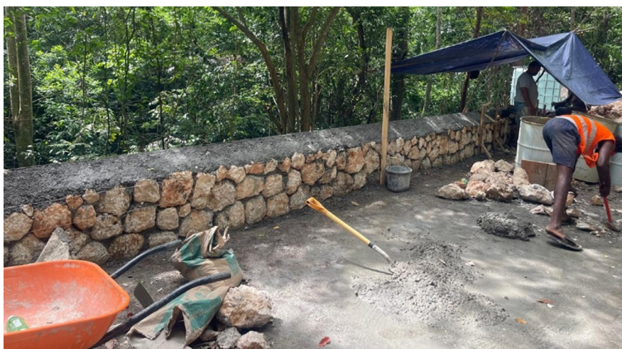
Parapet section of a retaining wall along with coping underway.
