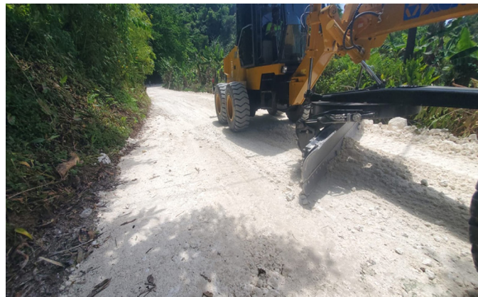
Motor Grader being used to spread approved base material at Bellevue Road
