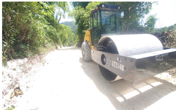
Compaction works underway along the Bellevue Road in Portland
