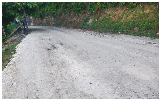
Base works in progress along Black Hill to Rodney Hall roadway
