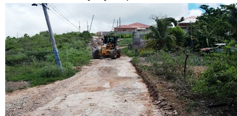
Grading along the Tryall PC Road
