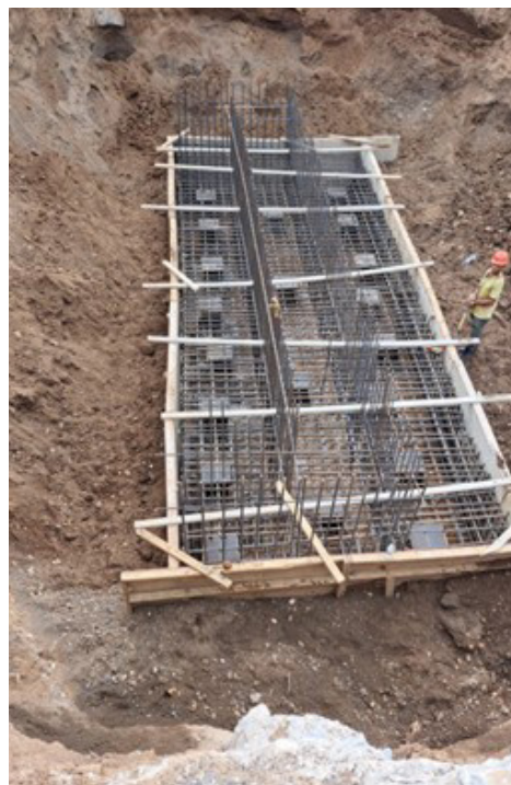
Reinforcement bars and formwork in place for pouring of abutment foundation
