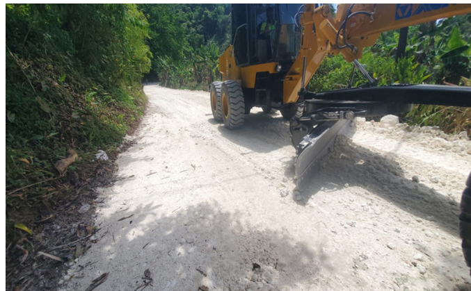
Motor Grader being used to spread approved base material at Bellevue Road
