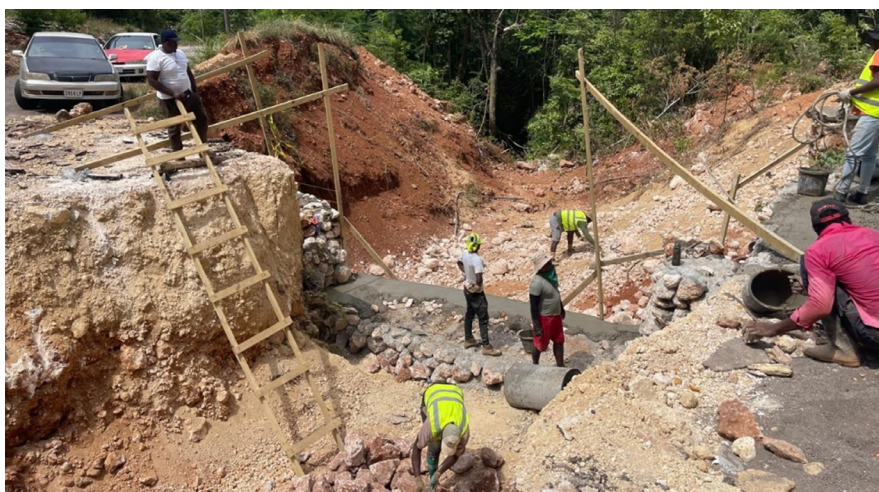
An excavated section of the road in preparation for the relaying of culverts.
