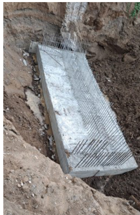
Completed foundation for north
