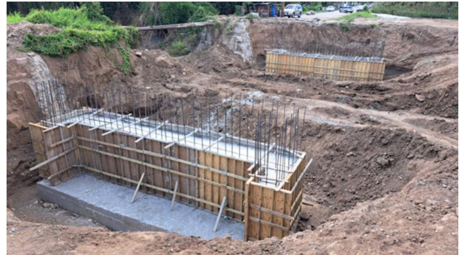
North and south abutments of Spring Village Bridge following concrete pour in early June 2025
