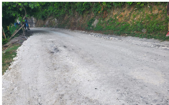
Base works in progress along Black Hill to Rodney Hall roadway
