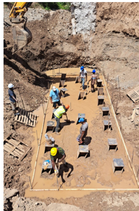
Preparations for blinding concrete on north and south abutments
