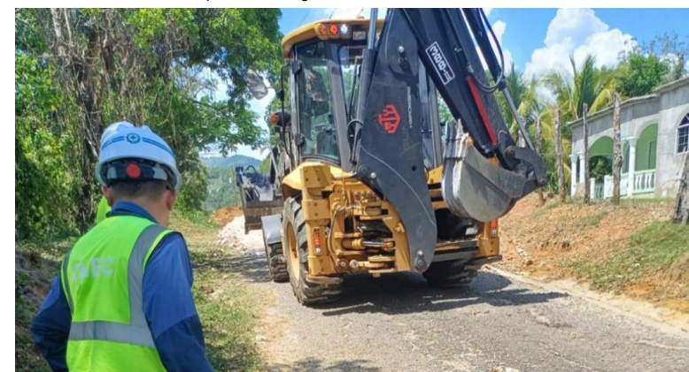
Preparatory work along the Holland Village road
