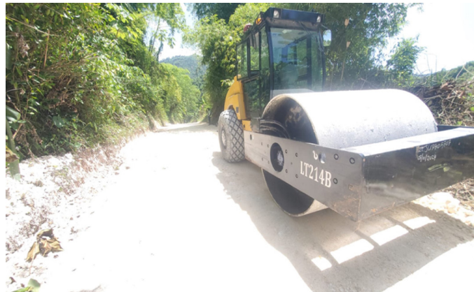
Compaction works underway along the Bellevue Road in Portland
