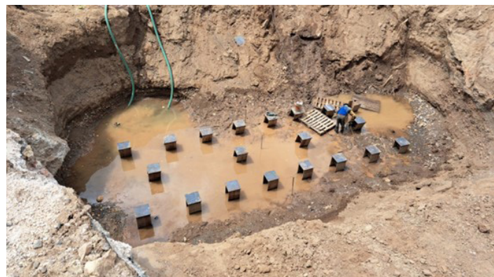
Capping of piles in north abutment
