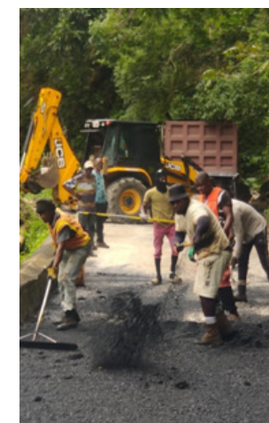
From Left: Lutemen helping to spread the asphalt onto the surface of the roadway; Roller being used to compact the material. Paved roadway.
