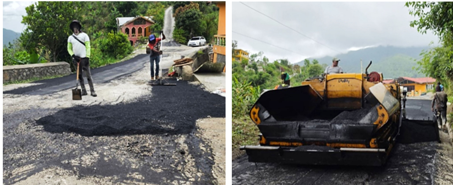
At left: Luteman and shovel men preparing the Section to Hardwar Gap roadway for paving. At right: Paver on site of Section to Hardwar Gap in Portland.
