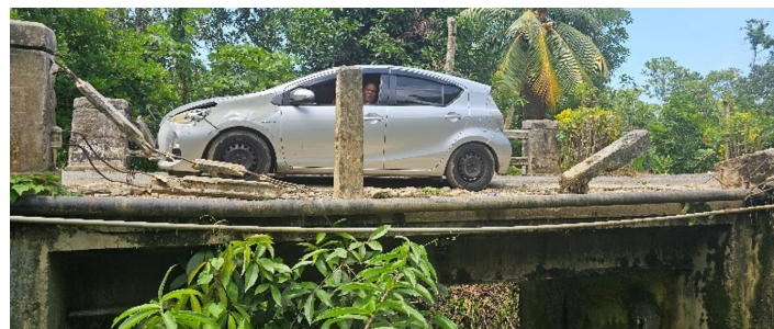
The Askenish Bridge in Hanover.
