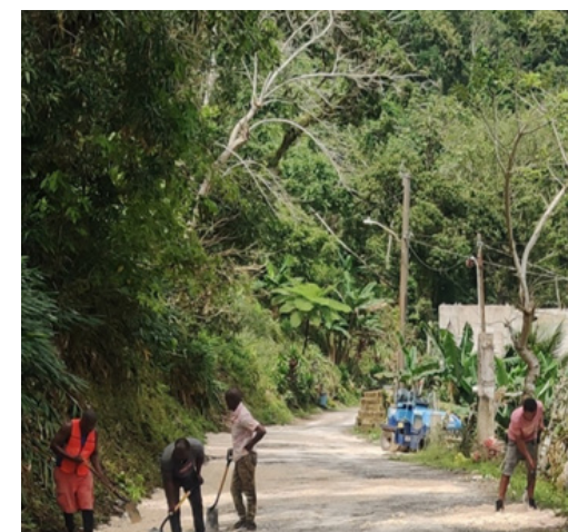
Preparatory works being done along the Wakefield to Red Shop roadway in Portland.
