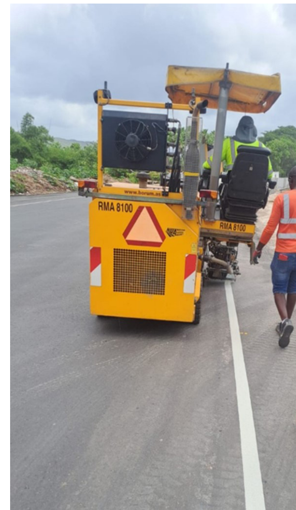
Team applying thermoplastic layer to the surface prior to the bridge's official opening
