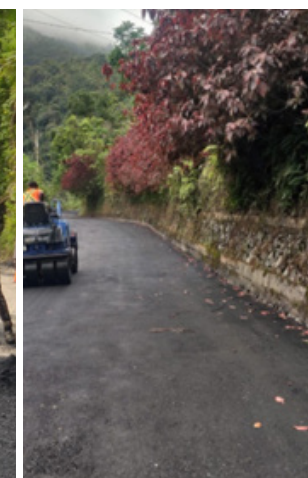
From Left: Lutemen helping to spread the asphalt onto the surface of the roadway; Roller being used to compact the material. Paved roadway.
