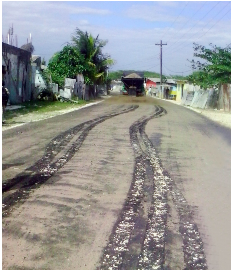
Road being sanded after oiling as part of the construction process.
