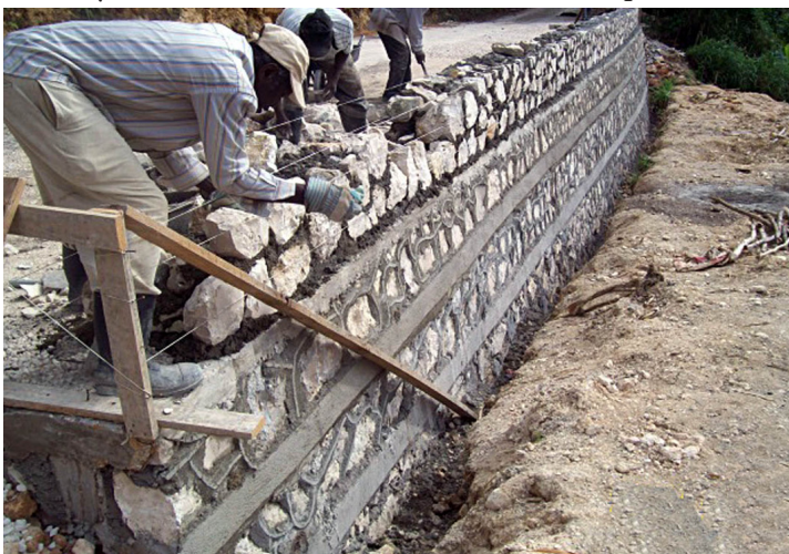
Random Rubble Retaining Wall along the Free Hill roadway during and after construction
