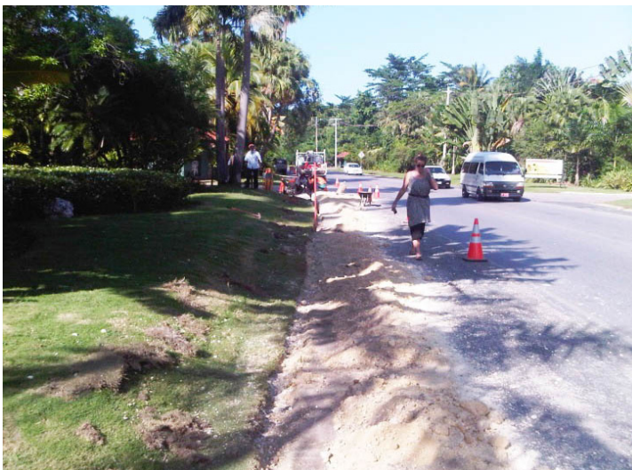
Negril, Westmoreland, Jamaica (tourist destination): Trench being cut for the installation of Fibre Optic Cable.
