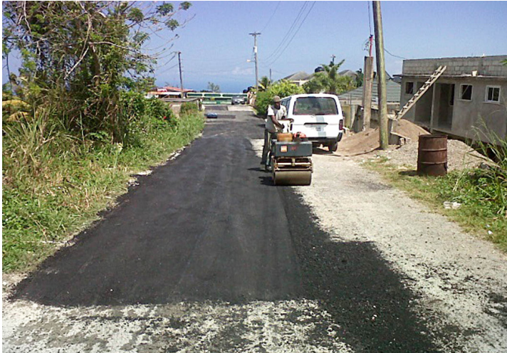
Sheet patching underway along the Free Hill main road in St. Ann
