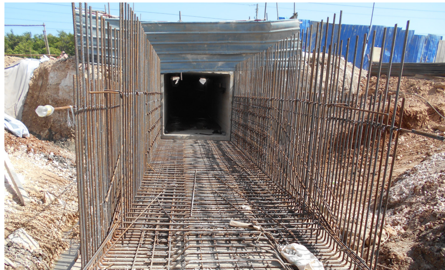
Construction of a Box Culvert which is among new drainage features along the corridor.
