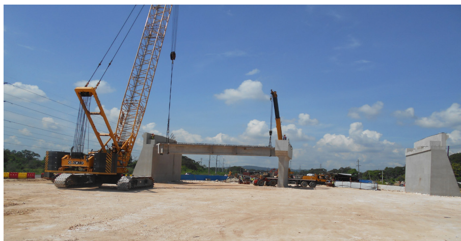
Concrete Girders being positioned as part of the construction of the Overpass Bridge that facilitates travel to and from the Mandela Service road.
