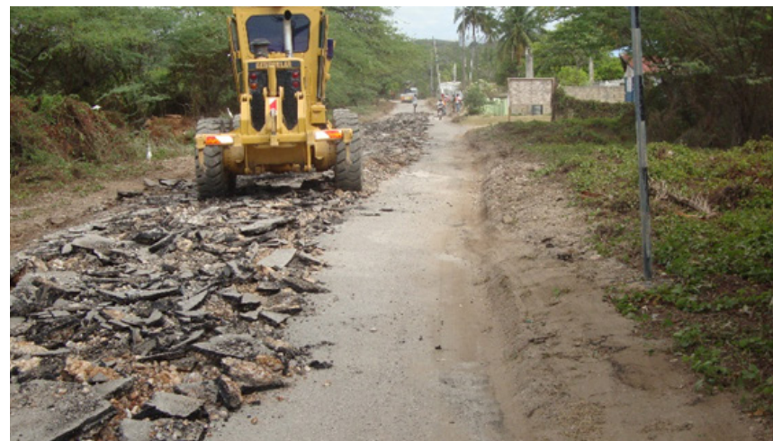
Scarification Works being undertaken
