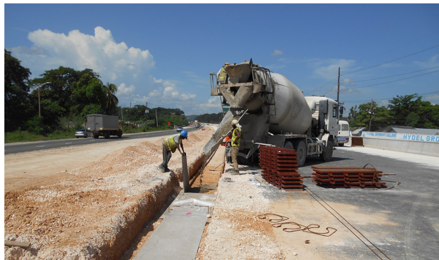
Concrete being poured for the construction of a section of the Retaining Walls along the corridor.
