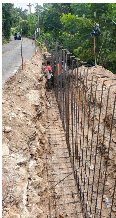
At left: Steelwork being done for reinforced concrete retaining wall; Right: formwork being removed from reinforced concrete retaining wall
