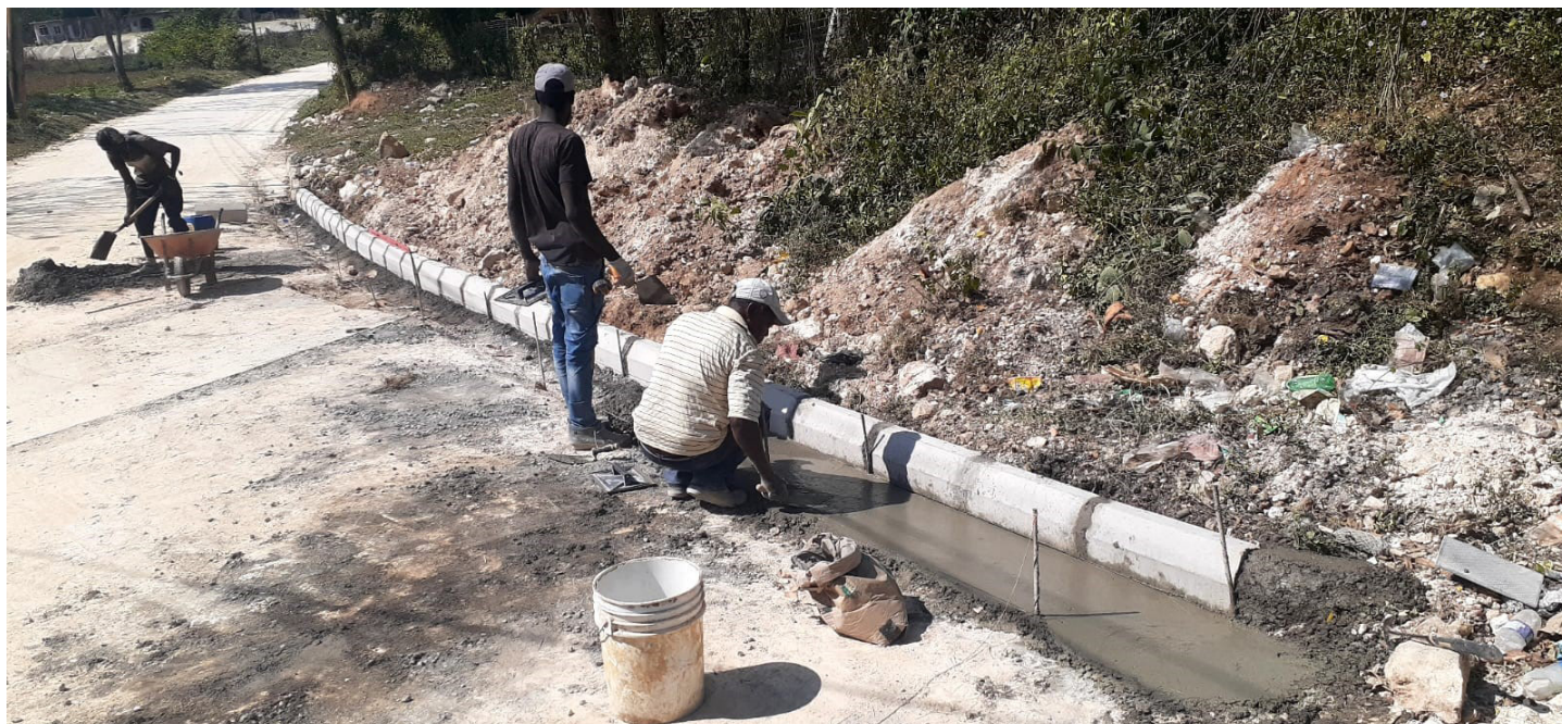
Installation of kerb and channel drains along a section of the Clarks Town to Hyde roadway in Trelawny.
