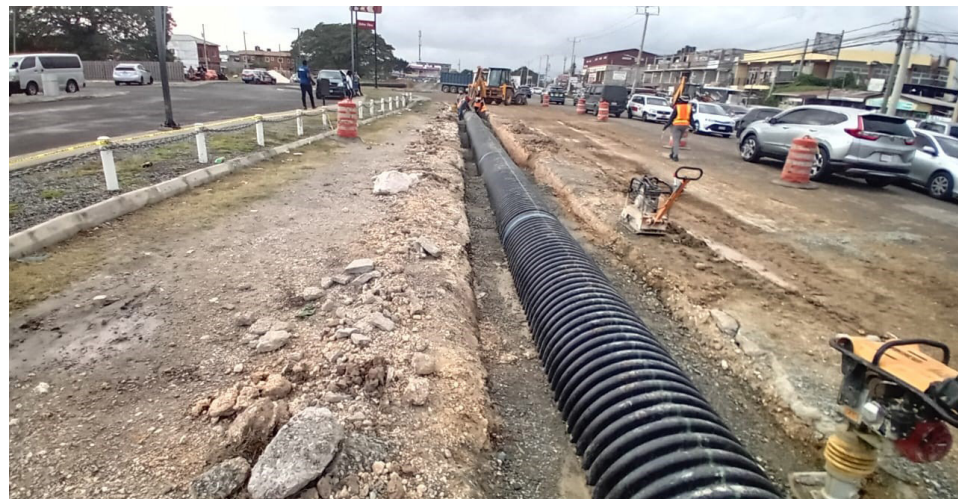
Installation of pipe culvert
