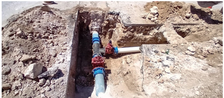
Connection of pipelines
