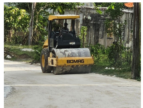
Base formation works along a section of the Little Spring to River Road corridor in Bluefields, Westmoreland.
