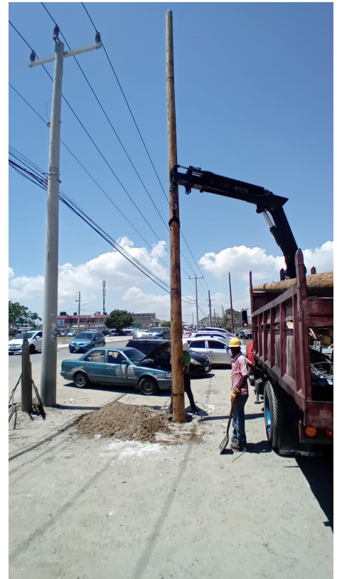
At left: installation of waterpipeline; At right: relocation of utility pole
