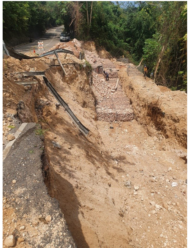
Construction of gabion retaining wall on Runaway Bay to Browns Town rehabilitation project
