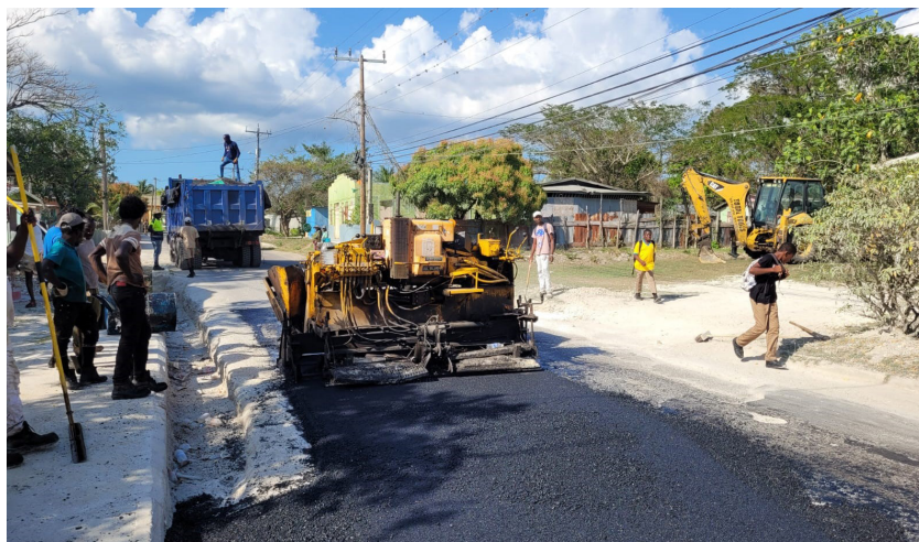
Paving works along a section of the Grange Hill to Little London roadway
