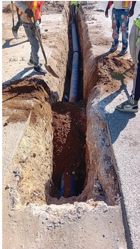
At left: installation of waterpipeline; At right: relocation of utility pole
