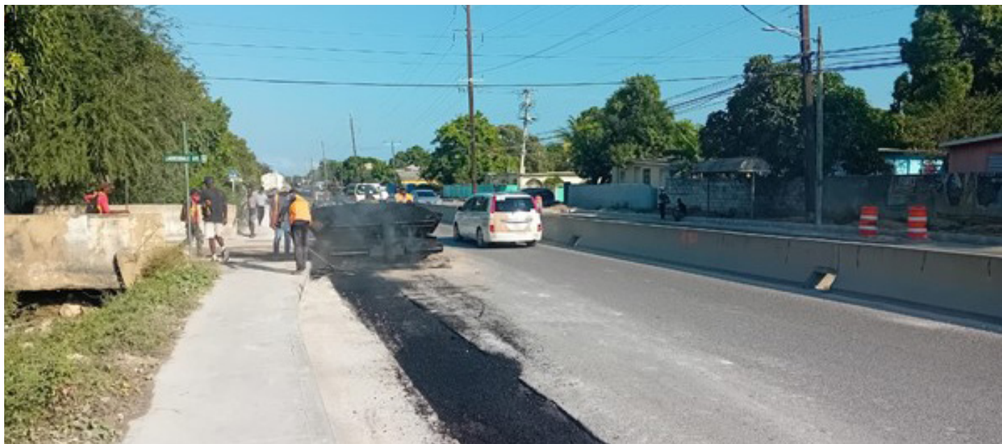
Reinstatement of pipeline trench
