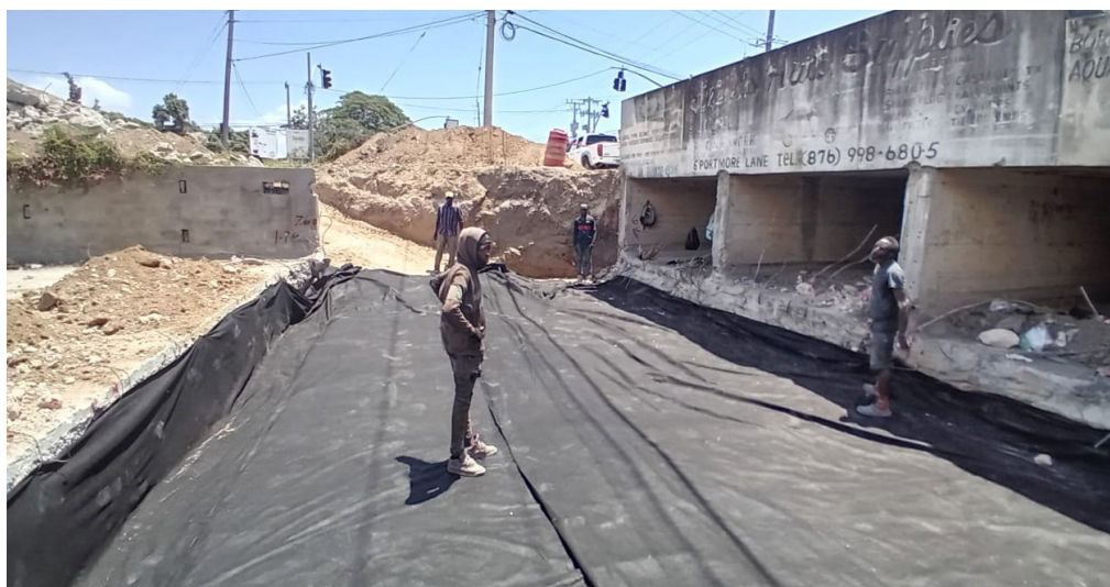
Placement of waterproofing membrane to prevent water from getting under the foundation of the box culvert
