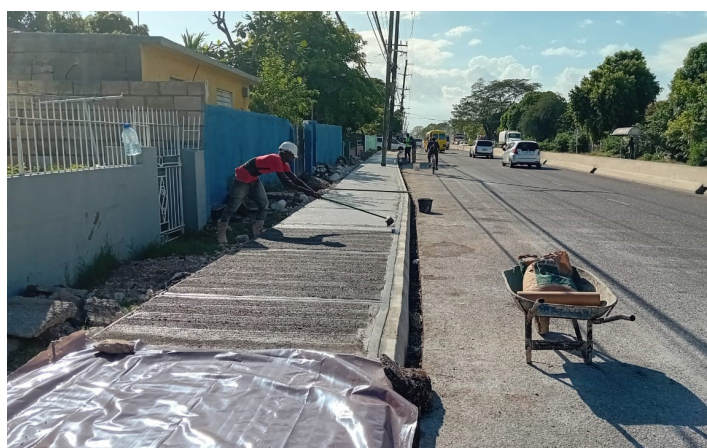
Construction of concrete sidewalks
