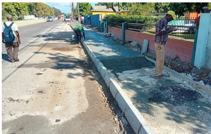
Construction of concrete sidewalks
