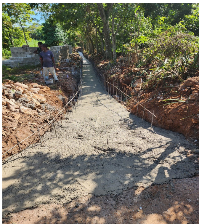
Cement Works as part of drain construction
