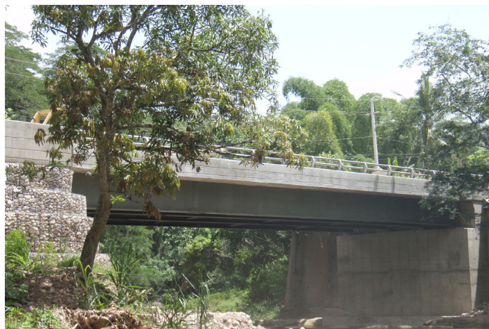
Angels River Bridge Clarendon
