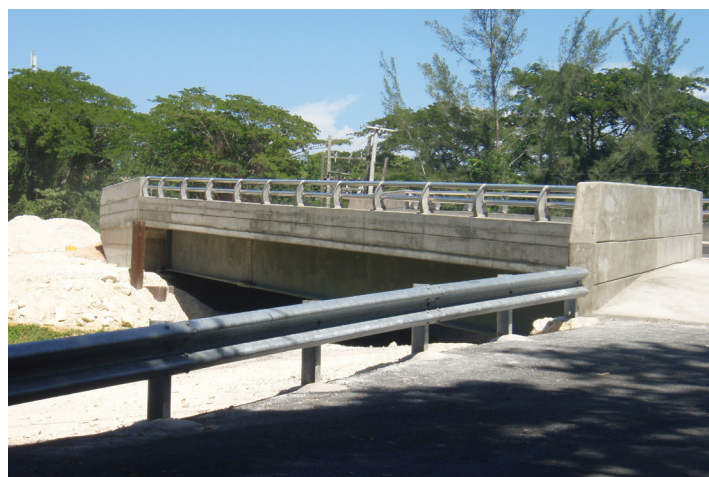
Martha Brae Bridge Trelawny
