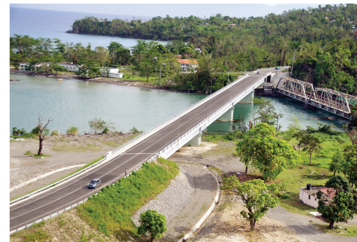
Rio Grande Bridge, Portland
