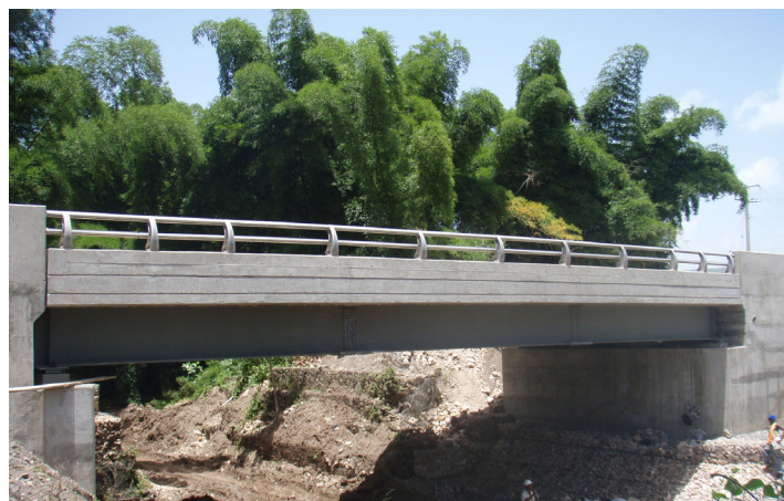
Worthy Park Bridge, St. Catherine
