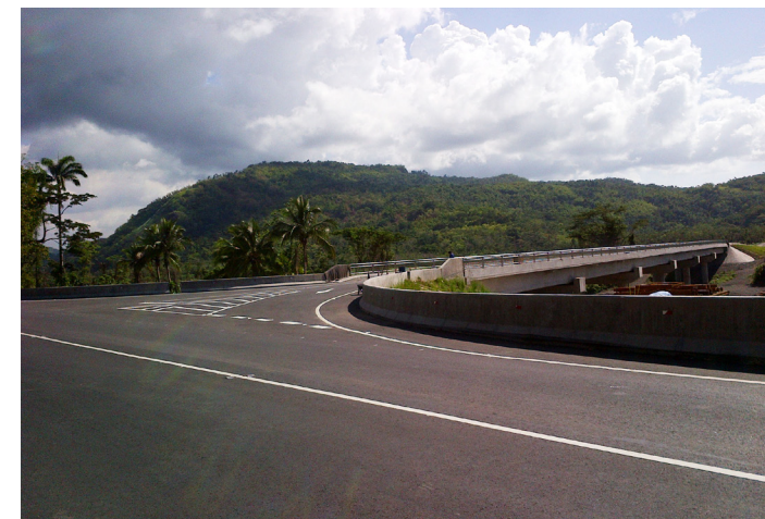
Westmoreland Bridge, St. Mary
