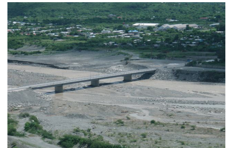
Yallahs Bridge, St. Thomas
