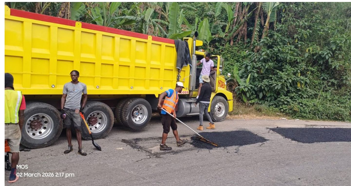
Patching works along a section of the North Coast Highway in Trelawny in the vicinity of the Greenside community.
