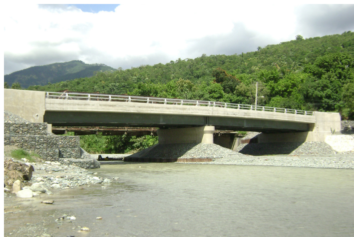
Johnson River Bridge, St. Thomas
