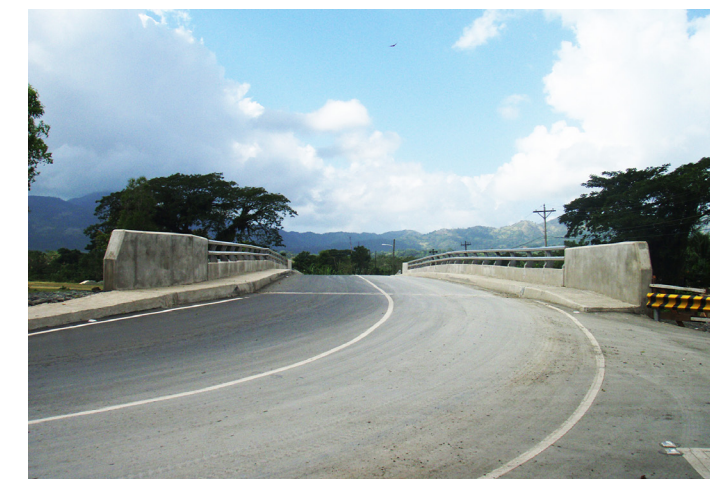
Black River Bridge, Portland
