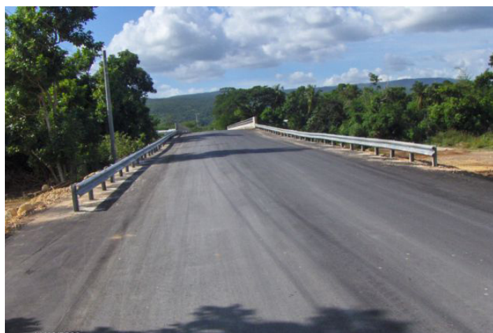
Milk River Bridge, Clarendon
