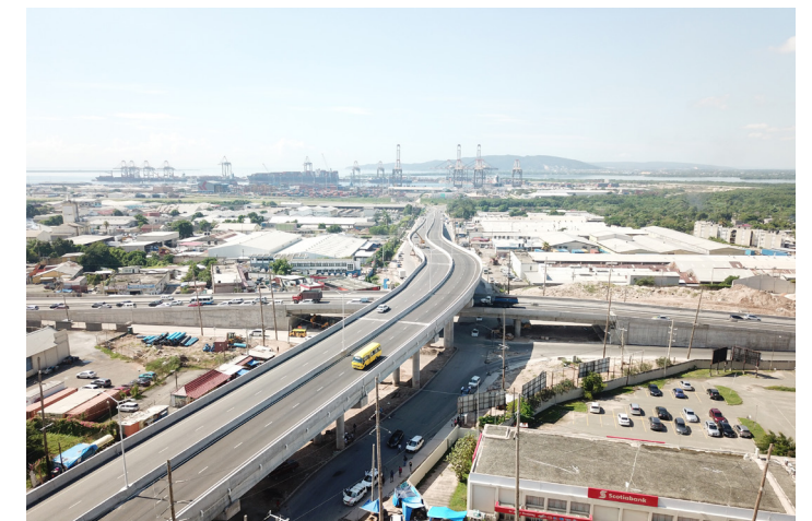
Overpass Structure, Three Miles, St. Andrew
