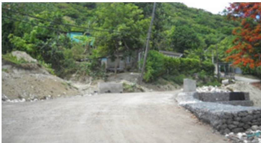
The completed box culvert and gabion retaining wall at Grants Town in St. Mary
