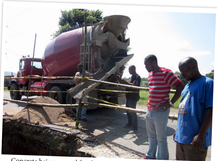
Concrete being poured for the Retaining wall foundation at Knollis, St. Catherine
