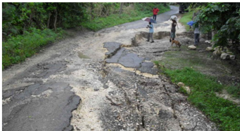
The Villa Road in St. Mary as at January 22, 2014, after being badly damaged by flood rains
