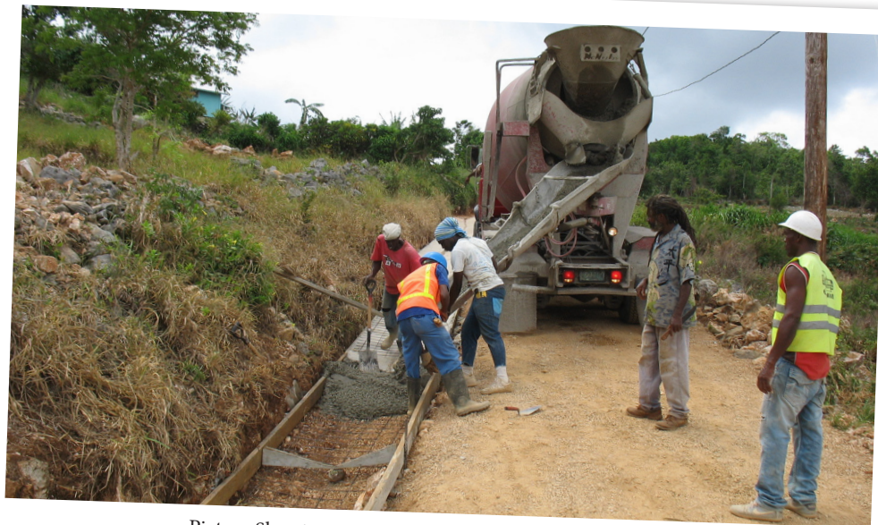
Picture Showing Pouring of Concrete to Construct V-Drain
