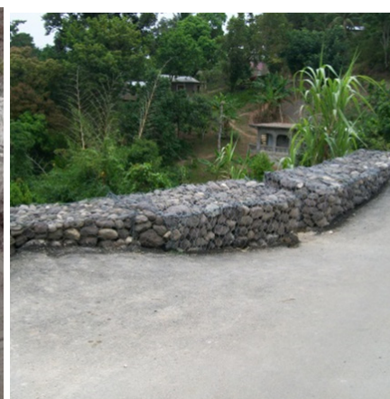
North Eastern Region St. Mary - Gibbs Hill, South East; Completed Gabion Wall
