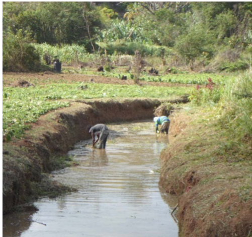
Southern Region Clarendon- Carthy Hill (Desire Road); Cleaning of Earth Drain
