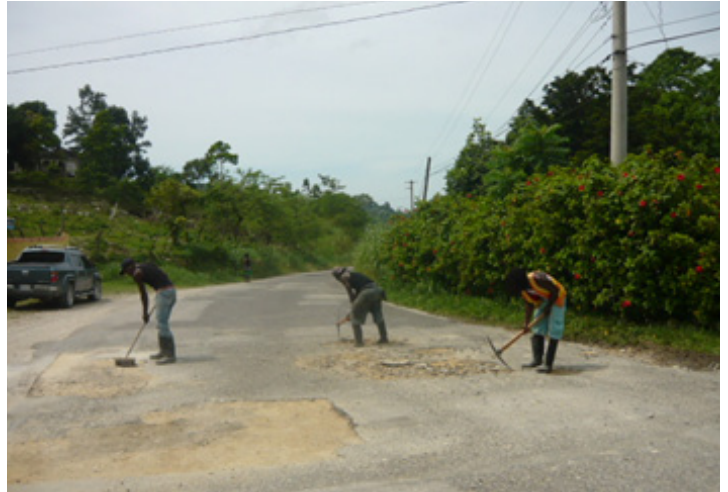
Workmen preparing sections of the Ferris Cross to Mackfield roadway for the application of Asphaltic Concrete
