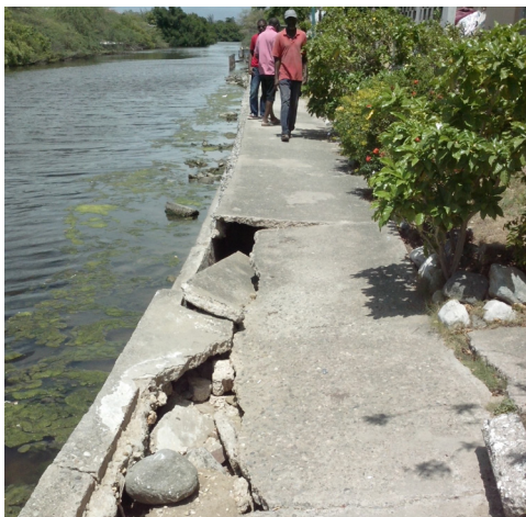
South East Region St. Catherine - Armarda Courts; Removal of collapsed pavement and reconstruction
