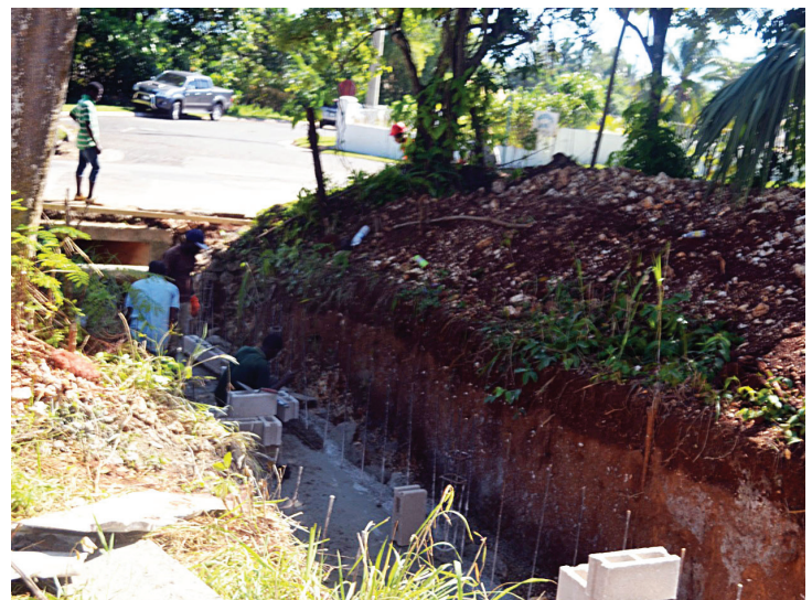
Concrete U-drain being built along the Leeds to Santa Cruz Road
