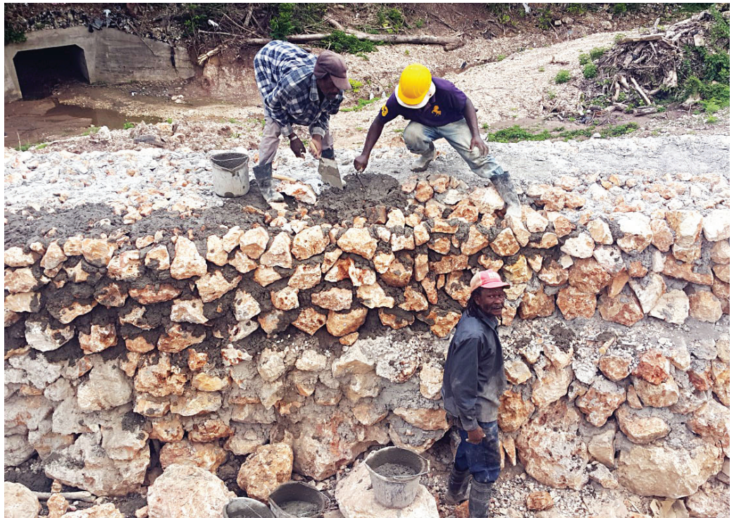
Workmen busy erecting a section of the wall, which will be backfilled to allow for the safe passage by motorists who use this busy road.
