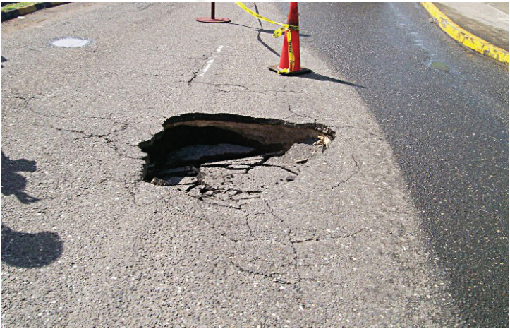
Failed section of roadway, as detected by passing motorists
