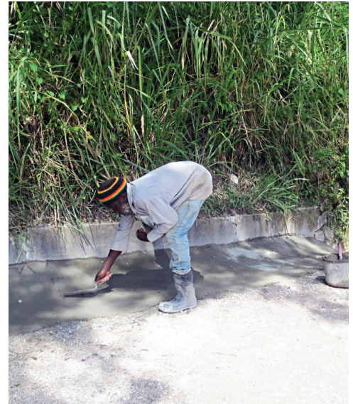
Pell River – Workmen construct a drain along the Pell River roadway
