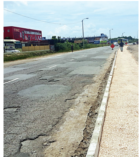
A section of the new sidewalk being constructed as part of the rehabilitative works.
