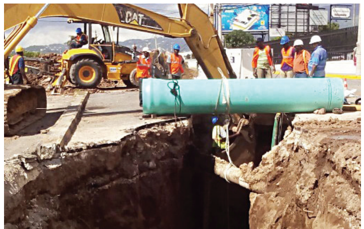
Sewer replacement pipe being placed in excavated roadway
