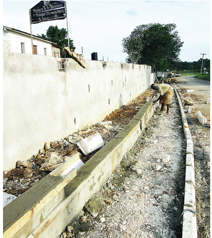
Work in progress at Bogue in St. Elizabeth - Flower Box and installation of kerbs
