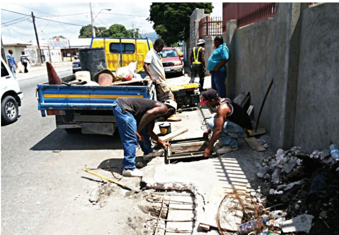
At left, workmen fixing a Manhole Cover along Lyndhurst Road. Right is the completed works.
