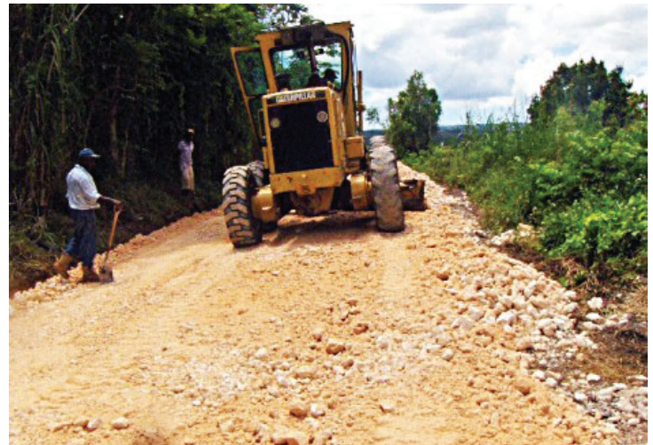
Marling of road in Broken Hurst
