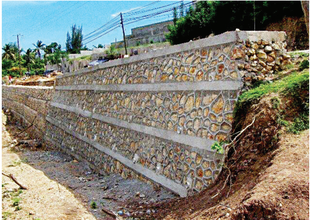
A partially completed section of the retaining wall
