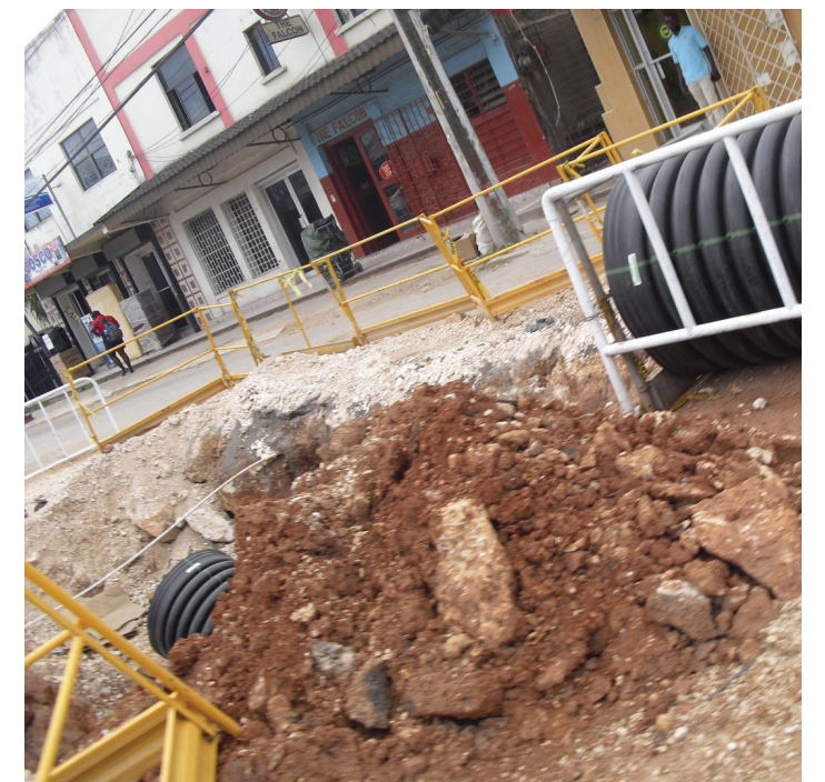
Work started to install 900mm pipe culvert along a section of Ward Avenue
