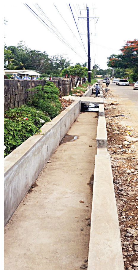
Construction of U-Drain nearing completion
