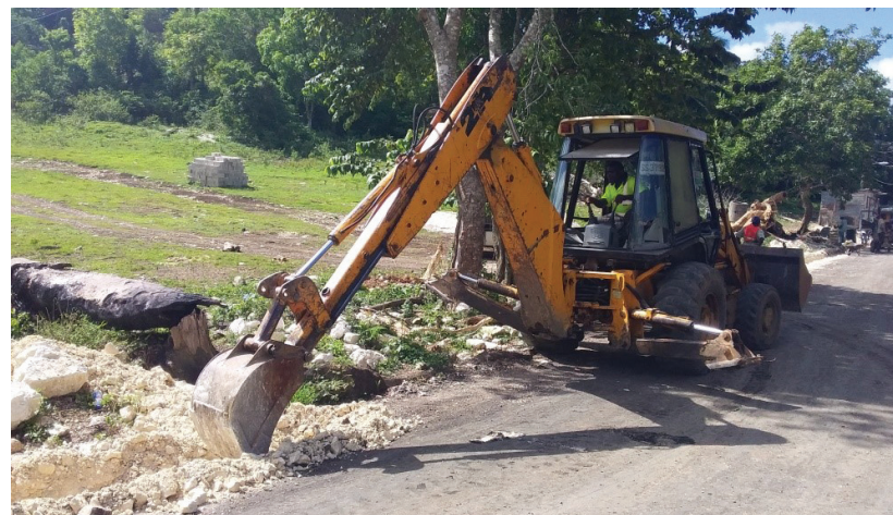
The excavation of a section of the roadway to facilitate the construction of drains
