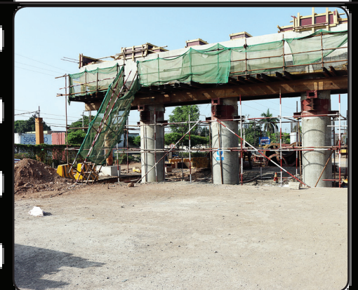
Pier and pier head construction complete.
