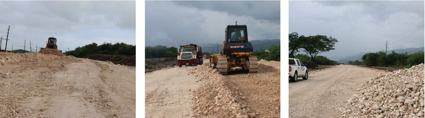
Sub-base works completed with base layer works in progress to form the two-lane 1.4km stretch of new road between Chesterfield and Marcus Garvey Drives. The project also involves the overlay of 700 metres of Chesterfield Drive, in the Seaview Community, which will have 1.5 metre-wide sidewalks on both sides. The approach to the Chesterfield Drive/Spanish Town Road intersection will also be widened to accommodate three lanes.
