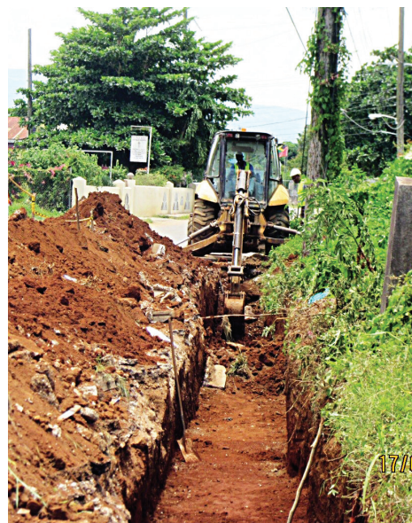
Excavation for 900 x 900mm U-Drain in progress
