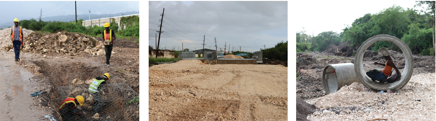
Labourers on the Chesterfield Drive ‘Bypass’ project filling gabion baskets with rocks as part of the protective works being undertaken in relation to a couple of waterways over which the road will pass (left). Two temporary Bailey bridges were installed closer to the Marcus Garvey Drive intersection to allow vehicular access over a major gully (centre) while a labourer shelters from the rain, which has hampered the pace of the project, in a concrete culvert (right).
