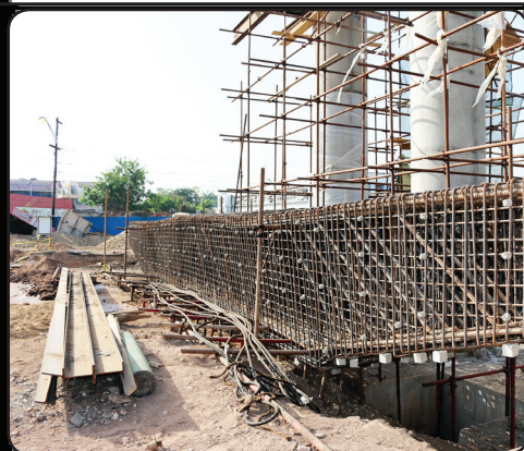
Prefabricated steel for the T-beam which is transported to the bridge construction site soon to be lifted atop the piers.
