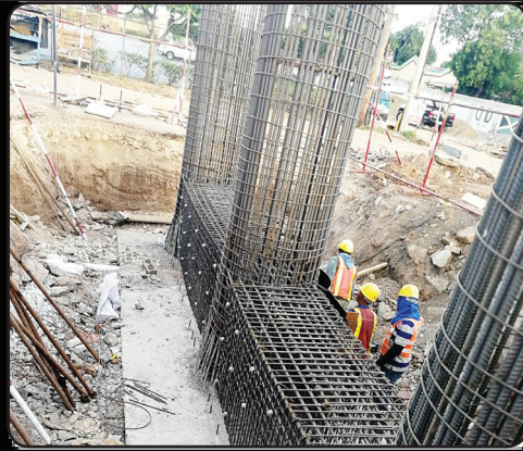
The ground work: intricate steel fabrication for the piers and pile caps that will anchor the piers below ground.
