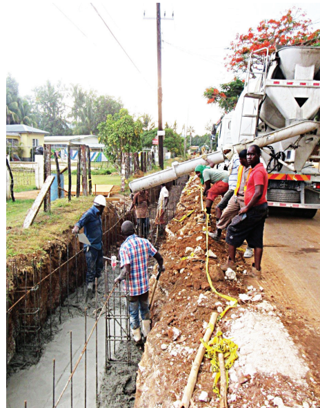
Concrete being poured for invert of 900 x 900mm U-Drain
