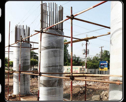
After being cast, reinforced concrete piers are wrapped in a special type of plastic material to complete the curing process
