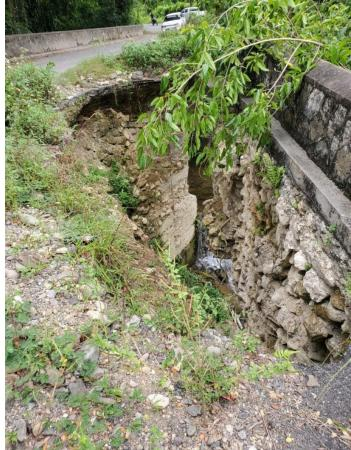
View of failure of roadway as a result of damage to retaining wall
