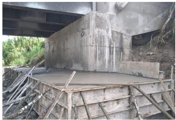
New beam seat and additional protective work to the southern abutment of the bridge
