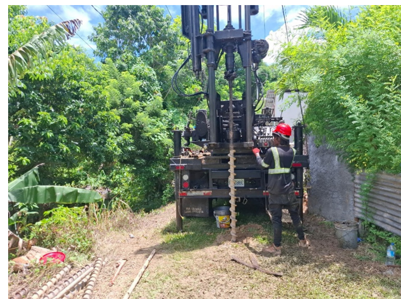
China Harbour Engineering Company Limited preparing their machine to conduct soil testing
