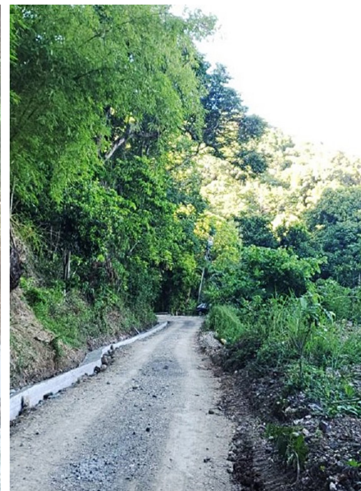
Camberwell Main Road: The Contractor erected formwork for the construction of kerb and gutter
