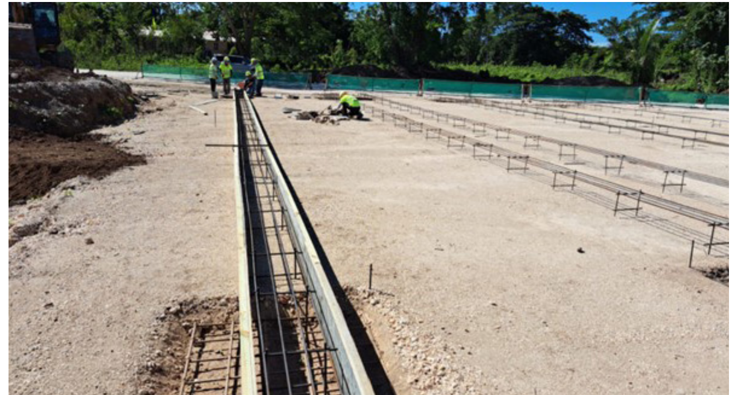
CHEC representatives toil on the installation of formwork for foundation beams
