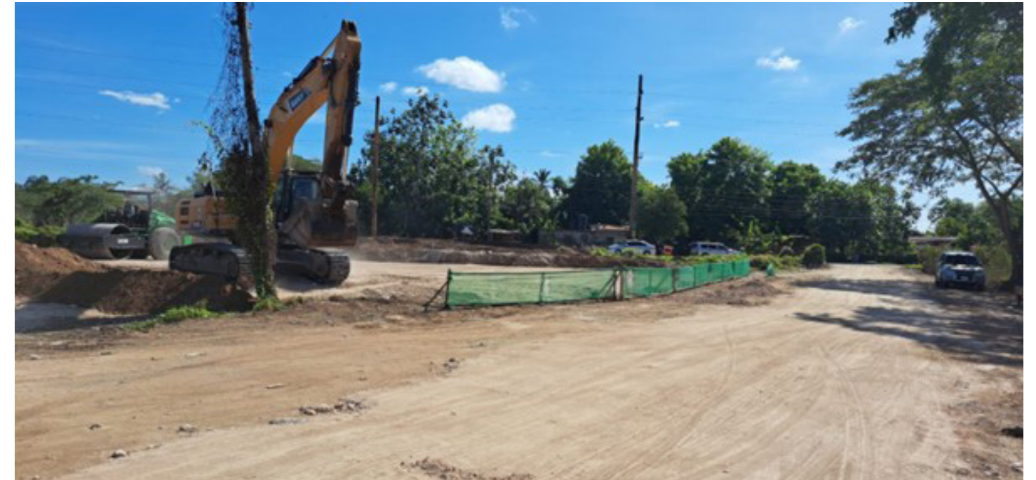
View of site yard to the left, properly delineated, and a then thinly marled detour road to facilitate traffic movements
