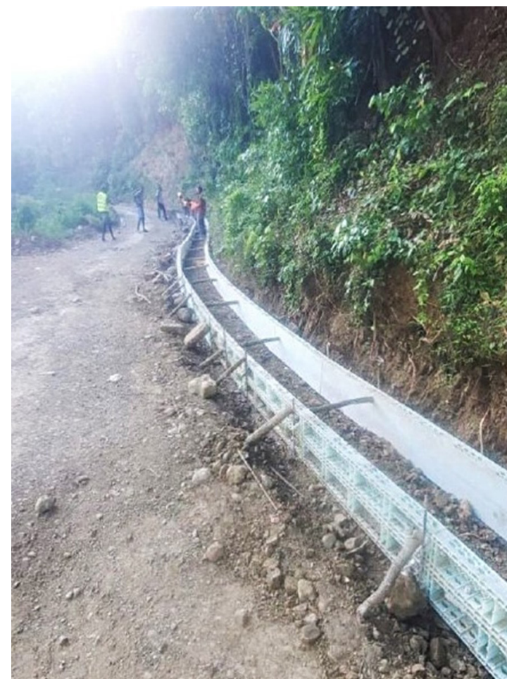
Camberwell Main Road: The Contractor erected formwork for the construction of kerb and gutter
