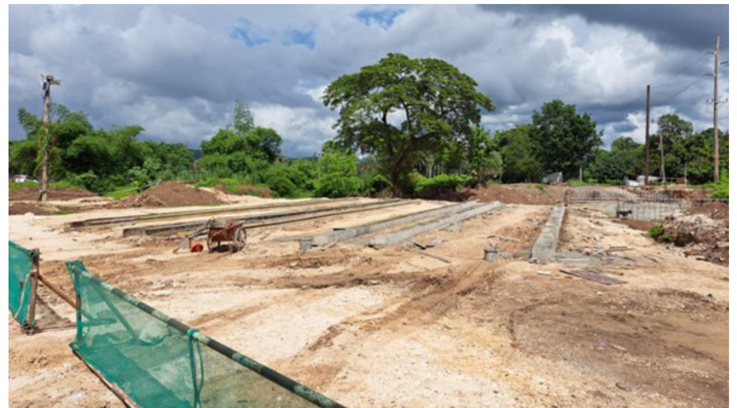
Three of the six bases, on which the girders will be constructed, are now complete.
