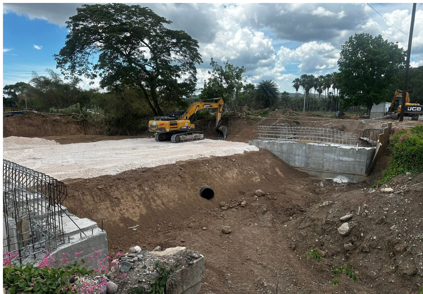
Construction of marl platform atop the earth base
