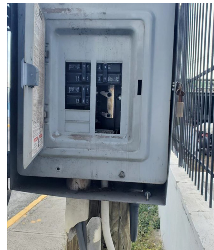
Vandalised and Tampered Panel Box along Dunrobin Avenue, St. Andrew
