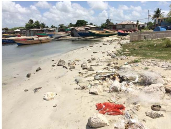
Figure 60: Rubbles on the beach indicating existence of groin in the past
